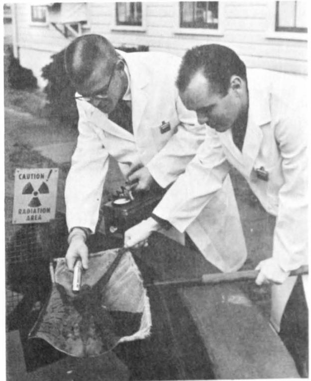
Scanning a skate for radioactivity after exposing it in water containing low levels of activity at Beaufort, N.C.
