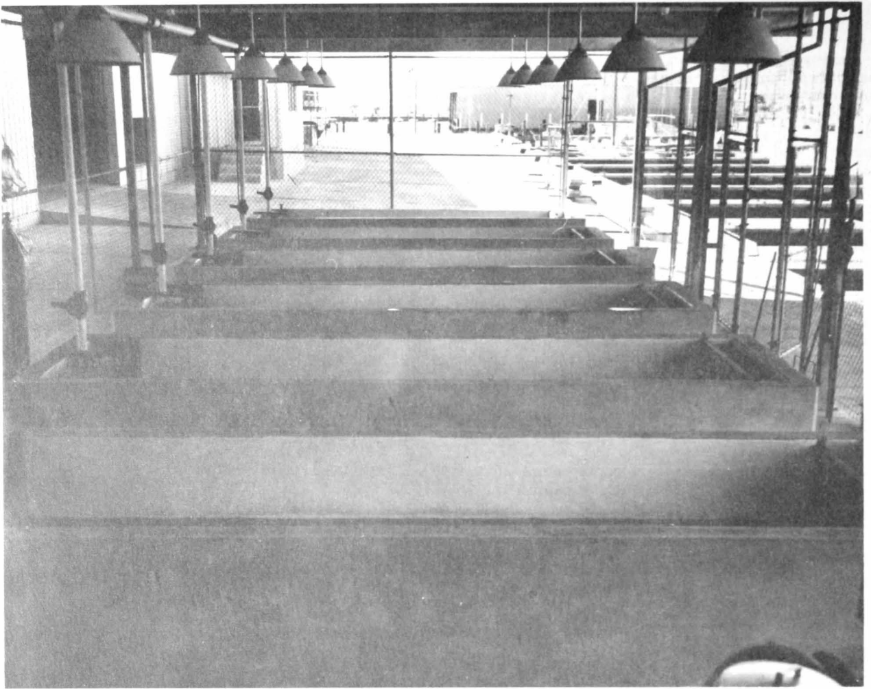
Figure 3.--Concrete holding tanks for bait shrimp.
