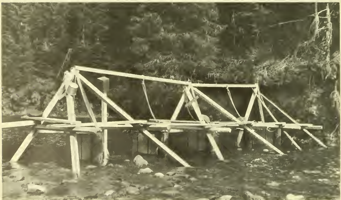
Figure 4.--Fry trap installation at Cannery Creek, showing method of hanging traps and spacing of traps across stream.
