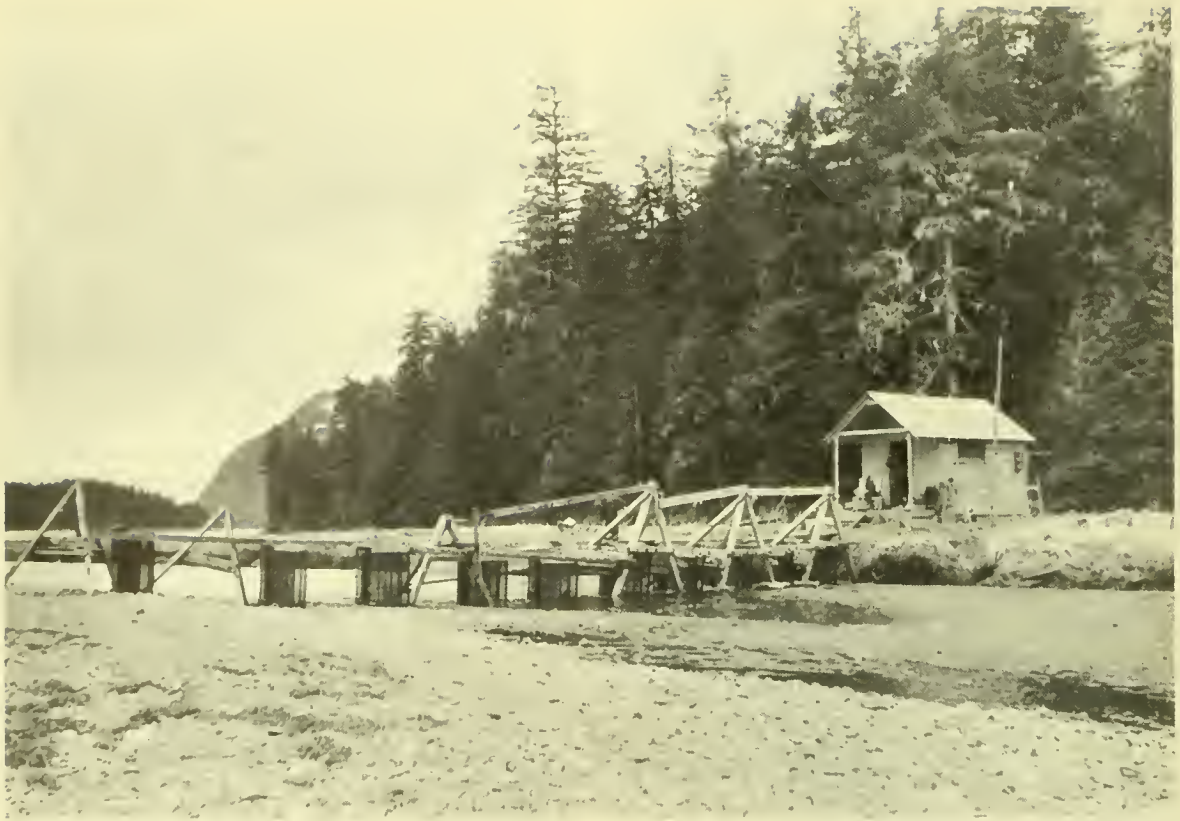
Figure 3.--Fry trap installation at Olsen Bay.
