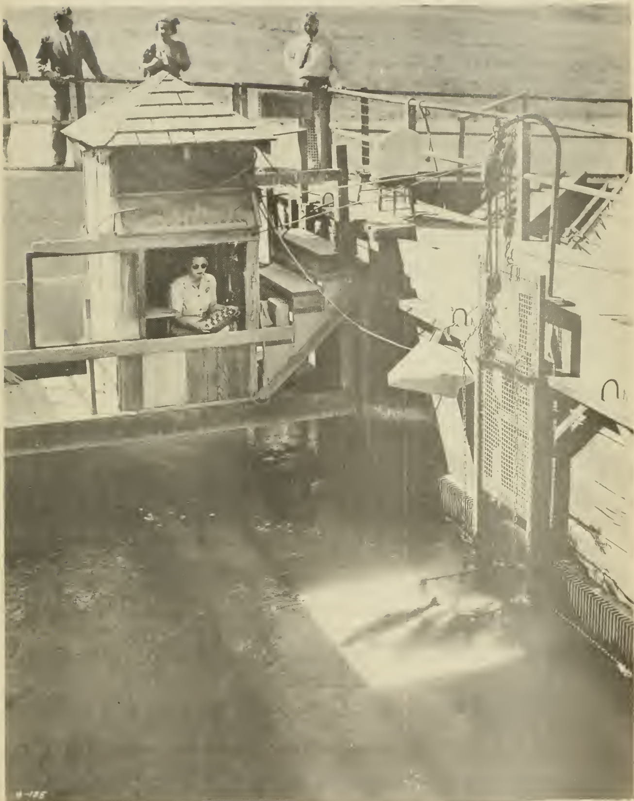
Fig. 4.--Counting station on Bradford Island fish ladder. (Photo by Corps of Engineers)
