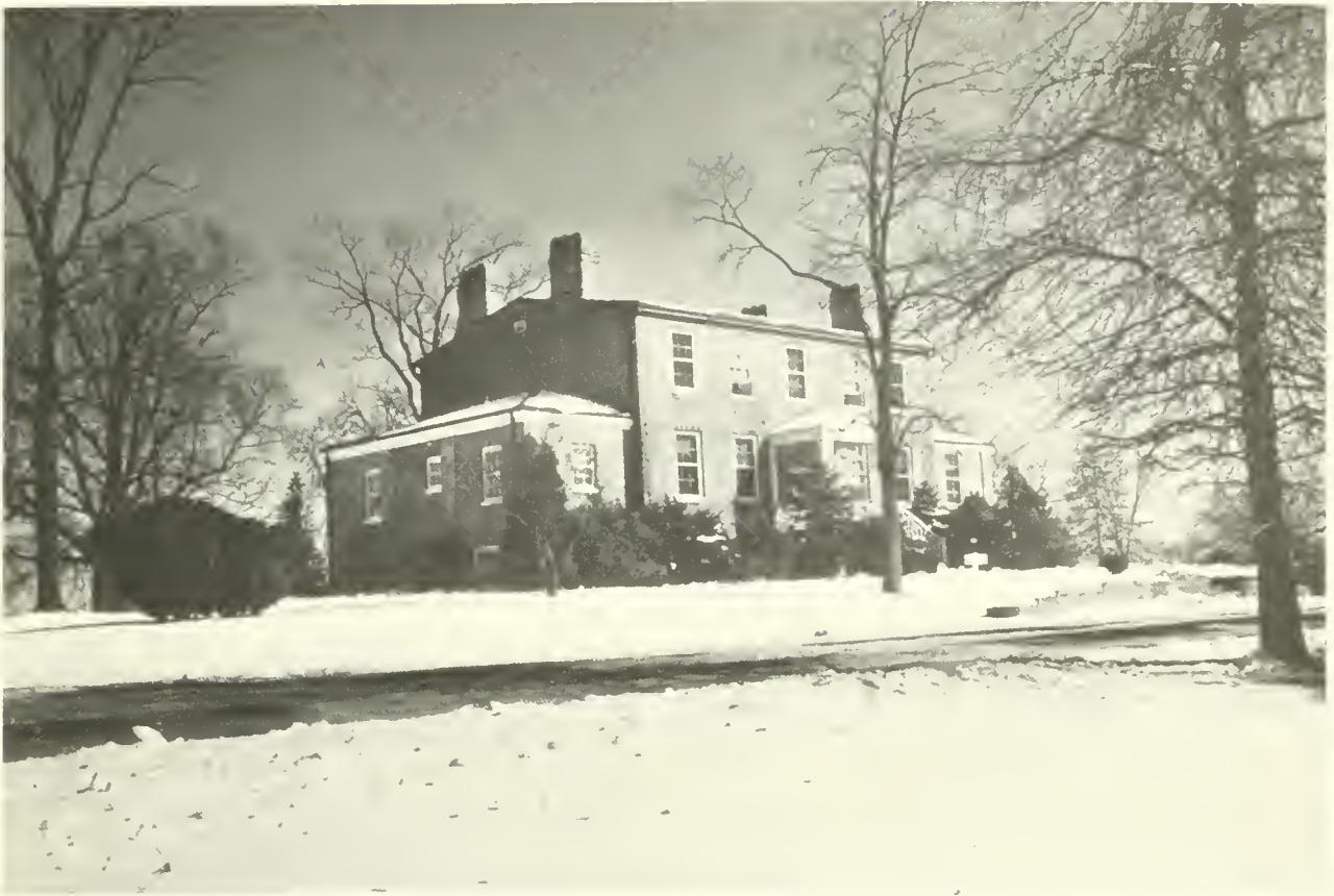
Snowden Hall—Colonial manor house built by the Snowden family over 200 years ago, now used as temporary office quarters.
