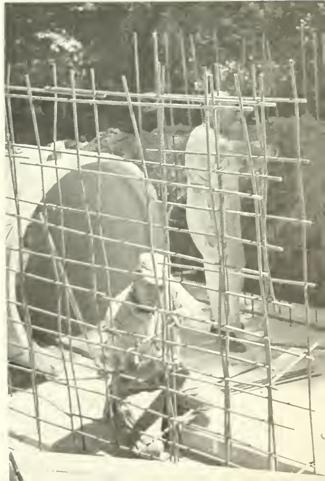
Building steel-reinforced concrete water-control structure for new waterfowl impoundment.
