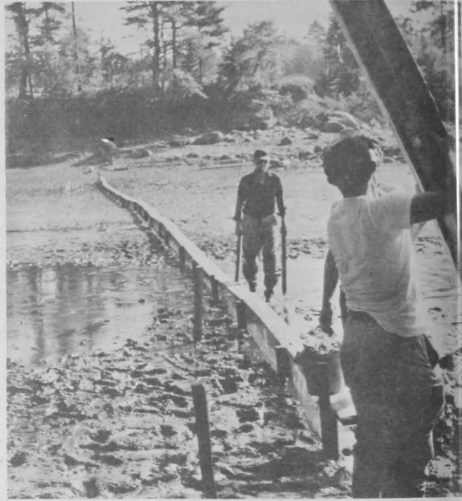
Installing fence across the constricted mouth of a cove to protect clam set from green-crab predation.
