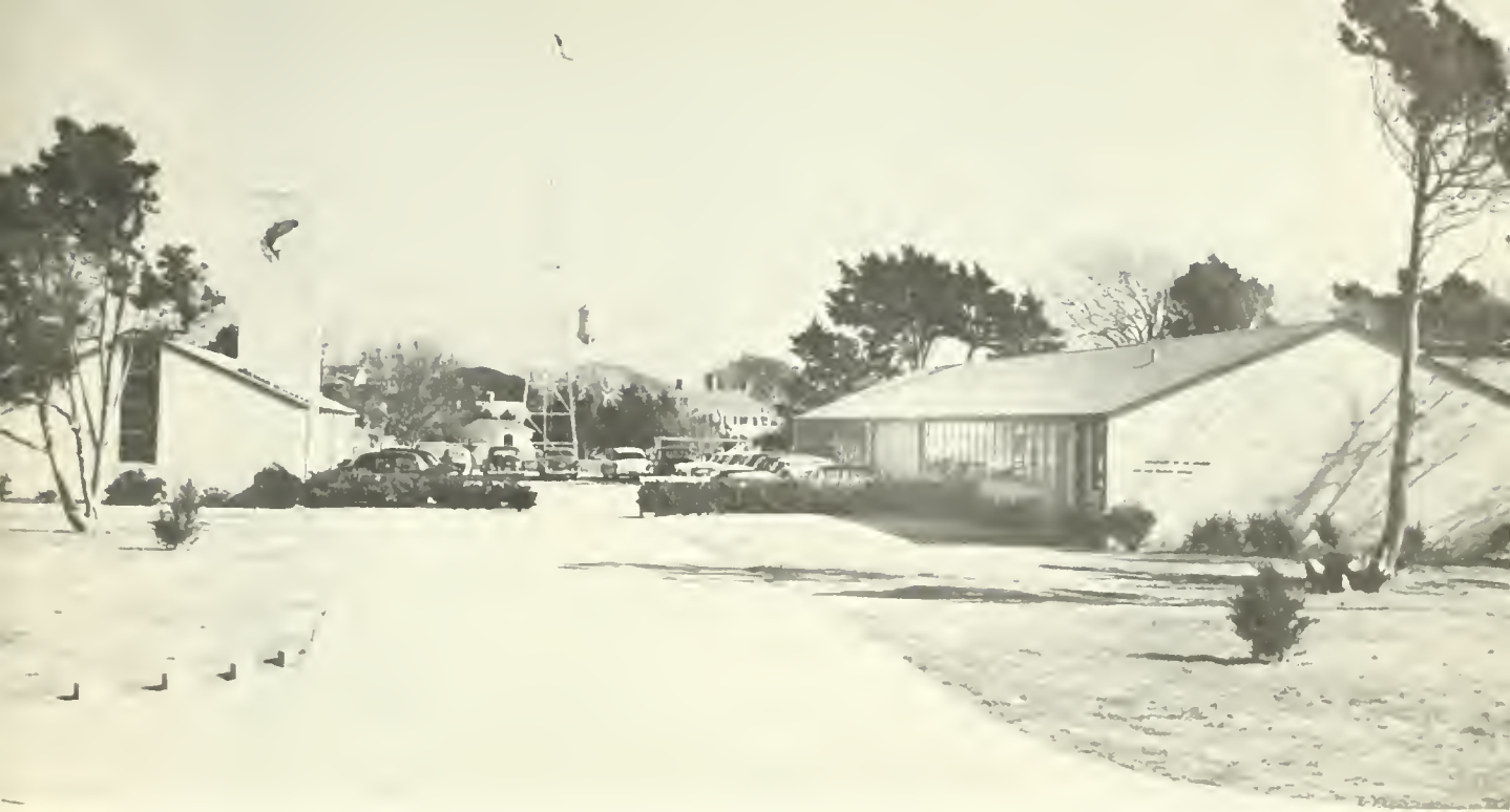
The fishery laboratory, service maintenance building, new concrete driveway and parking area. The maintenance building (on the left) houses the garage, shops, and pumping and heating facilities, and provides storage space
