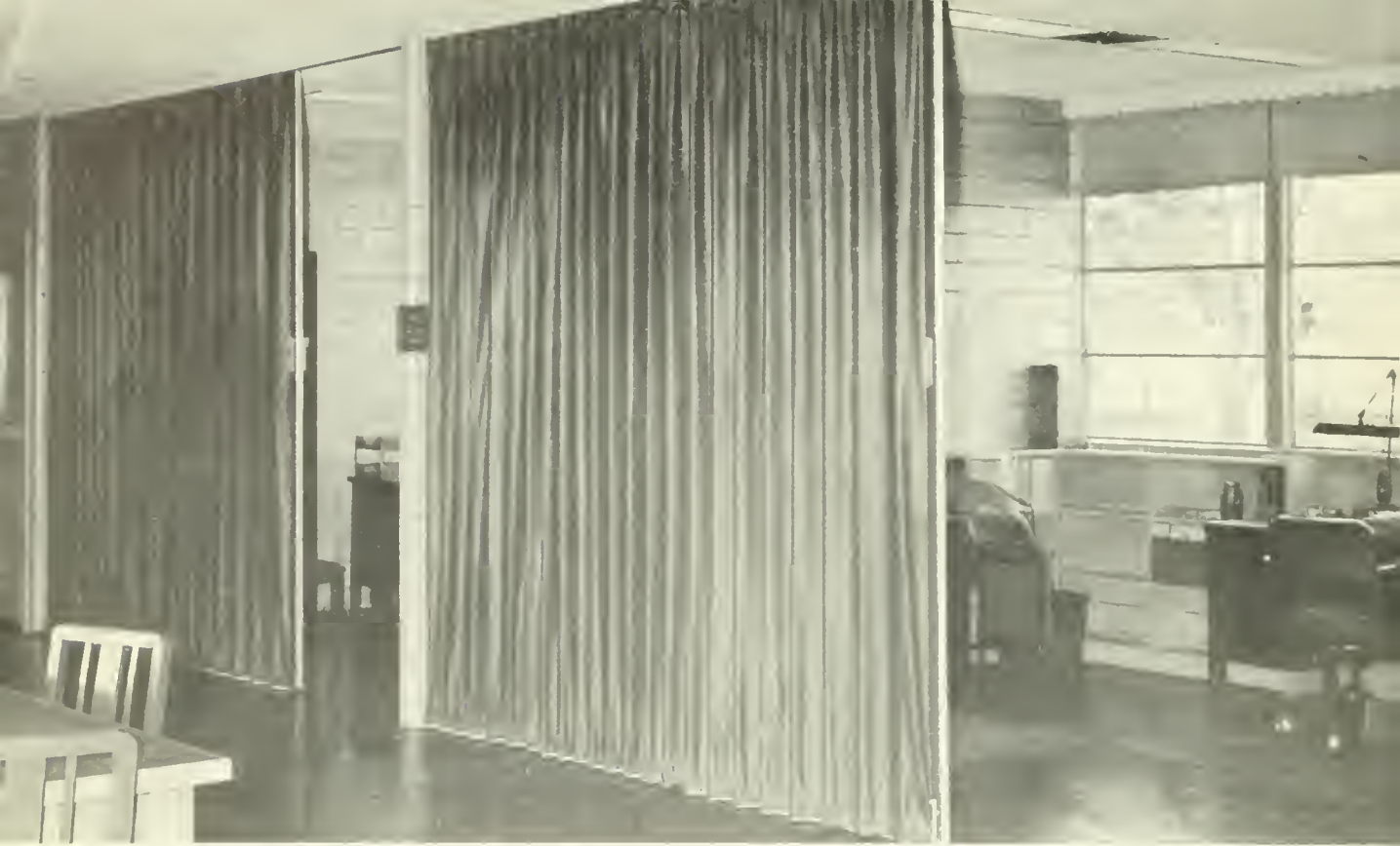
Folding doors between library and offices may be opened to provide a larger space for group meetings
