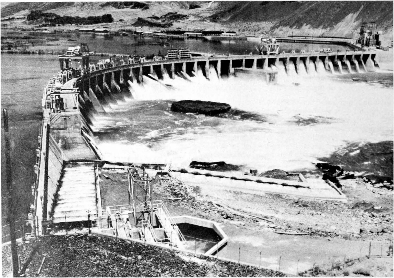
Figure 3.—Fish ladder (on near shore) at Rock Island Dam in Central Washington. Even with fish ladders, dams impede the passage of migratory fishes.
