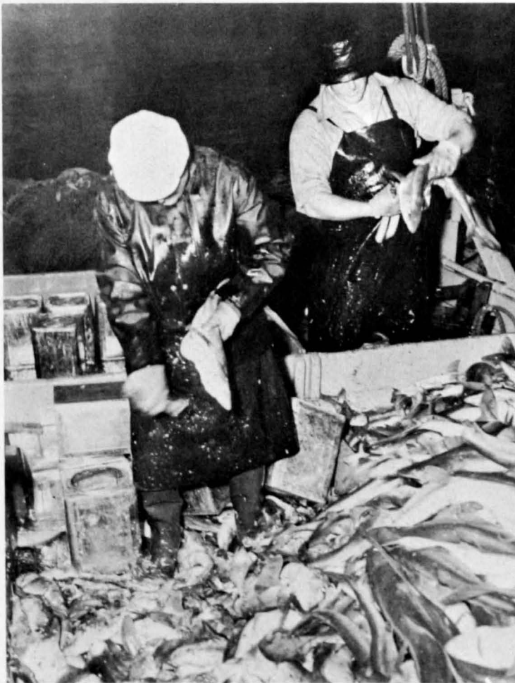
Figure 31.—Removing livers from grayfish. The livers are placed in 5-gallon cans to facilitate storage on the vessel and further handling.
