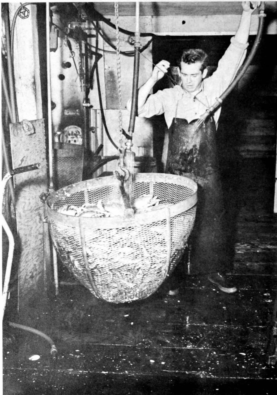
Figure 36.—Whole-cooked crab being rinsed and cooled after being cooked in brine water.
