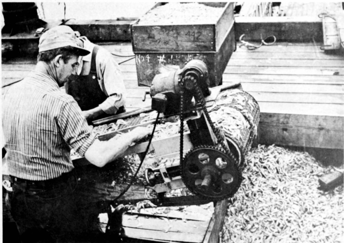
Figure 33.—Conveyor for use in grading pink shrimp by size.
