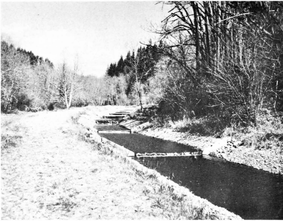
Figure 5.—Channel for incubating salmon eggs in Abernathy Creek near Longview, Washington, to evaluate rearing capacity and effects of environment on survival.
