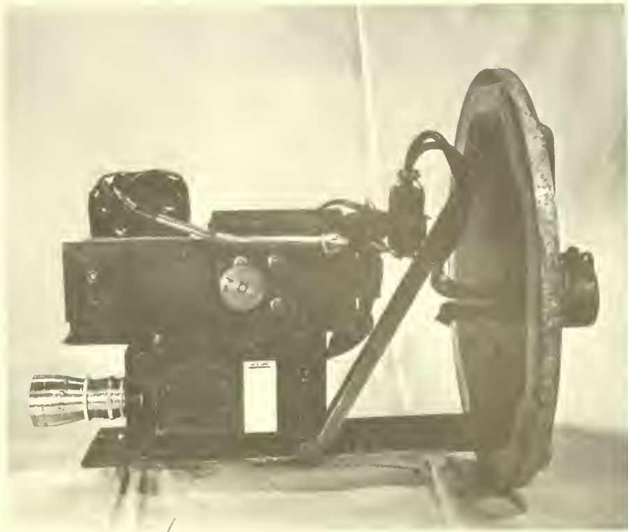
Figure 7.--Left side of large camera unit showing mounting plate, for power supply and take-up motor, bolted to camera top.
