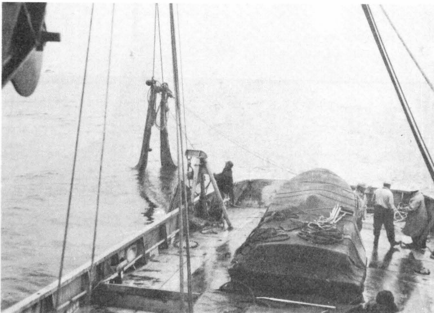
FIG. 11 - THE ELECTRIC BOOM WINCH IS USED TO PICK UP THE CABLE FROM THE NET WHILE THE VESSEL IS SWUNG TO THE STARBOARD.
