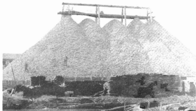
Figure 82.—Shell pile of a large Maryland oyster company, showing the conveyor for carrying shells from shucking tables to the pile (Churchill, 1921).
