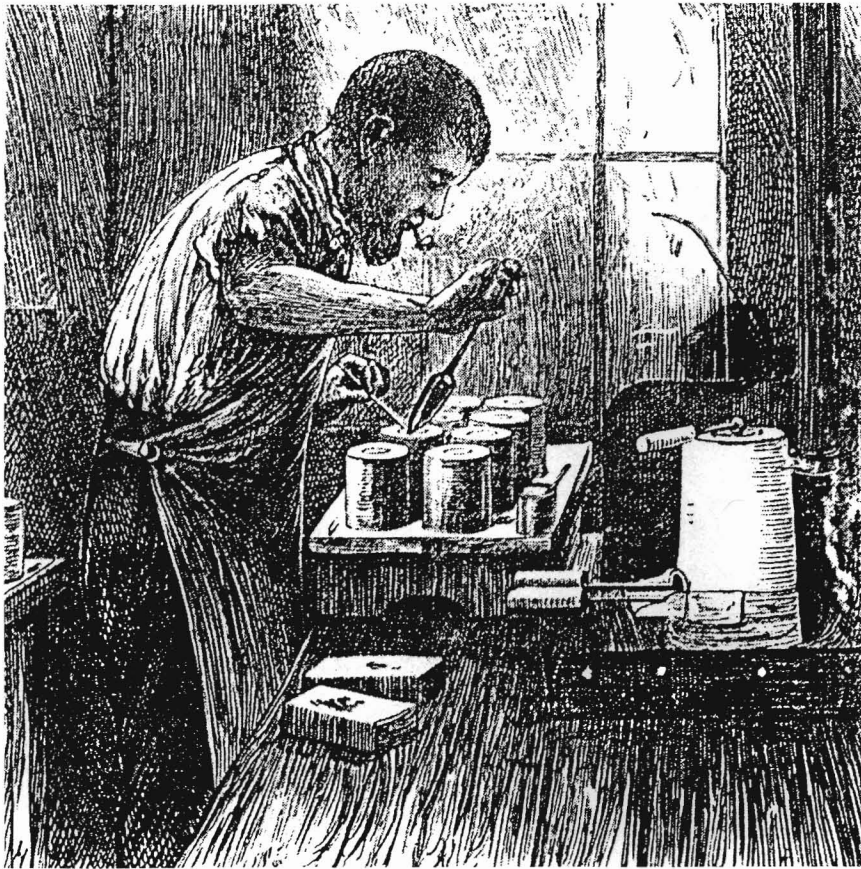
Figure 22.—Soldering the cans after the oyster meats have been placed in them. Source: Harper's Weekly , March 1872.
