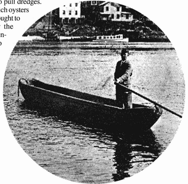
Figure 10.—This white pine dugout, 8.8 m (29 feet) long and 0.9 m (3 feet) wide, was the largest oyster boat in Connecticut in 1832. Dug out of a single log it was brought down from Lake Cayuga, N.Y., by water, and delivered in New Haven, Conn., for $42.00. Photograph provided by author; original source unknown.
