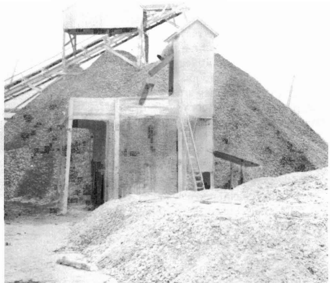
Figure 20.—Kiln for burning oyster shells to make lime, showing shell heap in background and pile of lime in foreground (Churchill, 1921).
