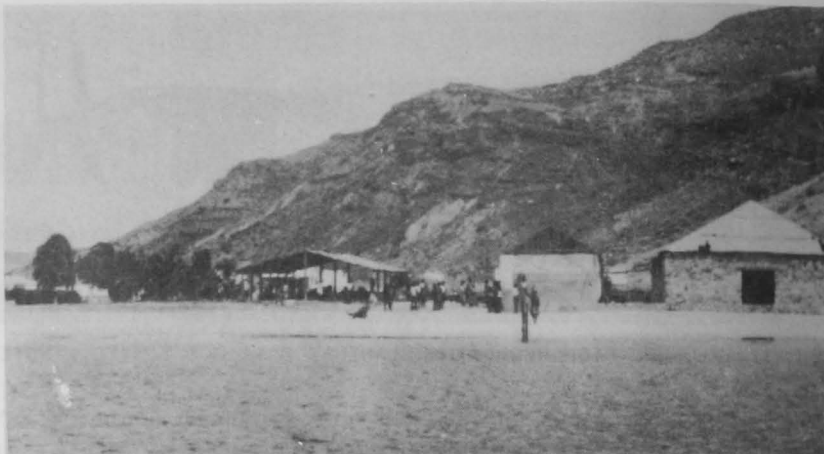
PART OF A FISH-HANDLING PLANT AT BAIJA DOS ELEFANTES. PRODUCTION IS PRINCIPALLY SALTED AND DRIED FISH, AND SOME MEAL AND OIL.
