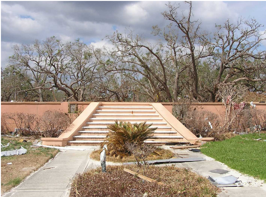
Figure 3.—Stairway to nothing is all that remains of a once substantial home in the Long Beach area of coastal Mississippi after Katrina, Oct. 2005. Photo: Palma Ingles.
