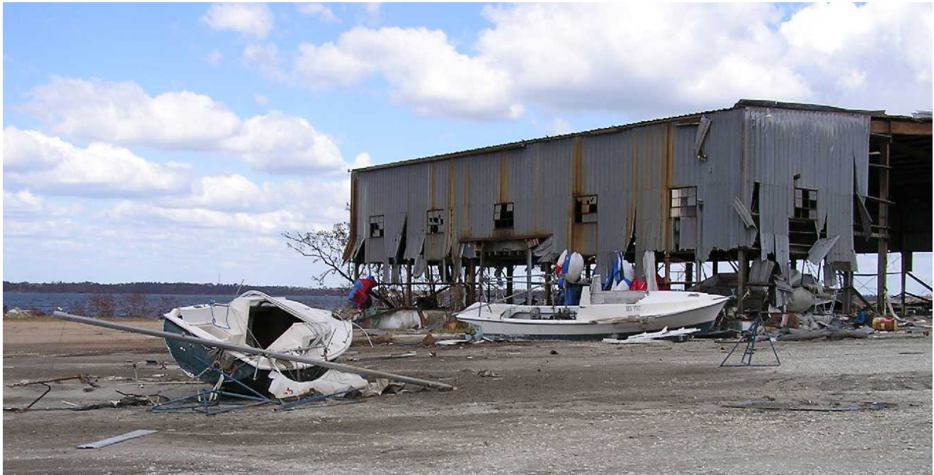
Figure 6.—Destroyed recreational boats and recreational boat storage facility, Biloxi, Miss., Oct., 2005. Photo: Palma Ingles.
