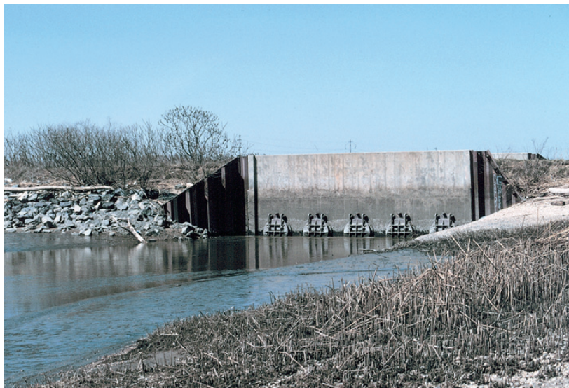
NOAA Restoration Center
