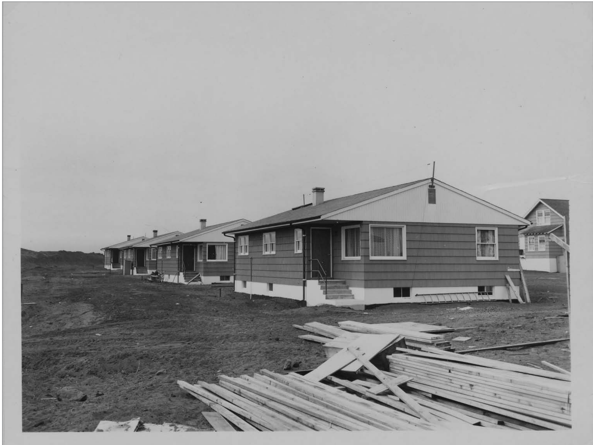
Photograph No. 95-ADMC-574 (Photographer unknown), 1966; Native housing construction, in view Aleut Laborer Houses 122–126, Aleut Laborer House 127 in progress. Records of the National Oceanic and Atmospheric Administration, RG 370; NARA—Pacific Alaska Region (A).
