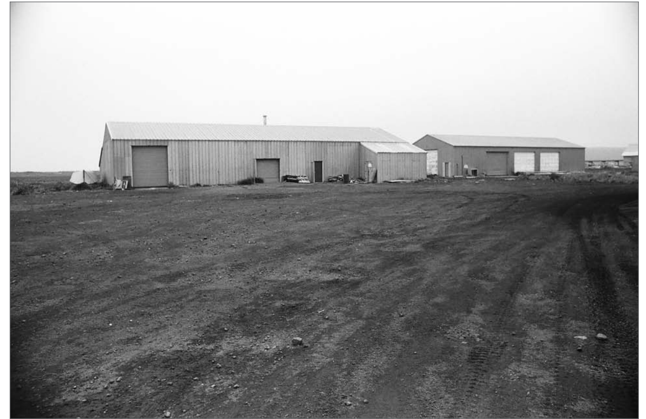
Photographer unknown. 1985. South and east sides, Combine Shop (left) and GARCO warehouse (right). Photograph. From Faulkner, 1986. Courtesy National Park Service, Anchorage, neg. file 01110031.
