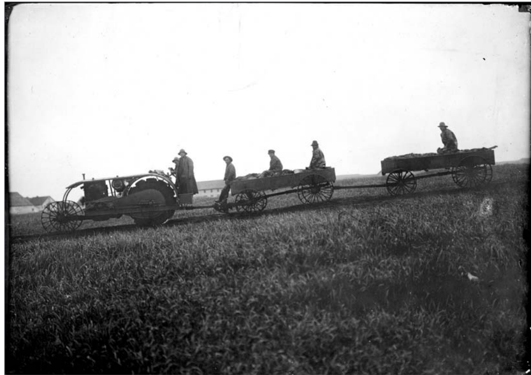
Photograph No. 22-MP-3-47 (Photographer unknown), circa 1918–1919; Tractor hauling wagons carrying sealskins. Seal carcasses and blubber were hauled by tractor to the By-Products Plant. Records of the National Oceanic and Atmospheric Administration, RG 370; NARA—Pacific Alaska Region (A).
