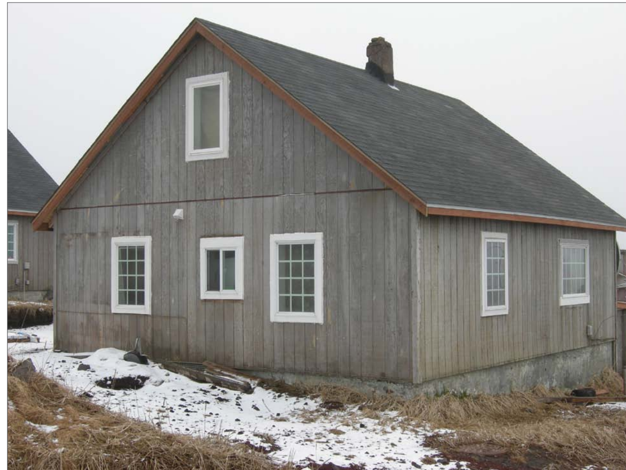
Mobley, Charles, photographer. 2007. West and south sides, Aleut Laborer House 30. Photograph (35mm). NOAA, NOS, Pribilof Project Office, Seattle.
