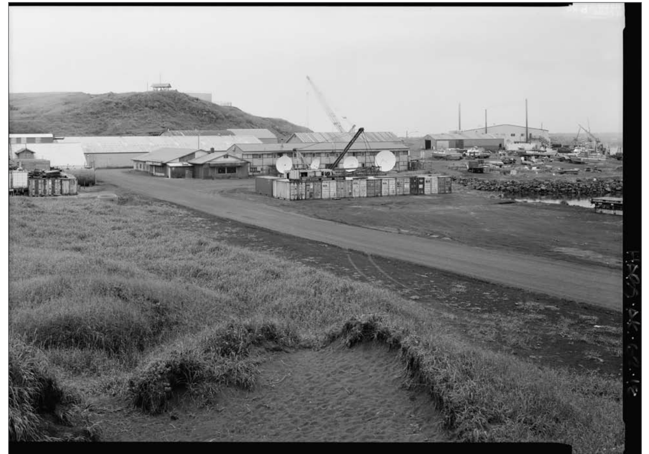
View showing Haul Road with Alaska Bunkhouse, Receiving Warehouse, boatyard, Trident Seafoods processing plant, and Village Hill gazebo in background. Jet Lowe, photographer. Photograph (5x7) . Library of Congress: HABS AK-62-18, 2004.
