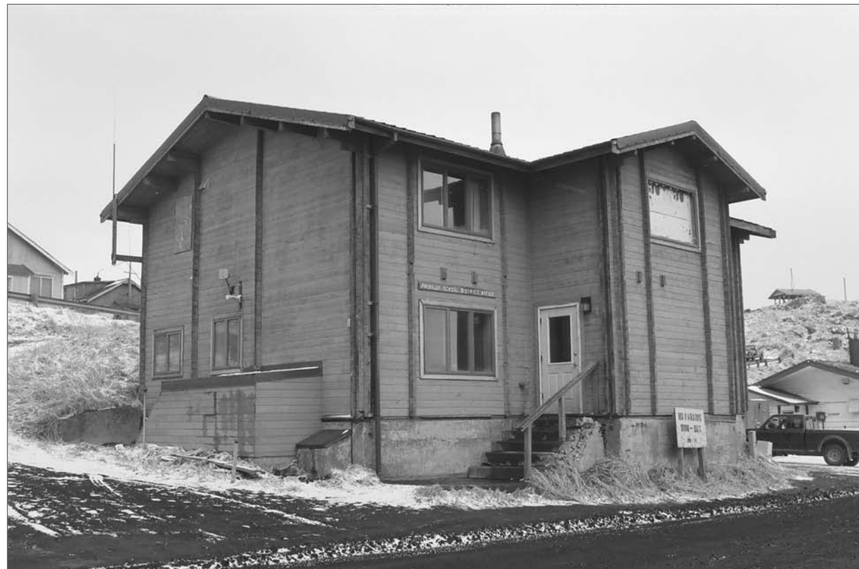
Mobley, Charles, photographer. 2007. East front and south side, School District Office. Photograph (35mm) . NOAA, NOS, Pribilof Project Office, Seattle.
