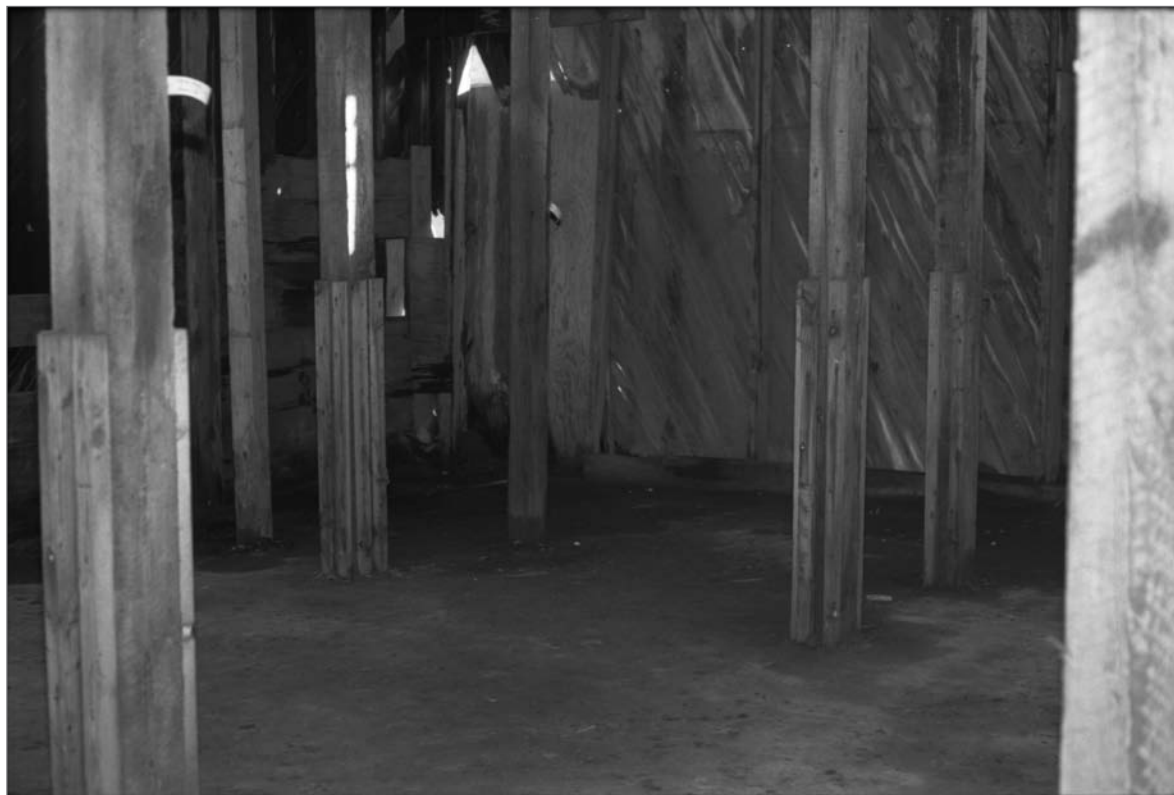
Young, Allison, photographer. 2000. Interior southwest wall, corner posts of kench; foreground two corner kench posts on southeast wall, 1st floor, Salthouse A. Photograph (35mm) . NOAA, NOS, Pribilof Project Office, Seattle: sheet JL 111379.1, neg. 4043.
