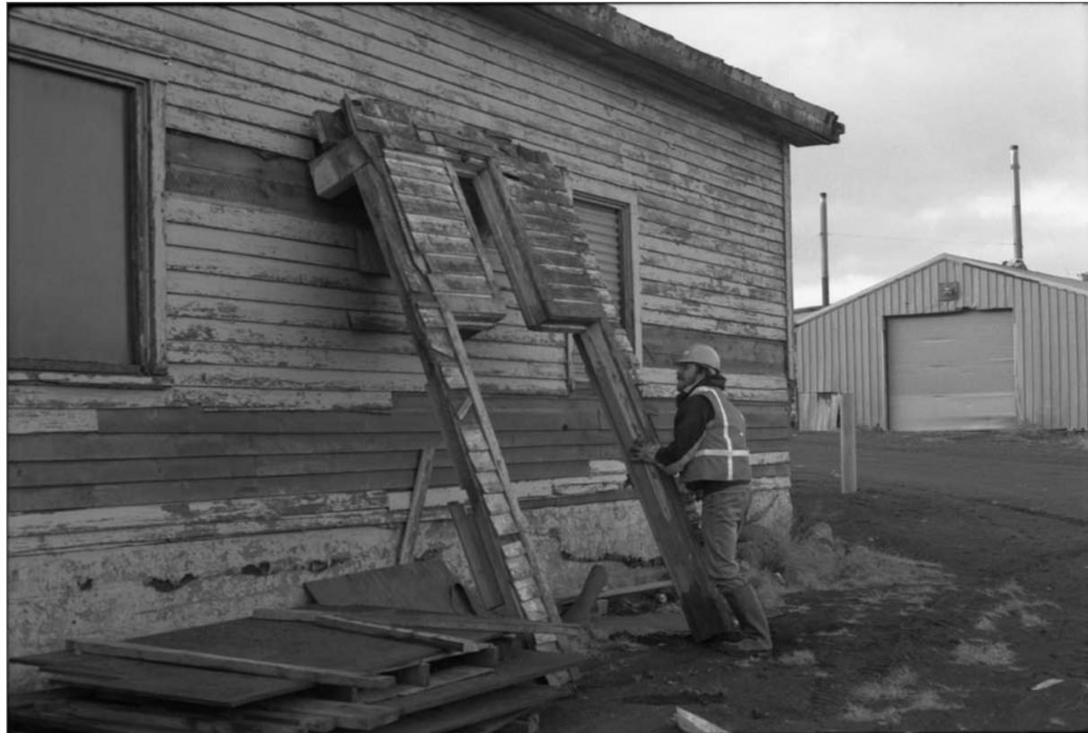
Young, Allison, photographer. 2000. Salthouse A, south end, Key-Hole door frame removed for archiving by the St. Paul Island Museum. Photograph (35mm). NOAA, NOS, Pribilof Project Office, Seattle: sheet JL 110929.1, neg. 4250.
