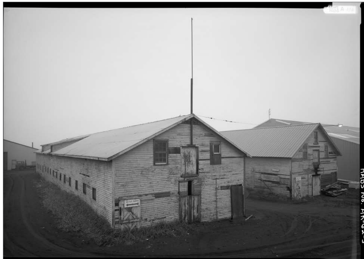
West and south sides, former Salthouse A/Boxing/Barreling Shed (left), Salthouse B (center), and Anderson Building (right). Jet Lowe, photographer. Photograph (5x7). Library of Congress: HABS AK-62-3, 1989.
