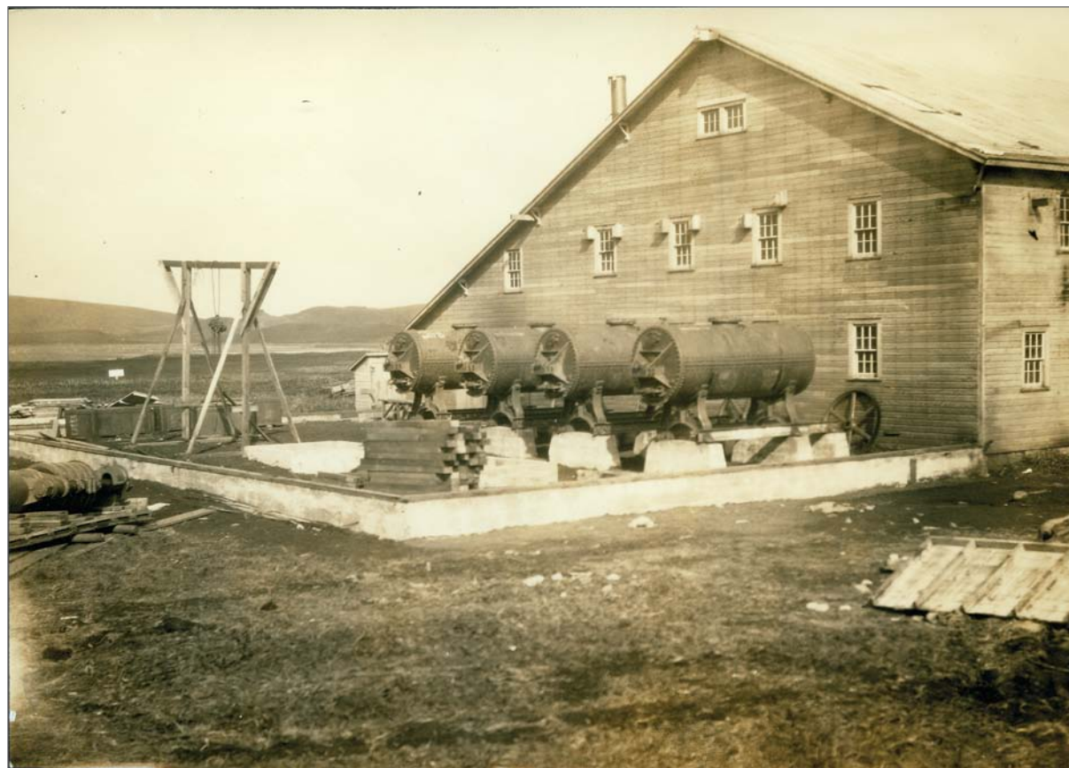
Chute, George Roger, photographer. Circa 1938–1940. East and south sides, By-Products Plant, showing four large digester tanks. Photograph. Washington State Historical Society, Tacoma, WA: S1991.51.2.399.
