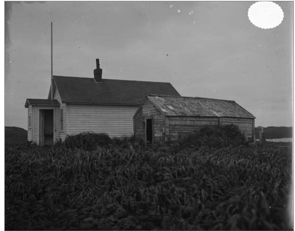
Photograph No. USBF 1.95 (Photographer G Dallas Hanna), 1915; Former Webster House and another building at Northeast Point. Records of the National Oceanic and Atmospheric Administration, RG 370; NARA—Pacific Alaska Region (A).
