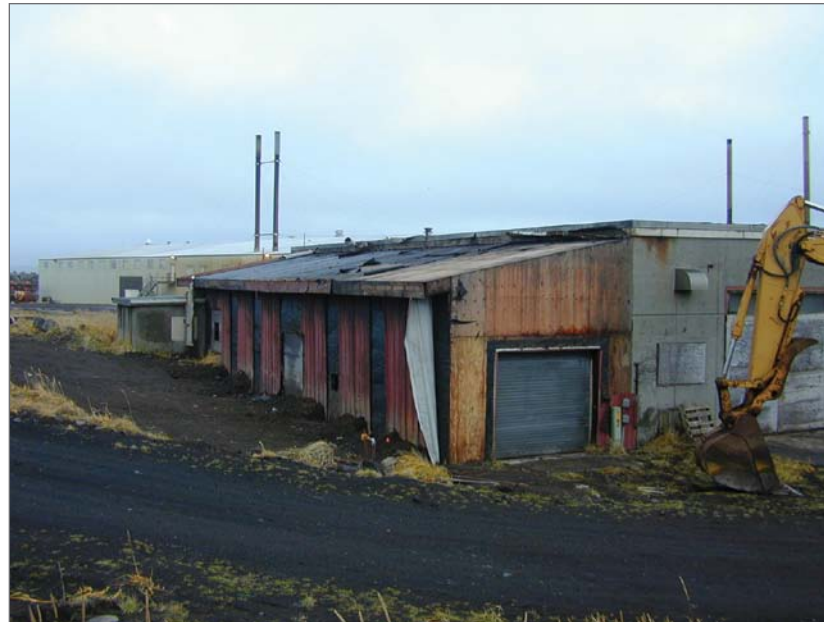
Photographer unknown. 2002. East and south sides, former Power Plant. Photograph (digital). NOAA, NOS, Pribilof Project Office, Seattle.
