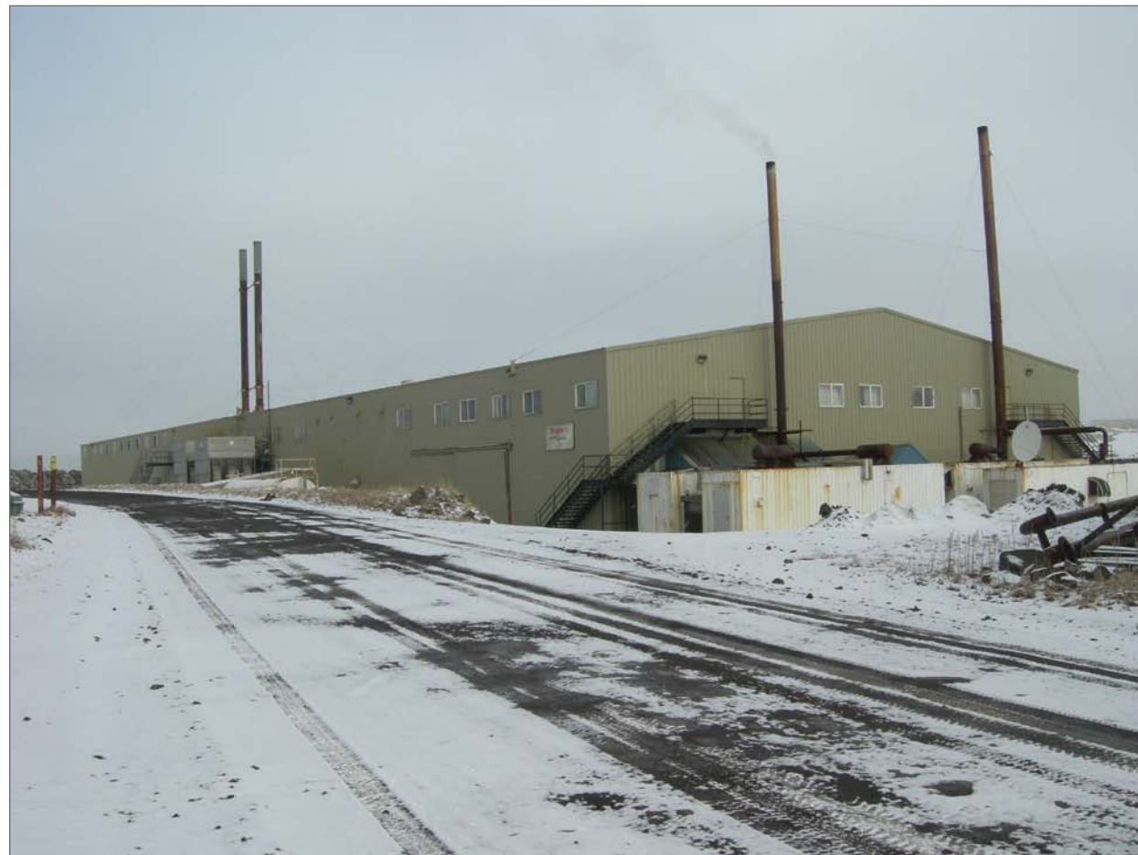
Mobley, Charles, photographer. 2007. South and east sides, Fish Plant/Trident Building. Photograph (35mm). NOAA, NOS, Pribilof Project Office, Seattle.
