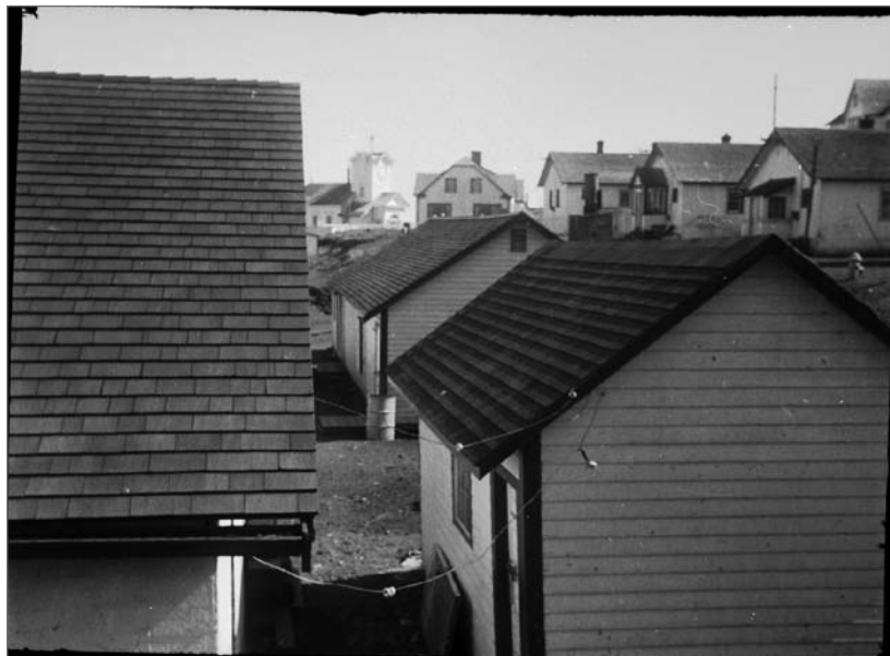
Photograph No. 95-ADMC-2368 (Photographer unknown), 1930's–1970's; Houses in St. Paul Village, looking north northeast, showing wash houses. Records of the National Oceanic and Atmospheric Administration, RG 370; NARA—Pacific Alaska Region (A).
