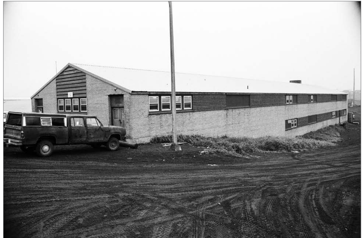
Brodherson, photographer. 1985. North front and south side, Community Store/Warehouse/Laboratory "Block 14 lot 3 and general store." Photograph. From Faulkner, 1986. Courtesy National Park Service, Anchorage, neg. file 01090014.
