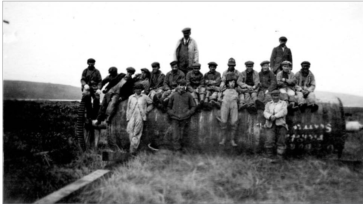
Photograph No. 22-MP-3-17 (Photographer unknown), 1918; Men sitting on By-Products Plant boiler. Records of the National Oceanic and Atmospheric Administration, RG 370; NARA—Pacific Alaska Region (A).
