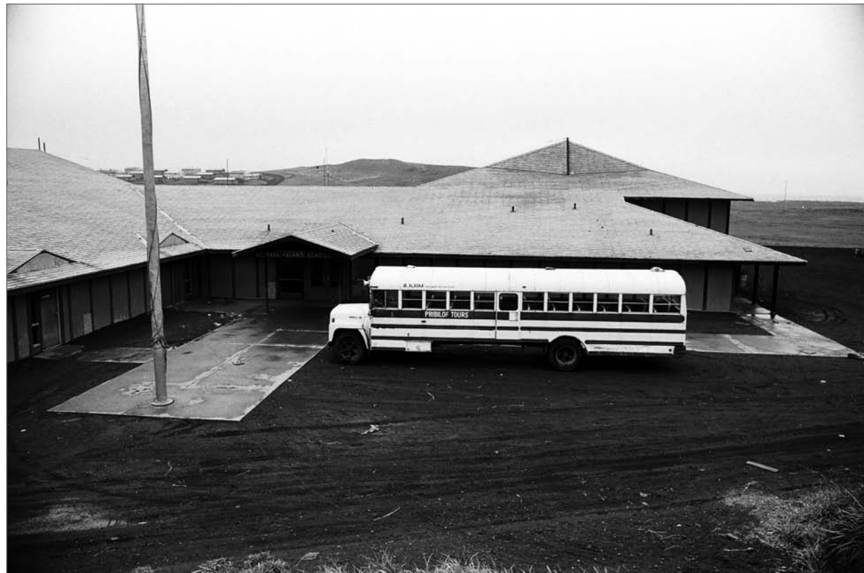
Brodherson, photographer. 1985. St. Paul Elementary and Junior High School Building. Photograph. From Faulkner, 1986. Courtesy National Park Service, Anchorage, neg. file 01090035.
