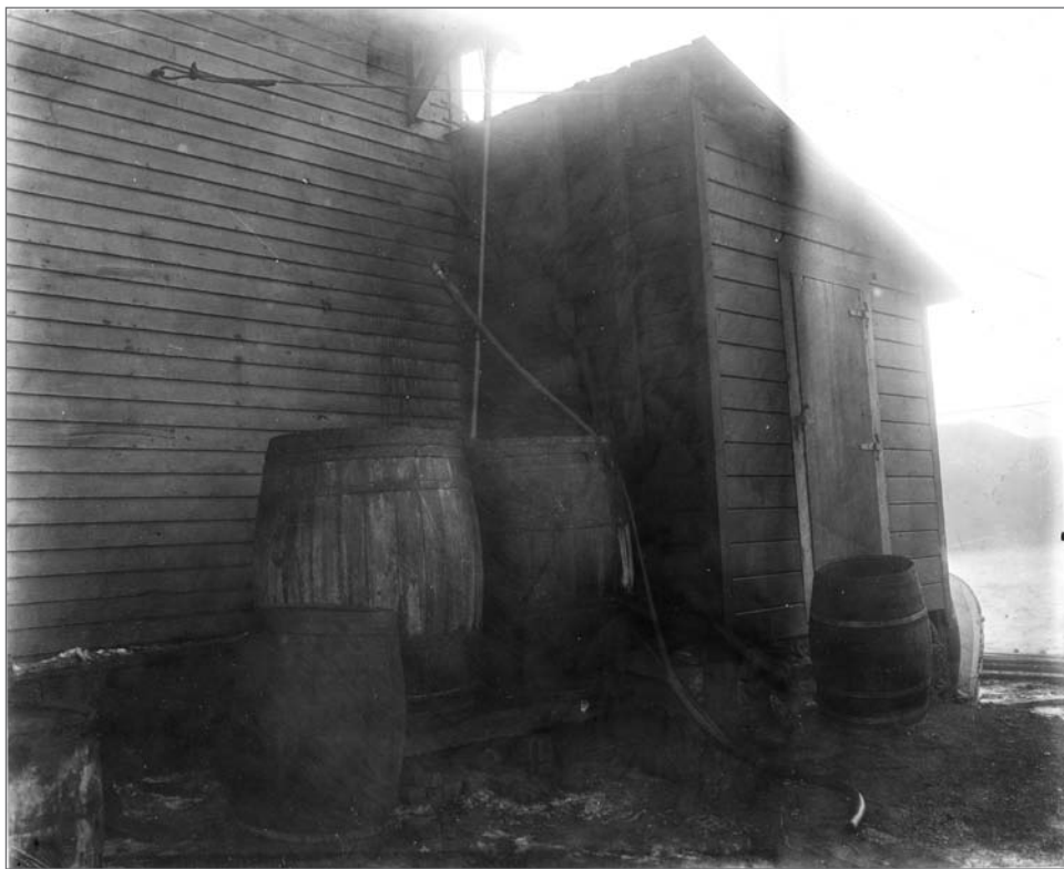
Photograph No. USBF 1.99 (Photographer unknown), circa 1914; Water barrels next to building. Records of the National Oceanic and Atmospheric Administration, RG 370; NARA—Pacific Alaska Region (A).
