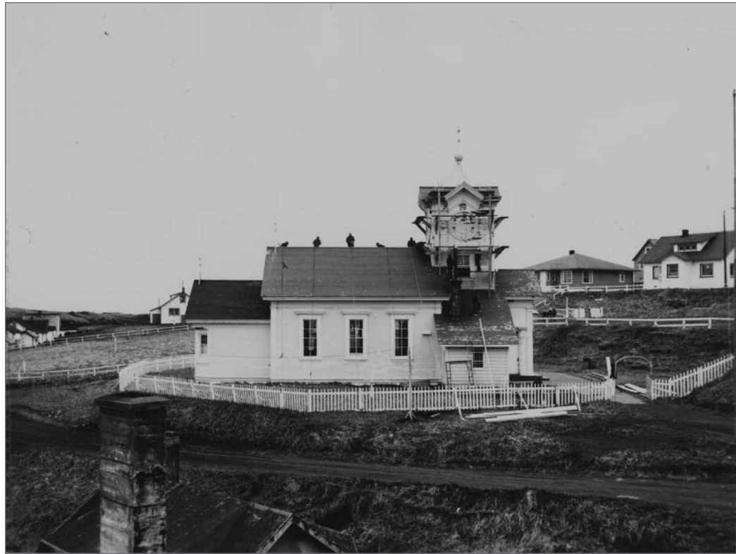
Photograph No. 95-ADMC-3191 (Photographer unknown), June 1972; North side, Crew performing restoration work on Church of the Holy Apostles Saints Peter and Paul. Records of the National Oceanic and Atmospheric Administration, RG 370; NARA—Pacific Alaska Region (A).
