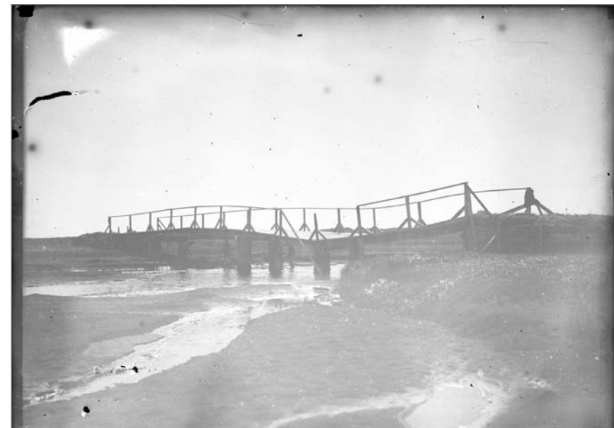
Photograph No. USBF 2.47 (Photographer Hanna, G Dallas), 1919; Bridge at Halfway Point (Polovina). The 103-foot long bridge was constructed in 1911 using two stumps of the USRC Perry's masts, part of its deck, and driftwood logs. The 24- and 20-inch bolts used on the bridge were handmade by Native workmen on St. Paul. The Perry ran aground on St. Paul Island on July 27th, 1910. Records of the National Oceanic and Atmospheric Administration, RG 370; NARA—Pacific Alaska Region (A).
