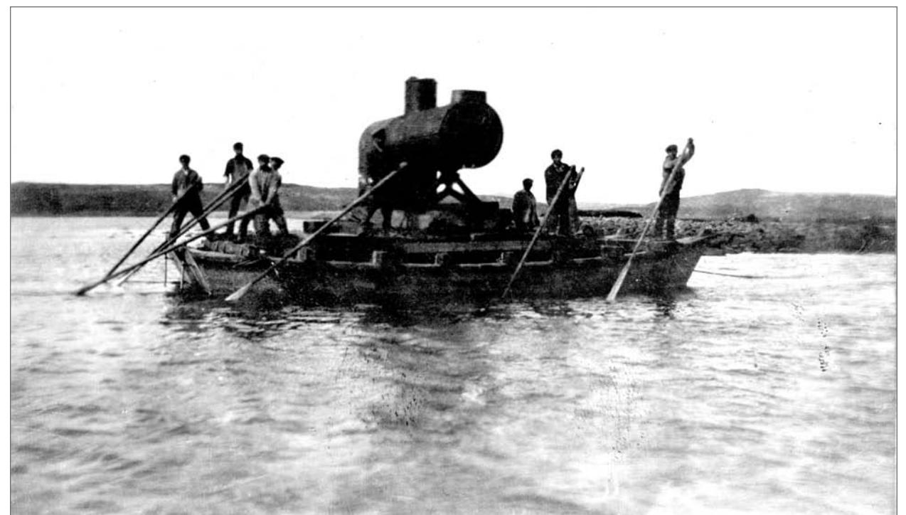
Photograph No. 22-MP-3-15 (Photographer unknown), 1918; Men transporting boiler for By-Products Plant up Salt Lagoon channel. Records of the National Oceanic and Atmospheric Administration, RG 370; NARA—Pacific Alaska Region (A).
