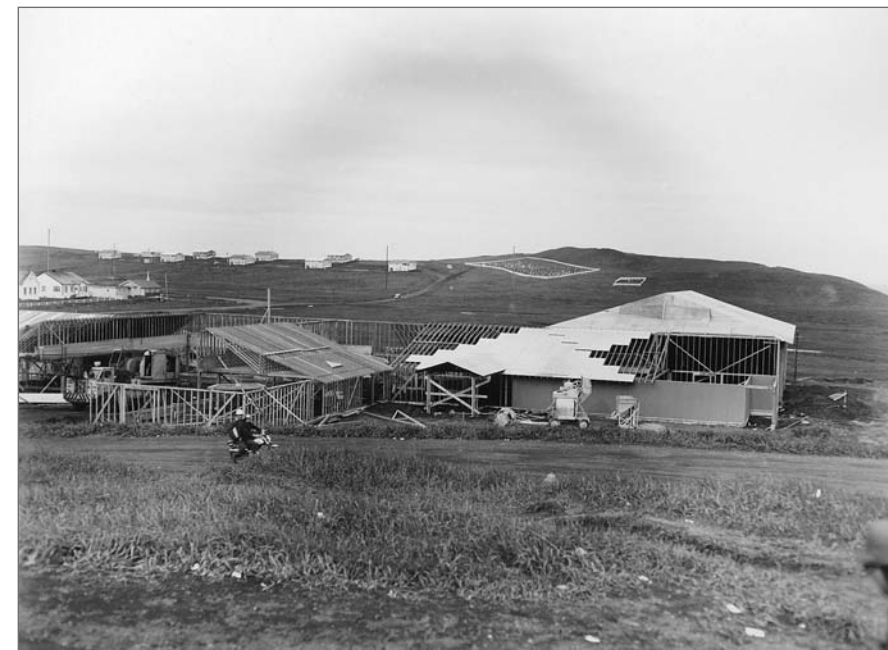
Photograph No. 95-ADMC-2175 (Photographer unknown), 1972; Construction of St. Paul Elementary and Junior High School Building. Records of the National Oceanic and Atmospheric Administration, RG 370; NARA—Pacific Alaska Region (A).
