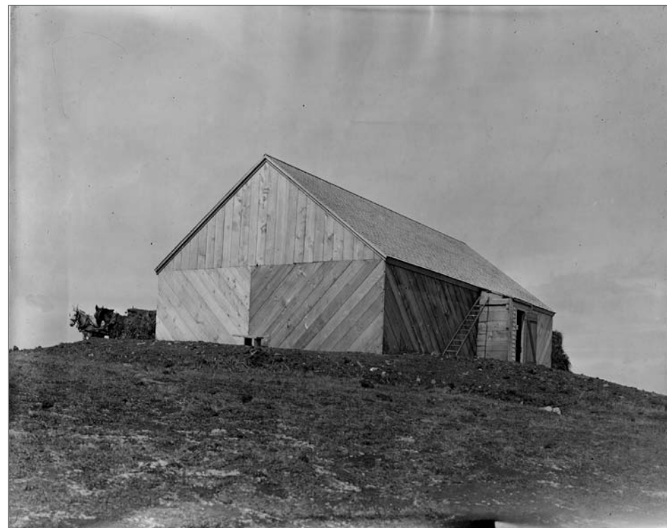
Photograph No. 95-ADMC-2902 (Photographer unknown), circa 1912; Tank House on Village Hill, showing completed construction and draft team hauling sod. NARA incorrectly identifies this as “stable with horses.” Records of the National Oceanic and Atmospheric Administration, RG 370; NARA—Pacific Alaska Region (A).
