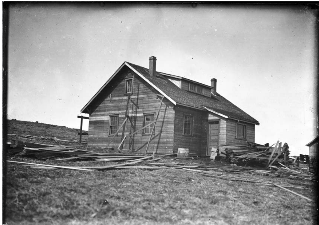
Photograph No. USBF 2.66 (Photographer G Dallas Hanna), September 1918; Southwest side and southeast front, Cottage "A" under construction in St. Paul Village. Plans for these new houses included a kitchen, living room, bathroom, and three bedrooms on the first floor. Government agents modified the plans to permit addition of extra bedrooms in the upper story. RG 370; NARA—Pacific Alaska Region (A).
