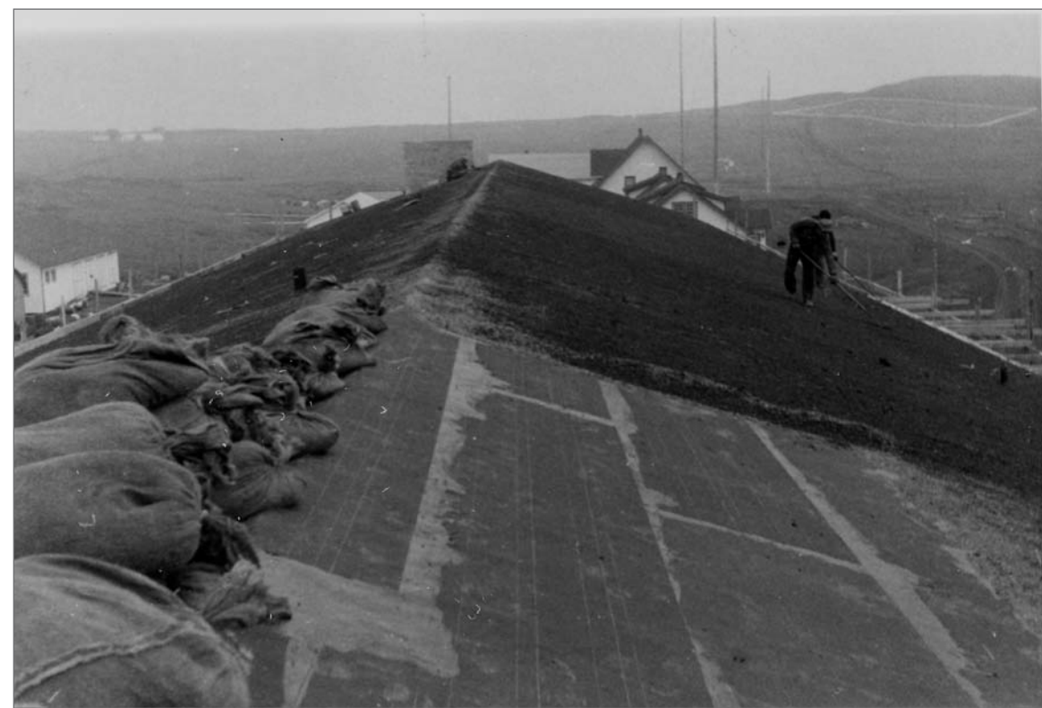
Photograph No. 95-ADMC-2010 (Photographer unknown), 1950's; Tarring roof, Community Store/Warehouse/Laboratory being tarred, looking east. Records of the National Oceanic and Atmospheric Administration, RG 370; NARA—Pacific Alaska Region (A).
