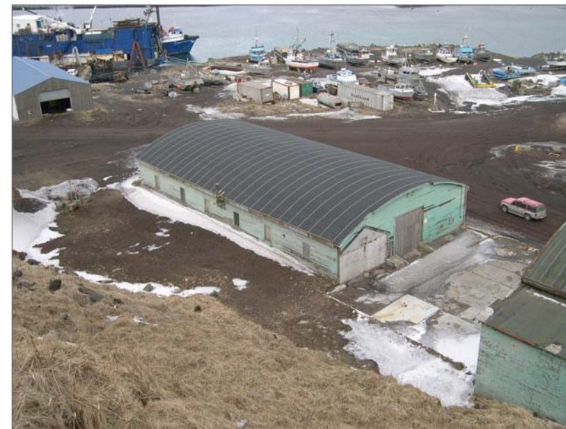
Photographer unknown. Circa 2006. Equipment Garage (left) and Machine Shop (right), following 2006 demolition of central addition (Connector Building), looking north northeast. Photograph (digital) . NOAA, NOS, Pribilof Project Office, Seattle.
