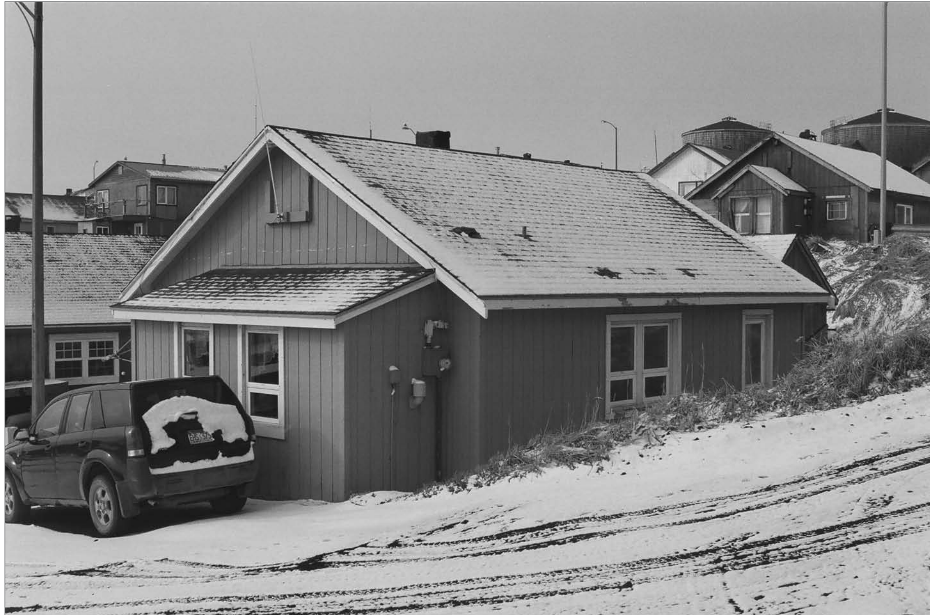
Mobley, Charles, photographer. 2007. East front and north side, Aleut Laborer House 6. Photograph (35mm) . NOAA, NOS, Pribilof Project Office, Seattle.
