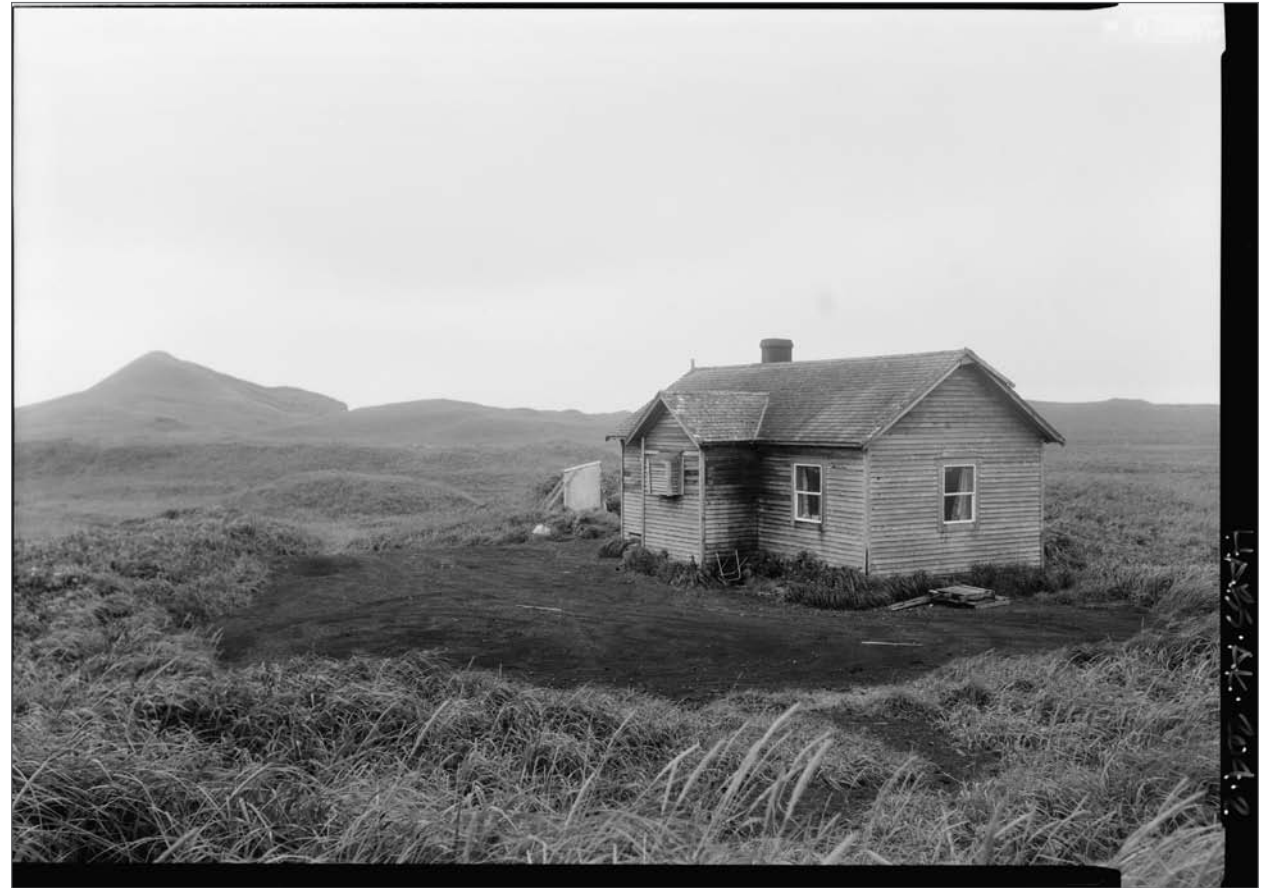
East front and north side, Webster House, looking northwest. Jet Lowe, photographer. Photograph (5x7). Library of Congress: HABS AK-204-2, 2004.
