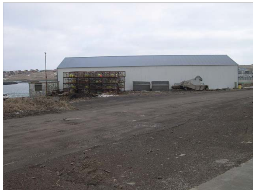
Winandy, David B., photographer. March 21, 2006. Receiving Warehouse. Photograph (digital). NOAA, NOS, Pribilof Project Office, Seattle.
