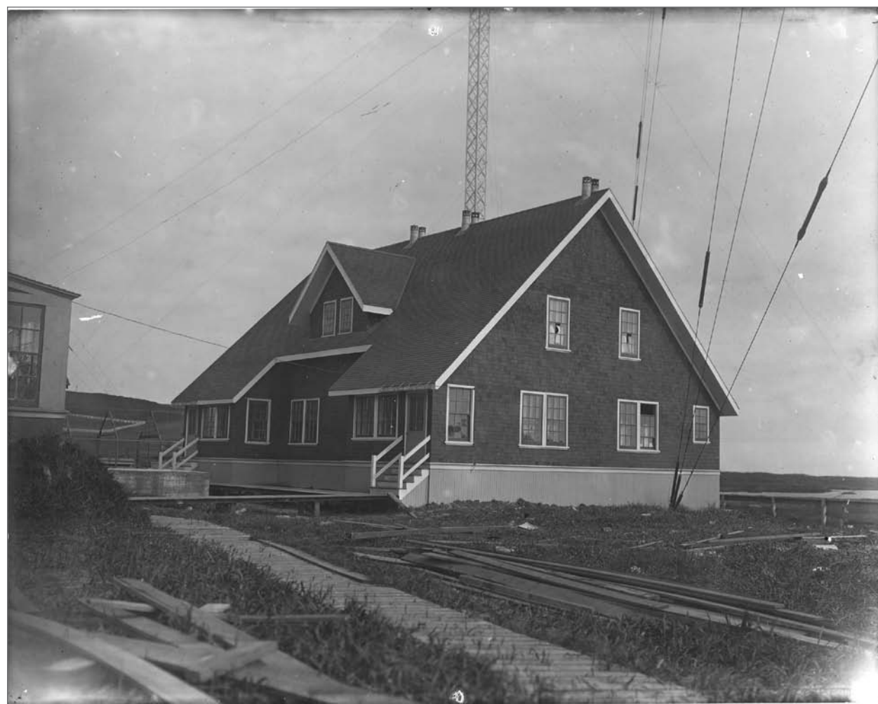
Photograph No. USBF 1.84 (Photographer G Dallas Hanna), 1919; North front and west side, Duplex 106/107, newly built, at Naval Radio Station. Records of the National Oceanic and Atmospheric Administration, RG 370; NARA—Pacific Alaska Region (A).
