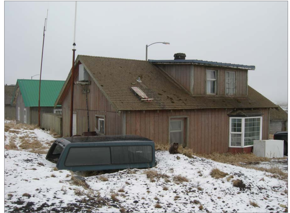
Mobley, Charles, photographer. 2007. West and south sides, Aleut Laborer House 20. Photograph (35mm) . NOAA, NOS, Pribilof Project Office, Seattle.
