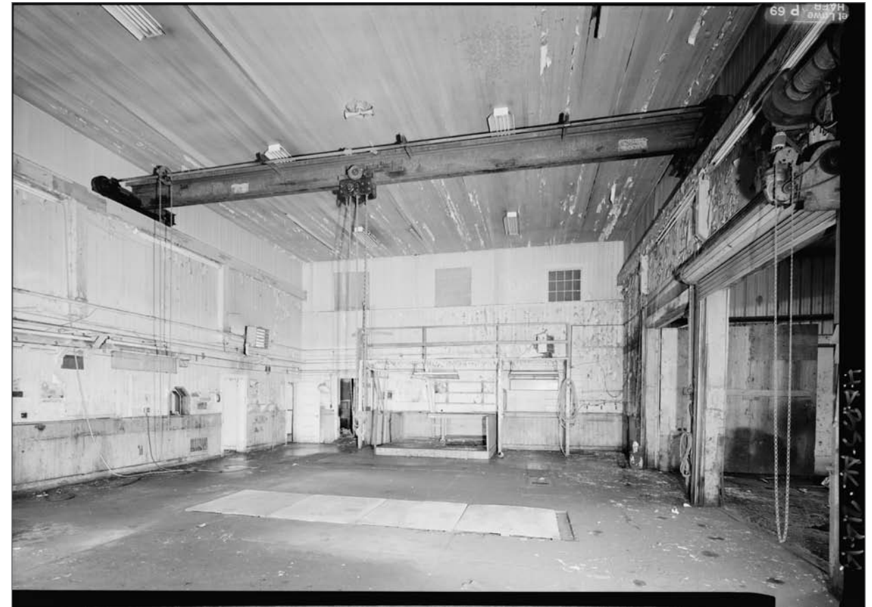
Interior, Machine Shop, showing bridge crane, looking south. Jet Lowe, photographer. Photograph (5x7). Library of Congress: HABS AK-214-14 , 2004.
