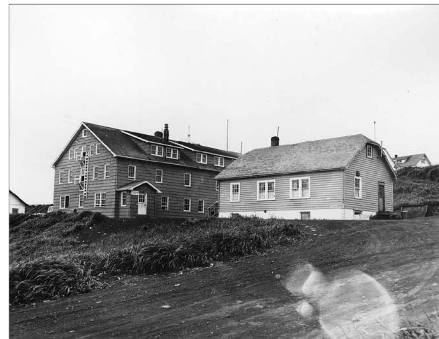
Photograph No. 95-ADMC-434 (Photographer unknown), n.d.; East and north sides, Fisheries Office, with Company House/King Eider Hotel in the background (left). Records of the National Oceanic and Atmospheric Administration, RG 370; NARA—Pacific Alaska Region (A) .
