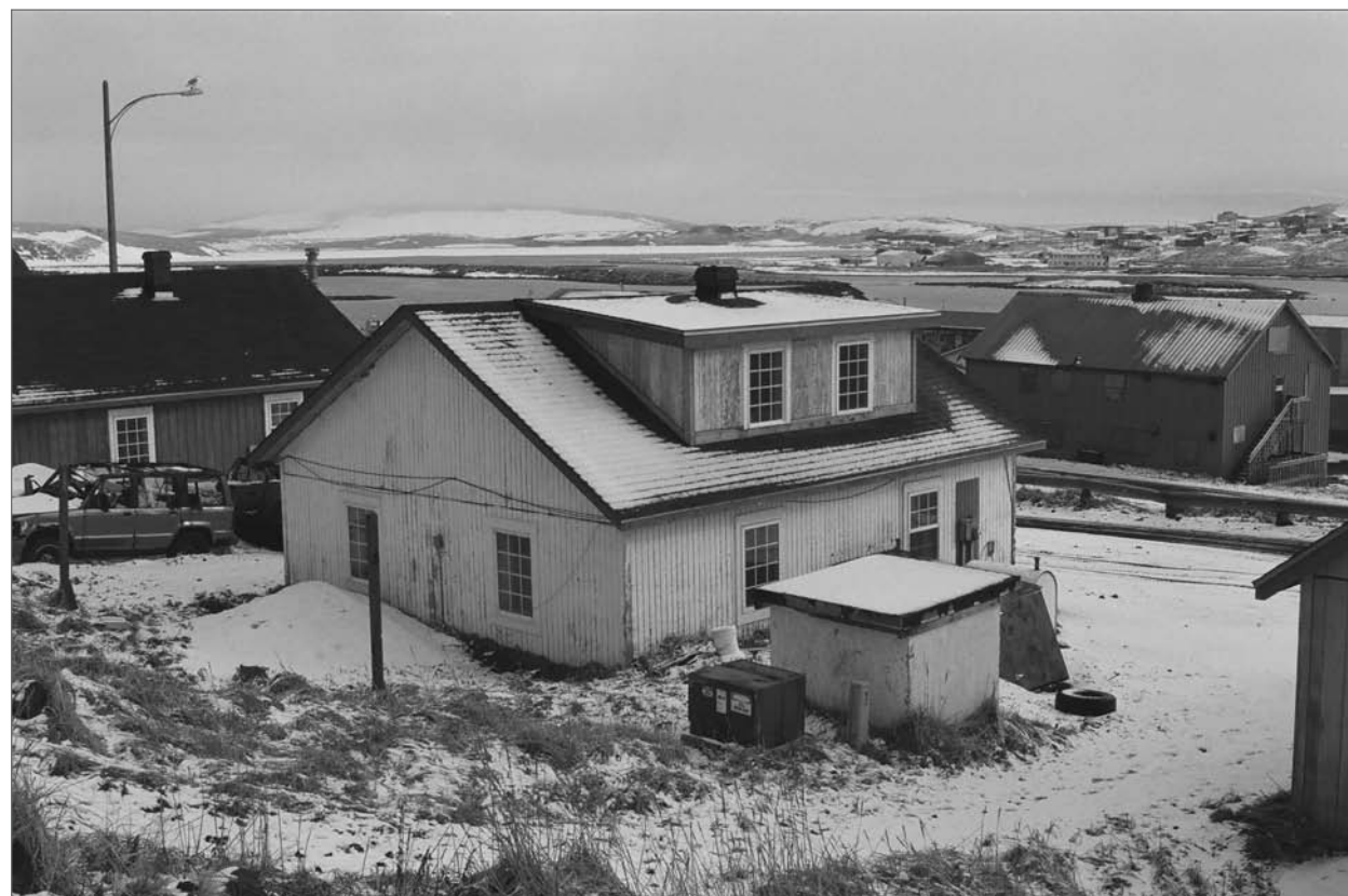
Mobley, Charles, photographer. 2007. West and south sides, Aleut Laborer House 4. Photograph (35mm) .
