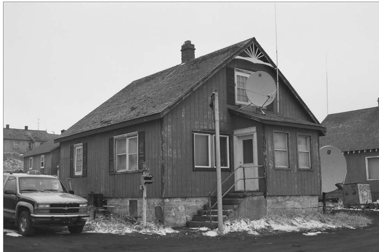
Mobley, Charles, photographer. 2007. South side and east front, Aleut Laborer House 56. Photograph (35mm) . NOAA, NOS, Pribilof Project Office, Seattle.
