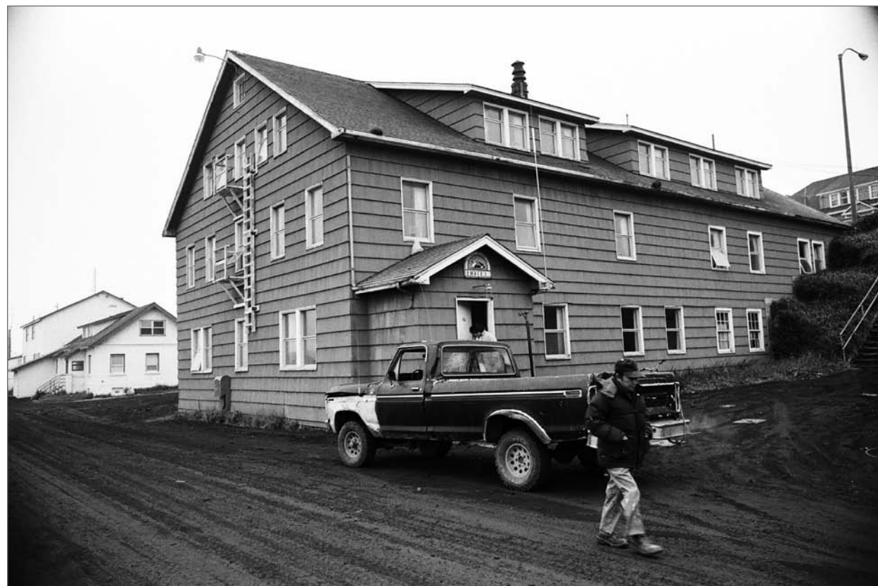
Brodherson, photographer. 1985. East side and north front, King Eider Hotel, formerly called the Company House "Block 18 lot 4, King Eider." Photograph. From Faulkner, 1986. Courtesy National Park Service, Anchorage, neg. file 01090031.
