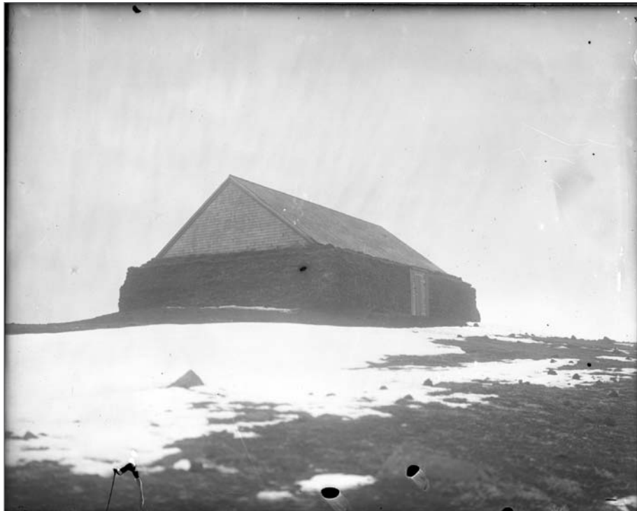
Photograph No. USBF 1.65 (Photographer G Dallas Hanna), 1912; Tank House on Village Hill, insulated with sod. Records of the National Oceanic and Atmospheric Administration, RG 370; NARA—Pacific Alaska Region (A).
