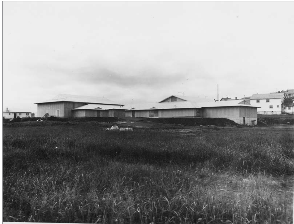
Photograph No. 95-ADMC-1706 (Photographer unknown), circa 1973; St. Paul Elementary and Junior High School Building. Records of the National Oceanic and Atmospheric Administration, RG 370; NARA—Pacific Alaska Region (A).
