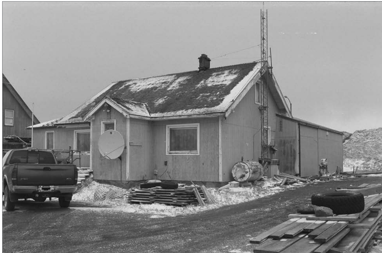
Mobley, Charles, photographer. 2007. South front and east side, House 105. Photograph (35mm) . NOAA, NOS, Pribilof Project Office, Seattle.
