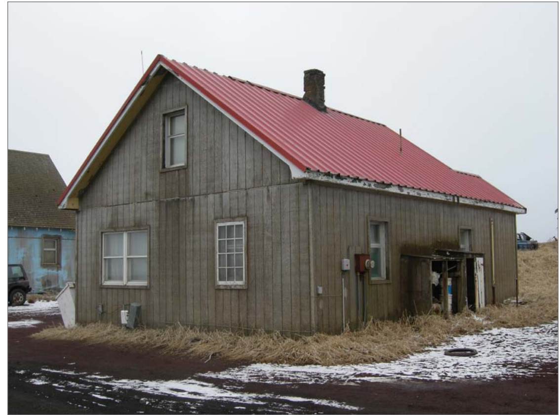
Mobley, Charles, photographer. 2007. East and north sides, Aleut Laborer House 42. Photograph (35mm). NOAA, NOS, Pribilof Project Office, Seattle.
