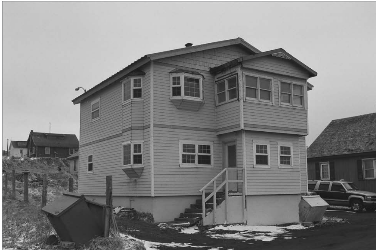
Moble, Charles, photographer. 2007. South side and east front, Aleut Laborer House 55. Photograph (35mm) . NOAA, NOS, Pribilof Project Office, Seattle.
