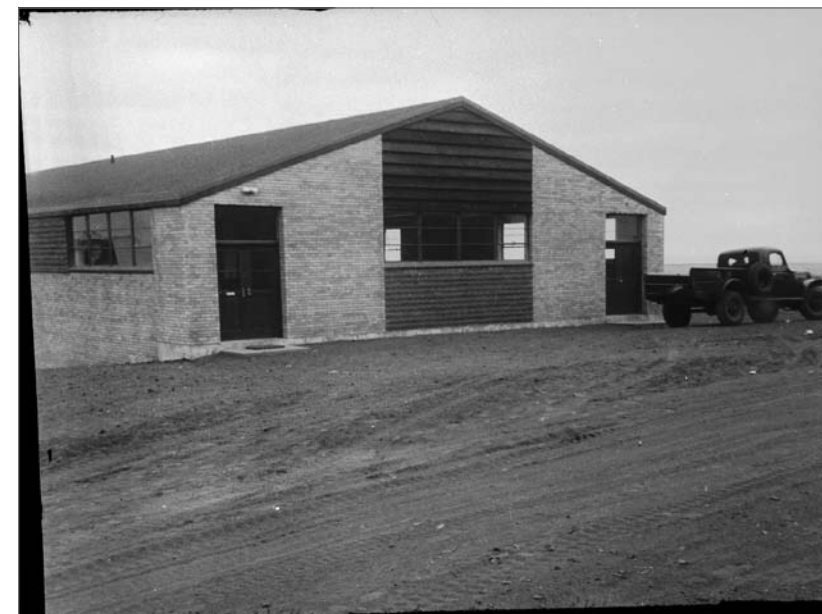
Photograph No. 95-ADMC-2355 (Photographer unknown), 1950's; North side and west front, Community Store/Warehouse/Laboratory. Records of the National Oceanic and Atmospheric Administration, RG 370; NARA—Pacific Alaska Region (A).
