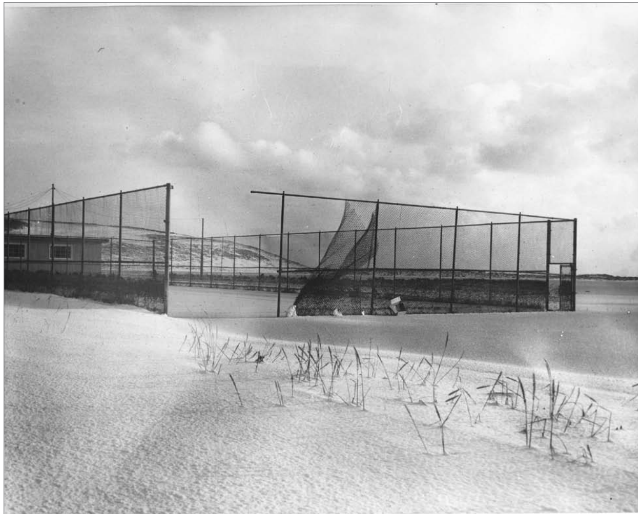
Photograph No. 95-ADMC-569 (Photographer unknown), December 1966 (Gregorian calendar); Flooded tennis court at Naval Radio Station, looking east. Records of the National Oceanic and Atmospheric Administration, RG 370; NARA—Pacific Alaska Region (A).
