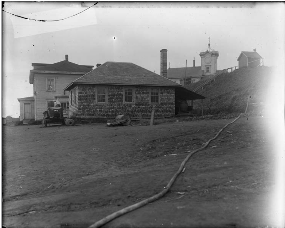
Photograph No. USBF 1.59 (Photographer G Dallas Hanna), circa 1912; Above-ground water line pipe next to shingled building, with Company House and Church of the Holy Apostles Saints Peter and Paul in background. Records of the National Oceanic and Atmospheric Administration, RG 370; NARA—Pacific Alaska Region (A).
