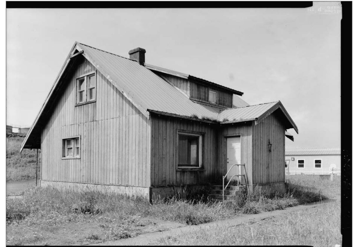
South side and east front, Teacher House 101. Jet Lowe, photographer. Photograph (5x7). Library of Congress: HABS AK-206-1, 2004.
