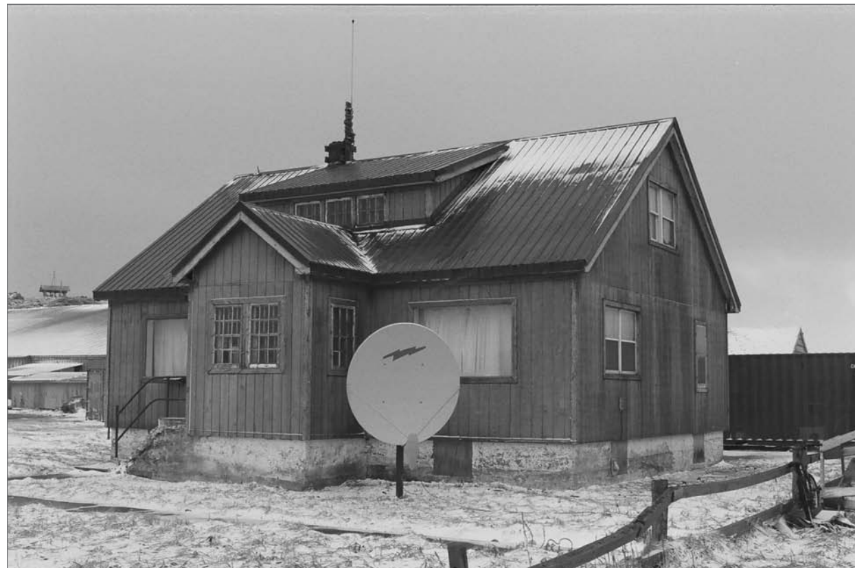
Mobley, Charles, photographer. 2007. South front and east side, House 112. Photograph (35mm) . NOAA, NOS, Pribilof Project Office, Seattle.
