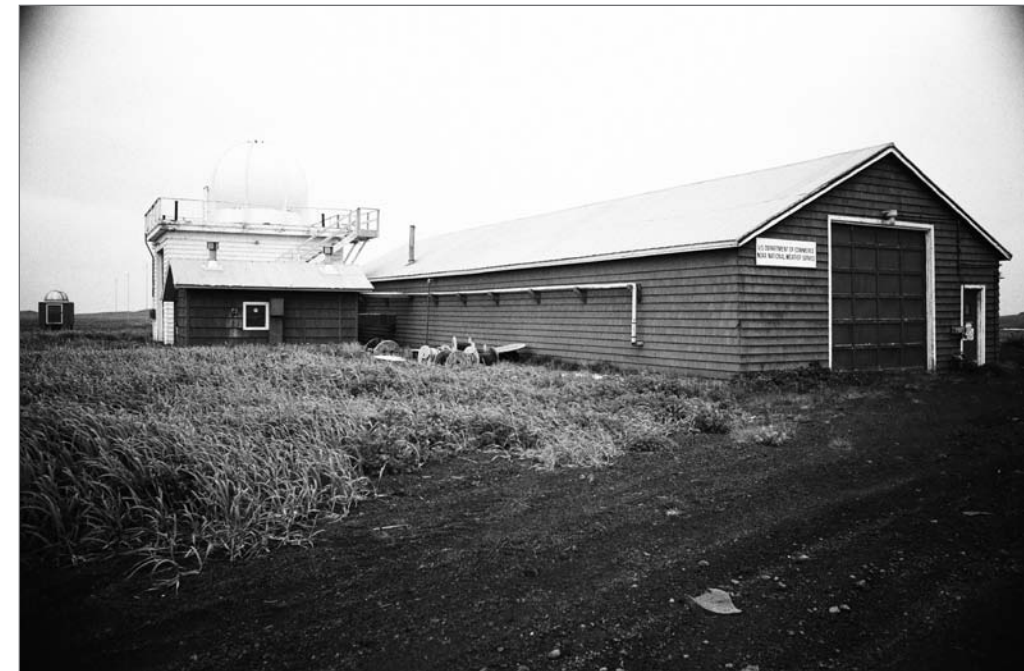
Photographer unknown. 1985. NOAA National Weather Service Station, garage and weather balloon launch area. Photograph. From Faulkner, 1986. Courtesy National Park Service, Anchorage, neg. file 01080007.
