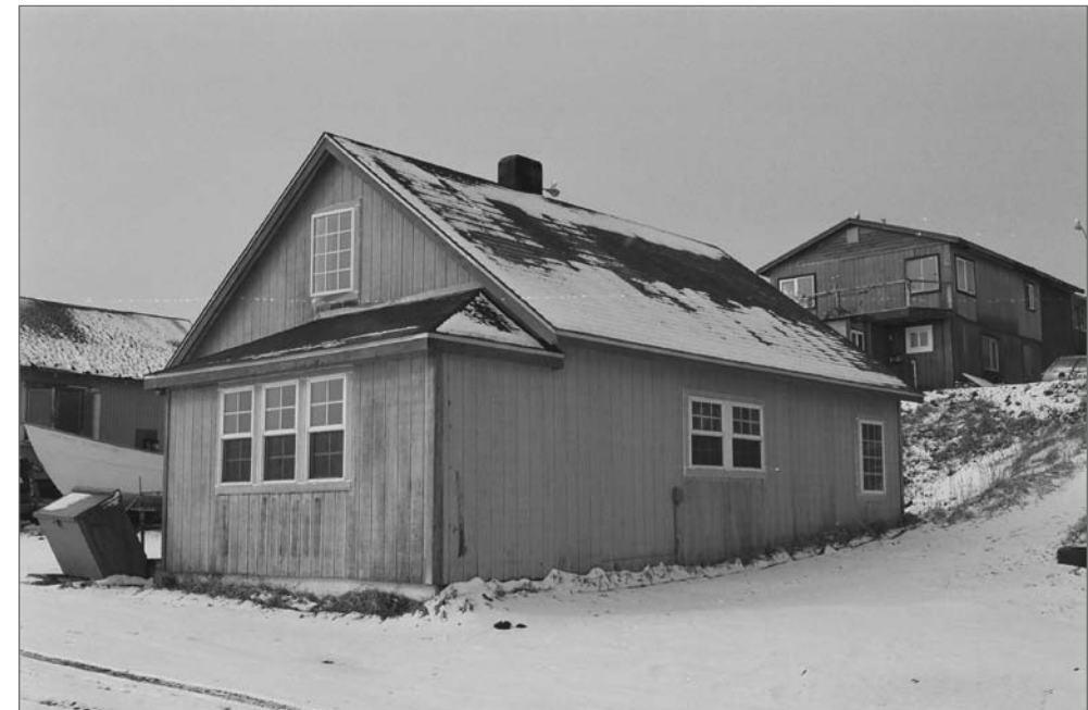
Mobley, Charles, photographer. 2007. East front and north side, Aleut Laborer House 3. Photograph (35mm) . NOAA, NOS, Pribilof Project Office, Seattle.
