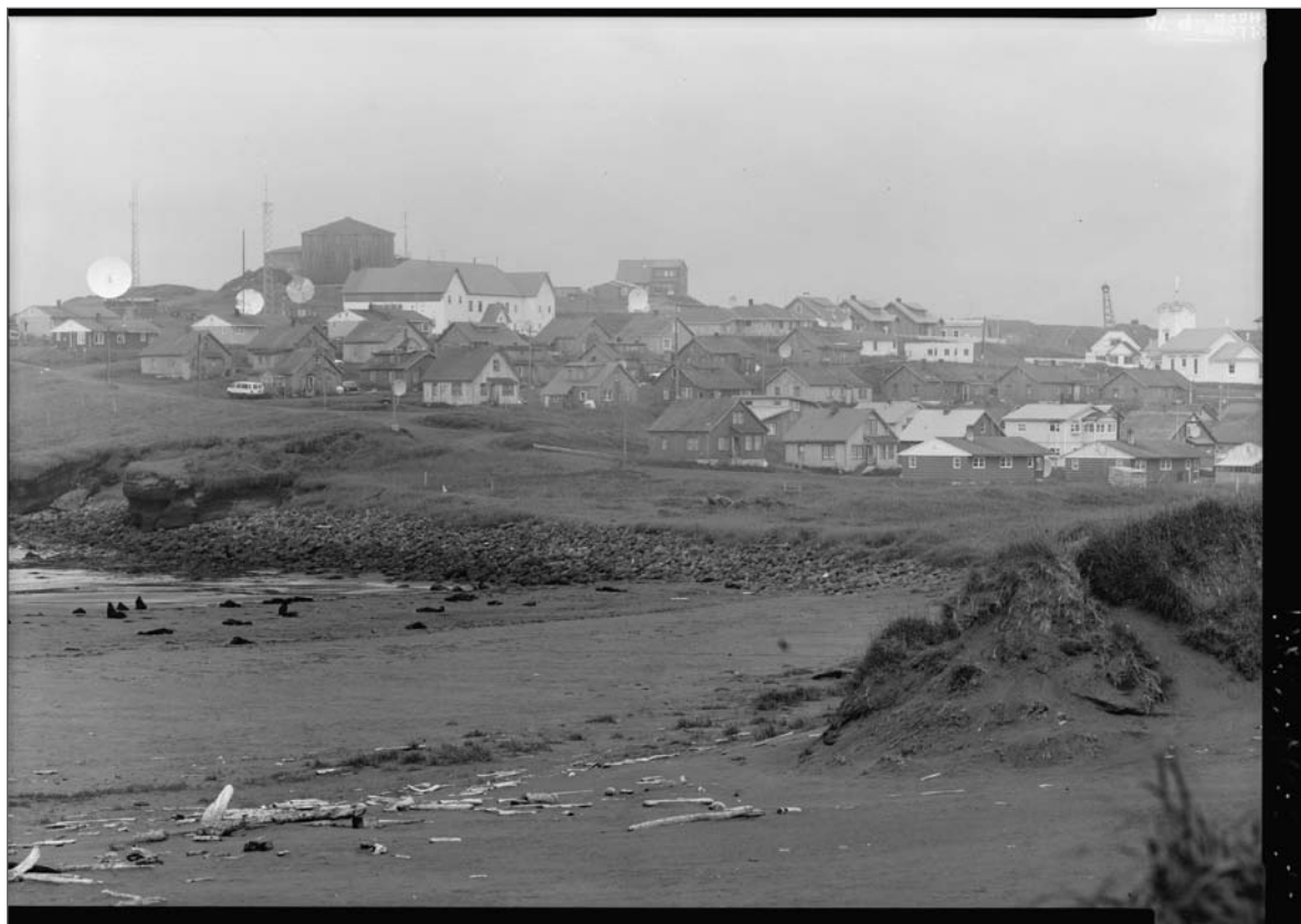
View of the City of St. Paul, looking from Zoltoi Sands. Jet Lowe, photographer. Photograph (5x7). Library of Congress: HABS AK-62-10 , 2004.
