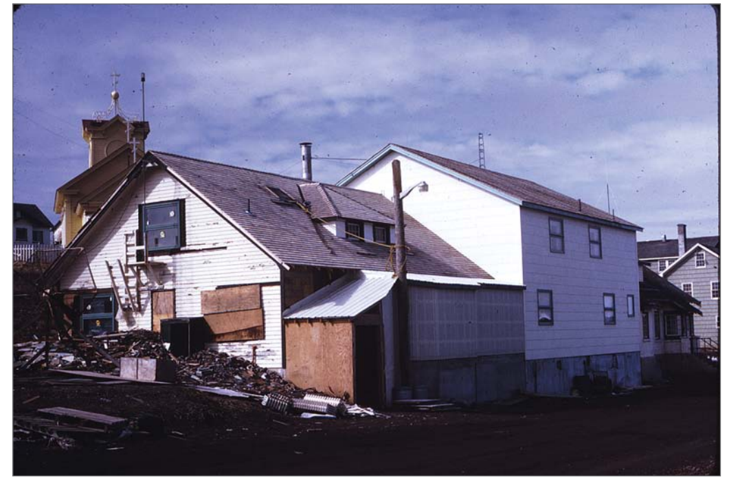
Fortune, Robert, photographer. April 1974. South and east sides, Hospital, showing 1974 center addition joining it to doctor's residence. Photograph (35mm). Courtesy Robert Fortune papers, Archives and Special Collections, Consortium Library, University of Alaska Anchorage. Collection number 7404aP6K05.
