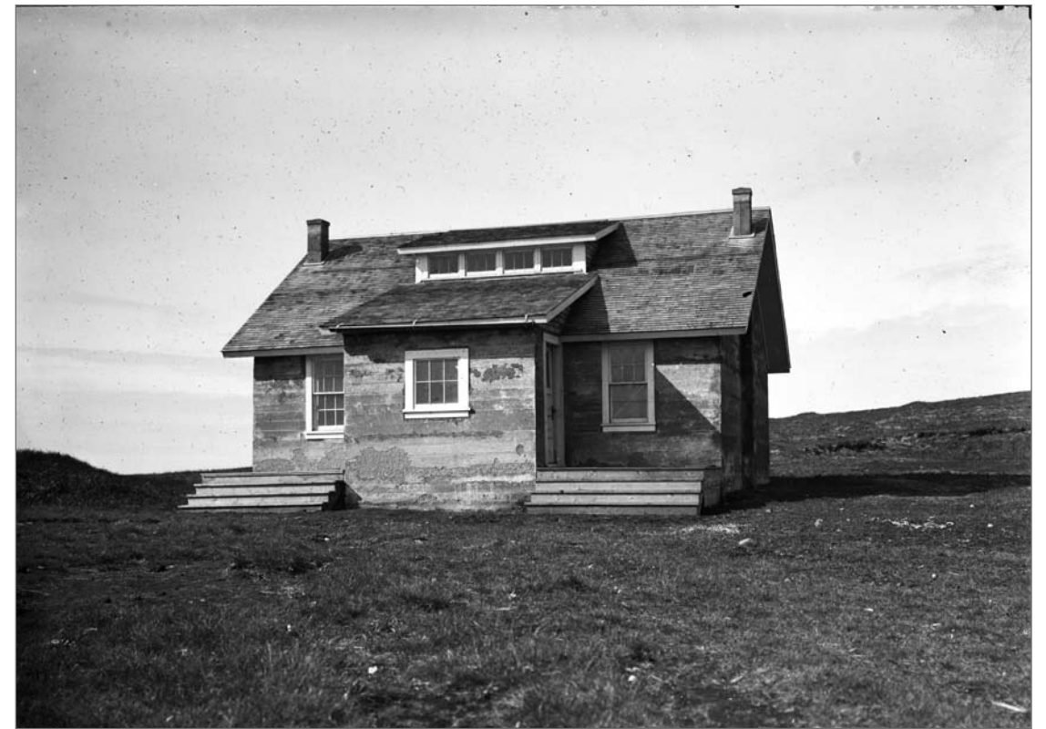
Photograph No. USBF 2.71 (Photographer unknown), 1920; Southeast front, concrete house. Records of the National Oceanic and Atmospheric Administration, RG 370; NARA—Pacific Alaska Region (A).
