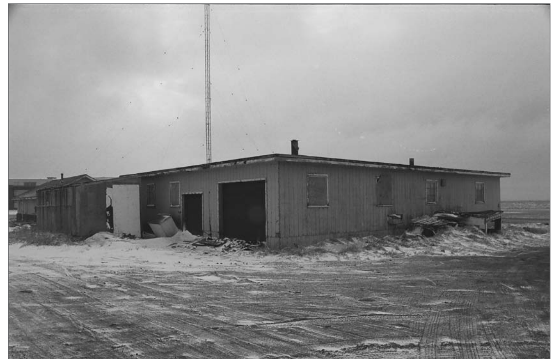
Mobley, Charles, photographer. 2007. West and north sides, Assembly of God Parsonage. Photograph (35mm). NOAA, NOS, Pribilof Project Office, Seattle.
