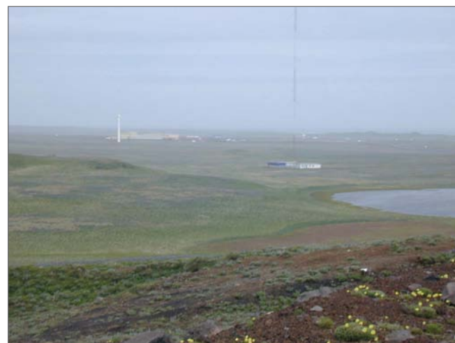
Photographer unknown. n.d. U.S. Coast Guard LORAN Station, St. Paul Island, AK. Photograph (digital). NOAA, NOS, Pribilof Project Office, Seattle.
