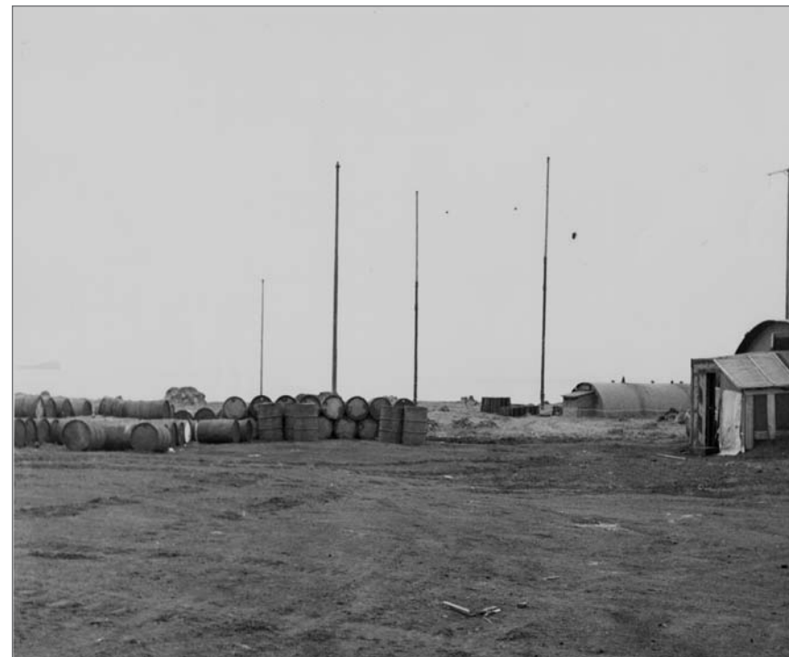
Photograph No. 95-ADMC-230 (Photographer unknown), August 5, 1948; Former Coast Guard LORAN Station at Southwest Point, showing fuel drums and Quonset huts. Records of the National Oceanic and Atmospheric Administration, RG 370; NARA—Pacific Alaska Region (A).
