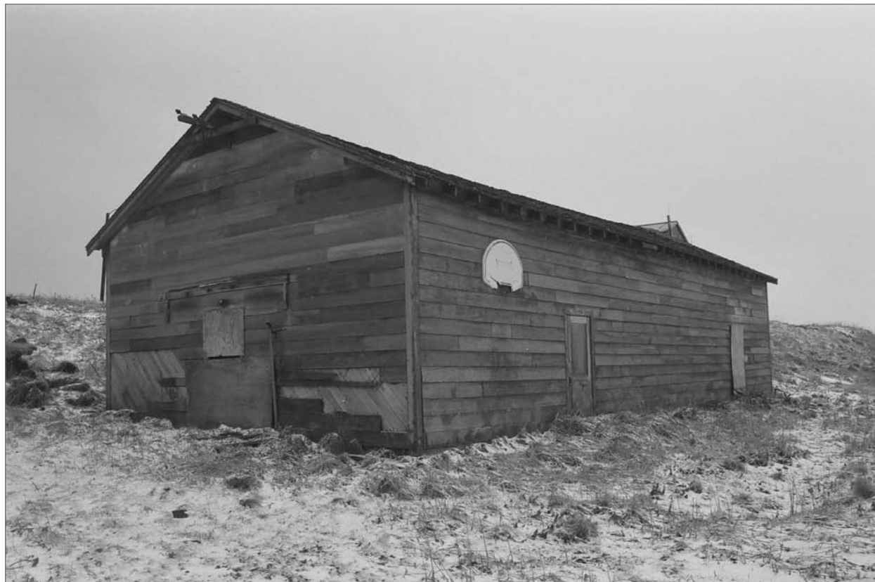
Mobley, Charles, photographer. 2007. Old Movie Theater, east and south sides. Photograph (35mm) . NOAA, NOS, Pribilof Project Office, Seattle.
