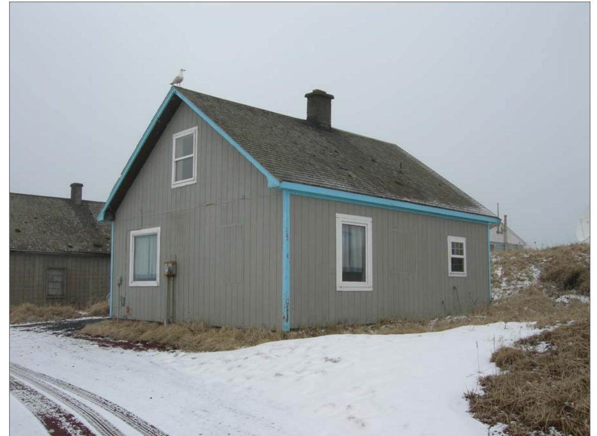
Mobley, Charles, photographer. 2007. East and north sides, Aleut Laborer House 25. Photograph (35mm). NOAA, NOS, Pribilof Project Office, Seattle.
