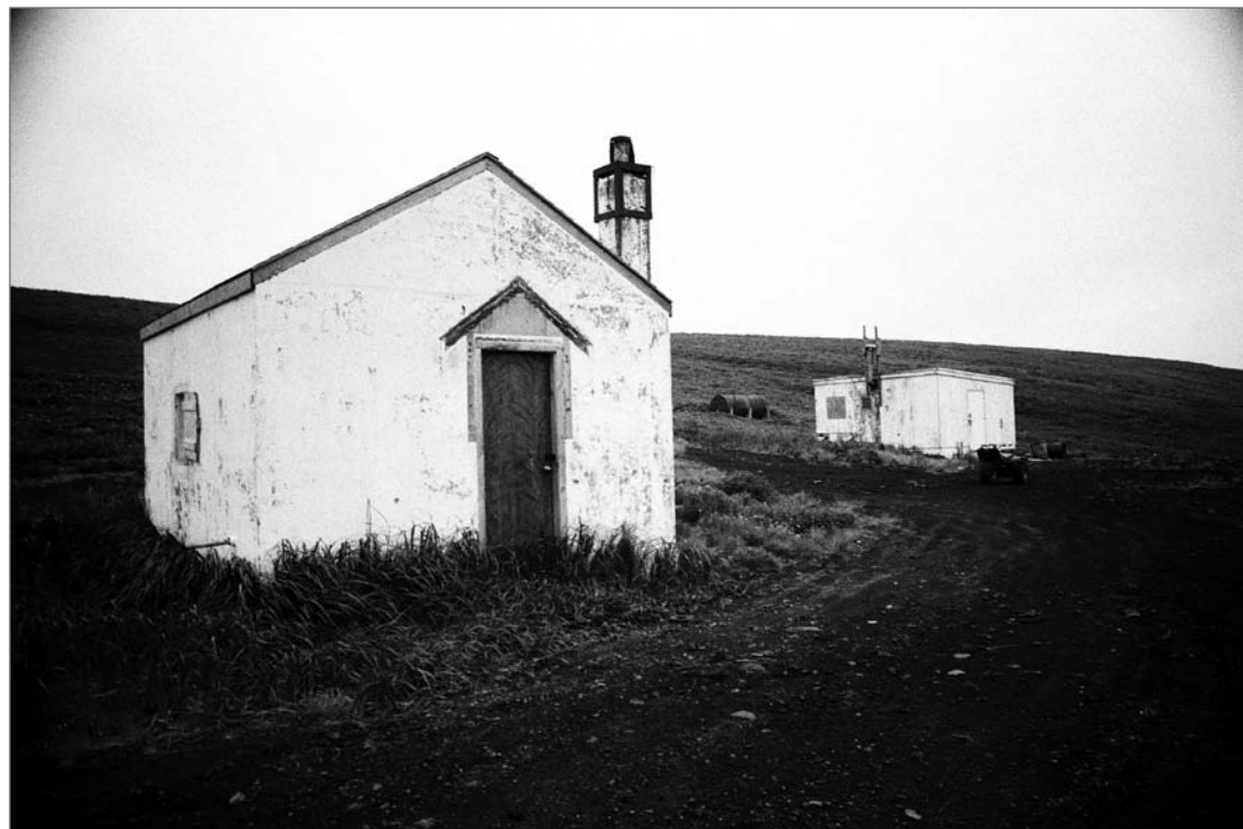
Photographer unknown. 1985. Pump House. Photograph. From Faulkner, 1986. Courtesy National Park Service, Anchorage, neg. file 10080008.
