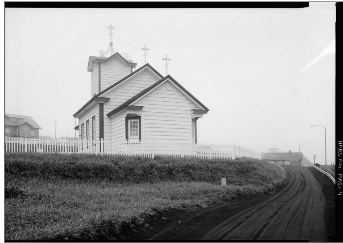
South and east sides, Church of the Holy Apostles Saints Peter and Paul. Jet Lowe, photographer. Photograph (5x7). Library of Congress: HABS AK-51-4 , 1989.
