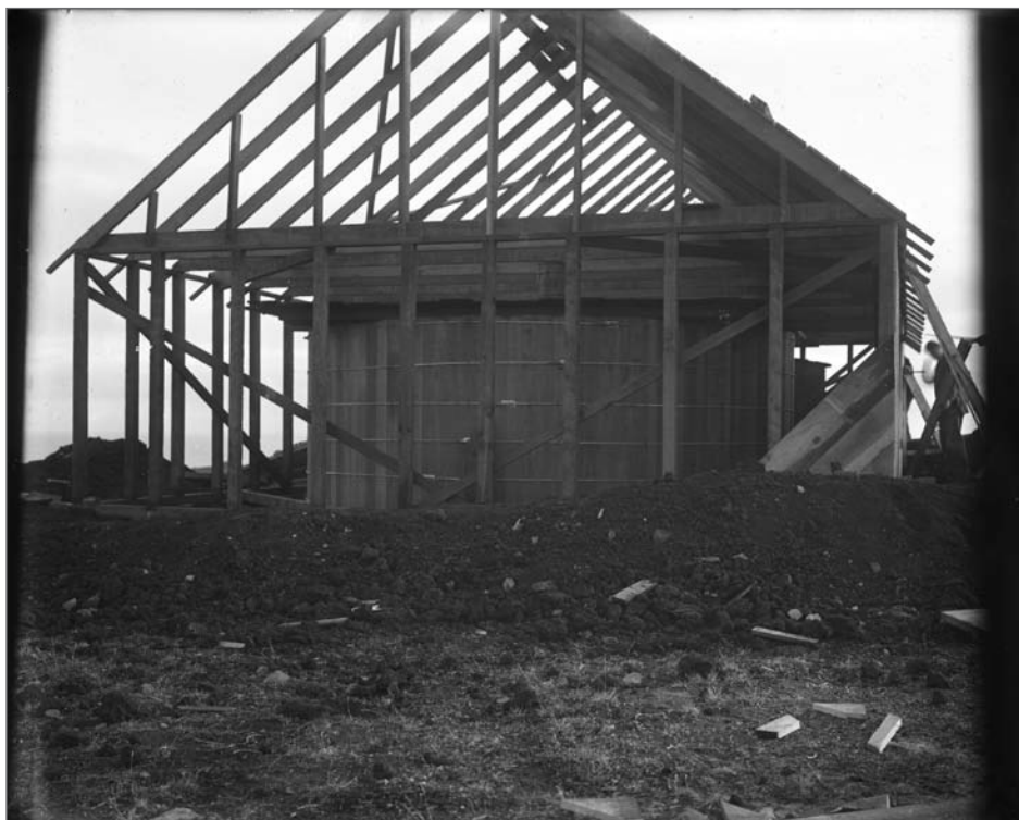
Photograph No. USBF 1.62 (Photographer unknown), 1912; Tank House under construction on Village Hill. 45 x 25 x 8 feet. The sides were made of 1 x 12 lumber laid diagonally and faced with two feet of sod. Freshwater was pumped from a well located about a half mile from the Naval Radio Station and stored in the tanks. Records of the National Oceanic and Atmospheric Administration, RG 370; NARA—Pacific Alaska Region (A).
