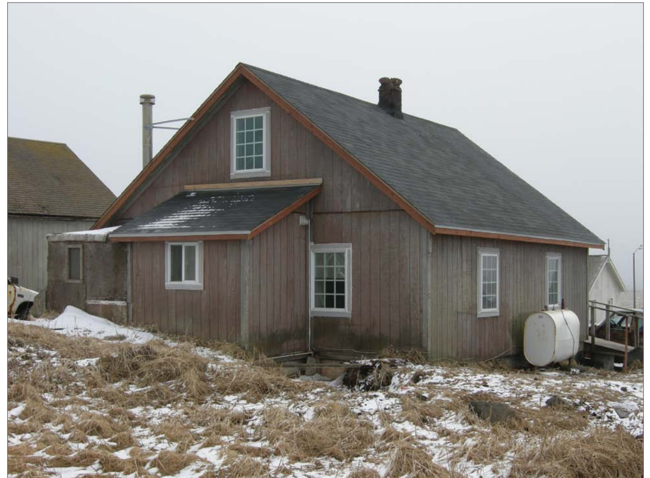
Mobley, Charles, photographer. 2007. West and south sides, Aleut Laborer House 29. Photograph (35mm). NOAA, NOS, Pribilof Project Office, Seattle.
