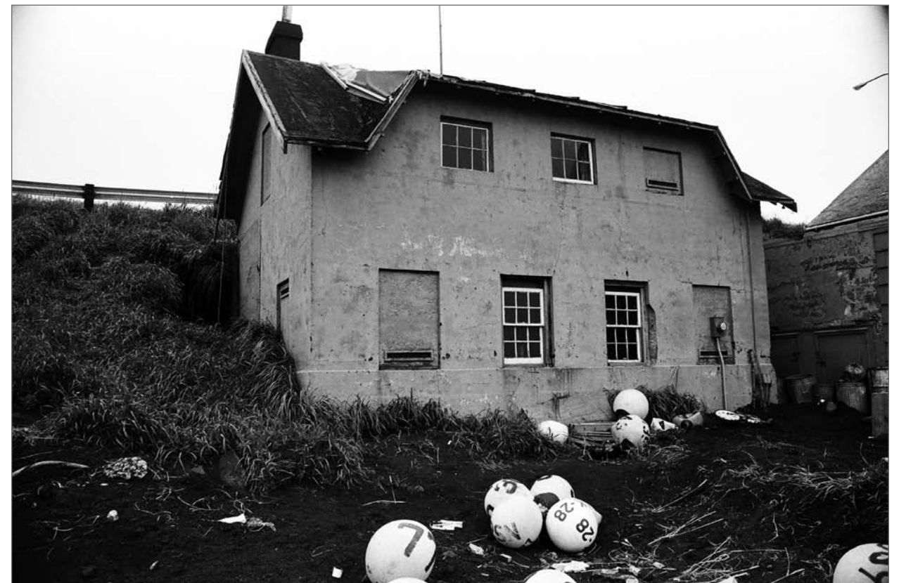
Brodherson, photographer. 1985. South and east sides, Laundry "Blck 18 Lot 3 concrete weird roofed." Photograph. From Faulkner, 1986. Courtesy National Park Service, Anchorage, neg. file 01090020.
