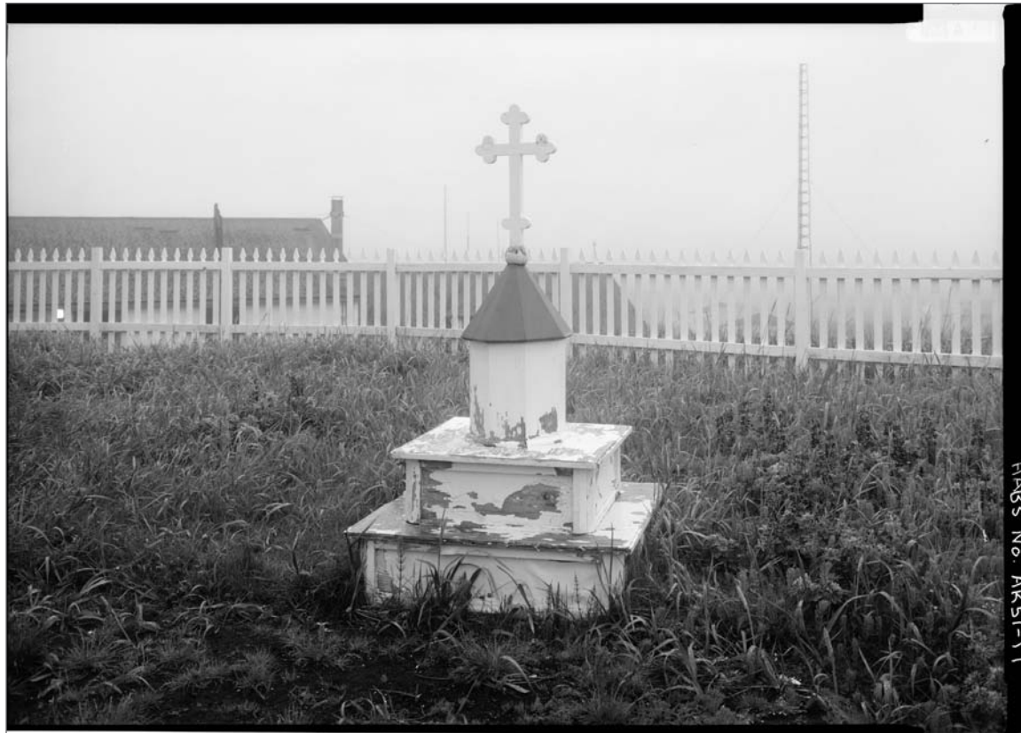
Shrine marking site of previous church [1875–1905], just south of present church, looking to east, 1989. Jet Lowe, photographer. Photograph (5x7). Library of Congress: HABS AK-51-17 , 1989.
