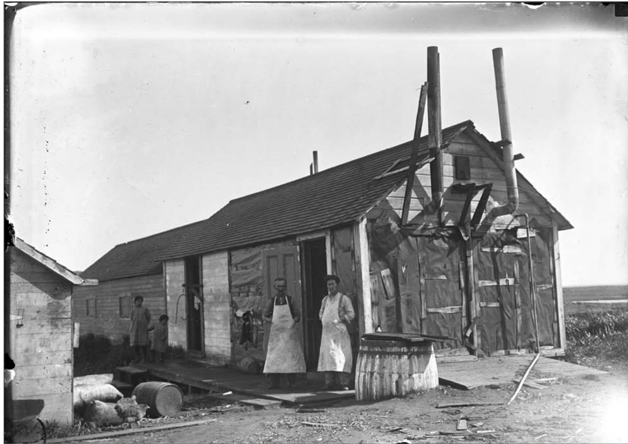
Photograph No. USBF 2.40 (Photographer Richard Culbertson), circa 1921; Former kitchen and mess for transient Unalaska laborers. The mess was created from the old bowling alley built in 1911 from a converted 30' x 12' x 8' boat house with a 40' x 12' x 6' extension. Two Miller Monitor #270 ranges were set up side by side for cooking, a temporary pipeline for saltwater was added, potable water was supplied in barrels. The Unalaska men slept in the Native Shop, which had been fitted with bunks. Records of the National Oceanic and Atmospheric Administration, RG 370; NARA—Pacific Alaska Region (A).
