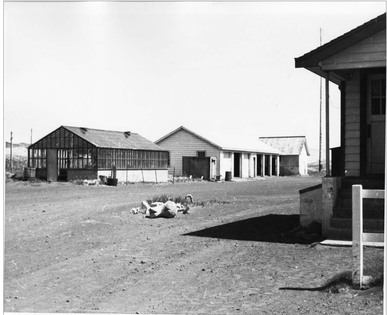
Photograph No. 95-ADMC-735 (Photographer unknown), n.d.; Greenhouse and garage on Sandy Lane, St. Paul Island, Alaska. Constructed in 1952 and visible in the 1966–67 Village of St. Paul air photo. Located to the left of the six-car garage and shingle shed. Records of the National Oceanic and Atmospheric Administration, RG 370; NARA—Pacific Alaska Region (A).
