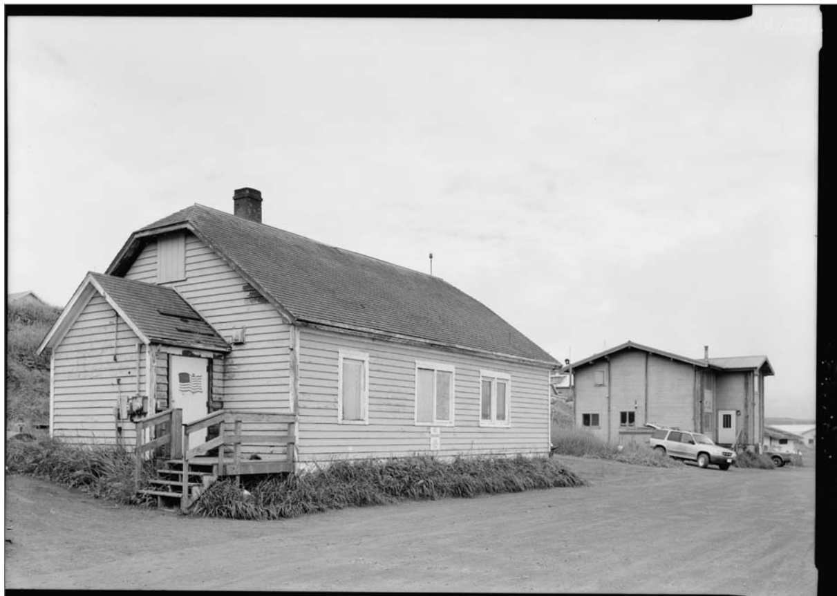
South front and east side, front view, Former Fisheries Office. Jet Lowe, photographer. Photograph (5x7). Library of Congress: HABS AK-211-1 , 2004.
