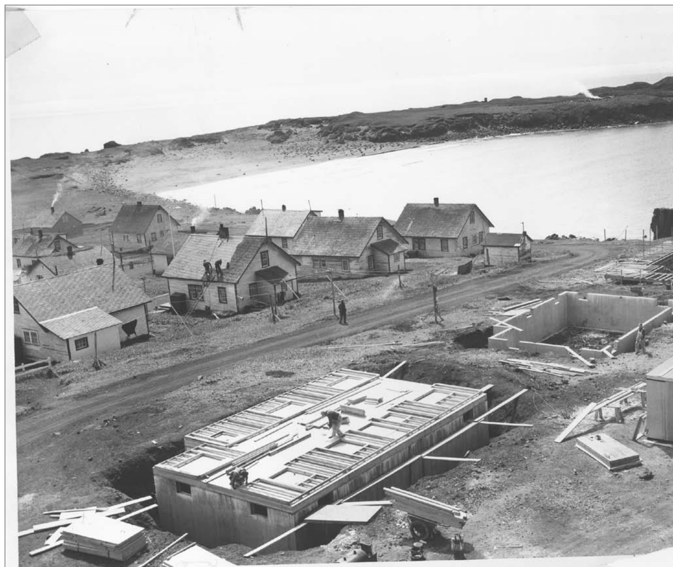
Photograph No. 95-ADMC-1989 (Photographer unknown), 1963; Ranch houses 117, 118, and 119 (left to right) under construction, with Gorbach in background. Records of the National Oceanic and Atmospheric Administration, RG 370; NARA—Pacific Alaska Region (A).
