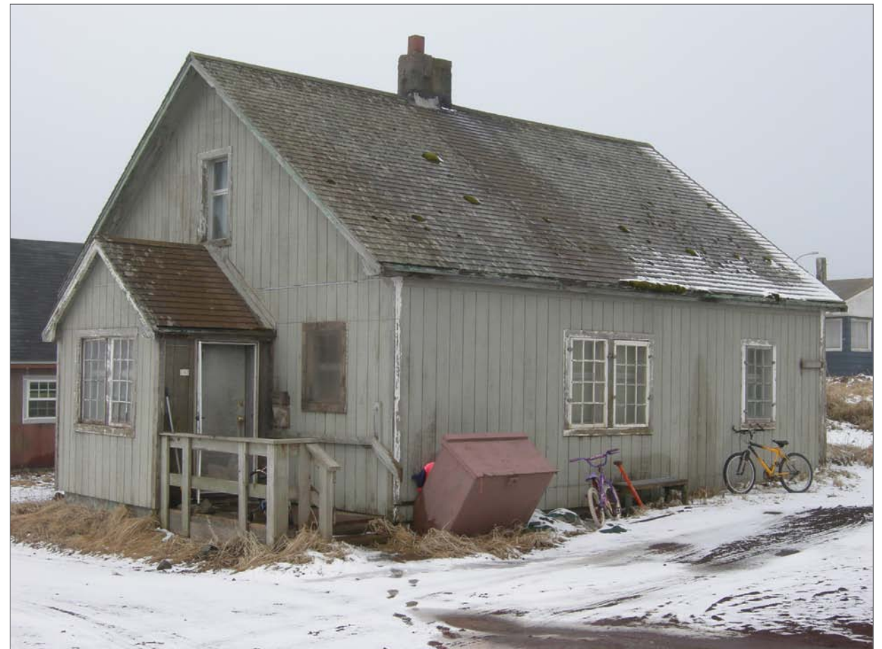
Mobley, Charles, photographer. 2007. East front and north side, Aleut Laborer House 28. Photograph (35mm). NOAA, NOS, Pribilof Project Office, Seattle.
