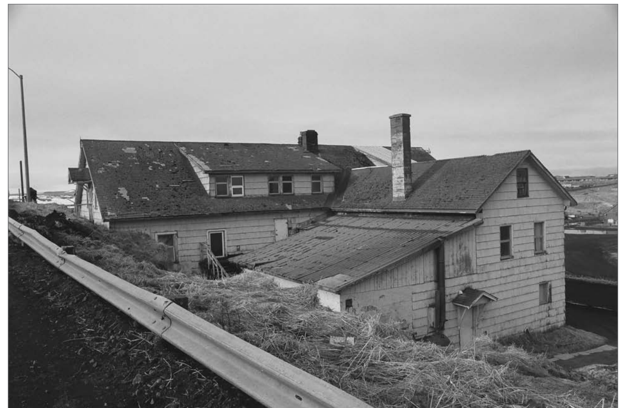
Mobley, Charles, photographer. 2007. West and south sides, King Eider Hotel, formerly called the Company House. Photograph (35mm). NOAA, NOS, Pribilof Project Office, Seattle.
