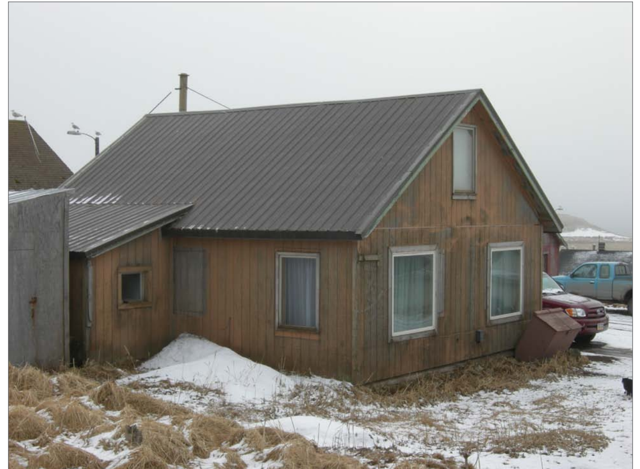
Mobley, Charles, photographer. 2007. West and south sides, Aleut Laborer House 27. Photograph (35mm). NOAA, NOS, Pribilof Project Office, Seattle.
