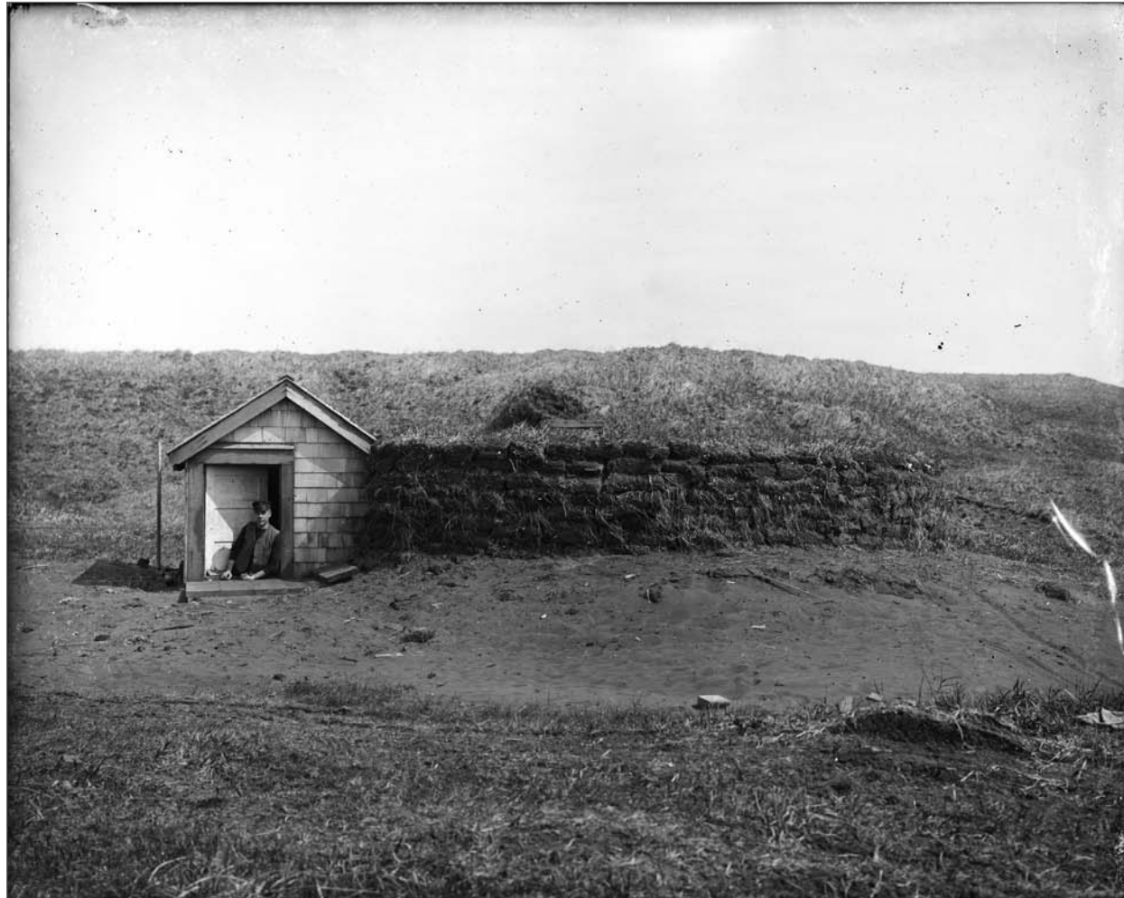
Photograph No. USBF 1.66 (Photographer unknown), 1912; Man standing in doorway of semi-subterranean structure, possibly a Pump House. In 1912, the U.S. Navy installed a pump at its Wireless Station and offered to pay for pipe to supply water to the Village. Native laborers dug a three-foot trench to carry the pipe a distance of 1480 feet from the Wireless Station to the Village flagstaff which was connected by pipes to two tanks on Village Hill. Small hydrant houses were strategically placed in the Village from which fresh water was obtained. Records of the National Oceanic and Atmospheric Administration, RG 370; NARA—Pacific Alaska Region (A).
