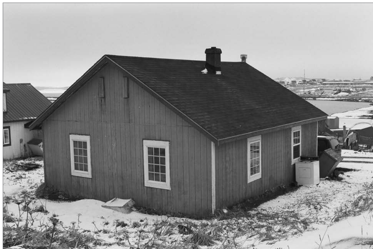
Mobley, Charles, photographer. 2007. West and south sides, Aleut Laborer House 16. Photograph (35mm). NOAA, NOS, Pribilof Project Office, Seattle.
