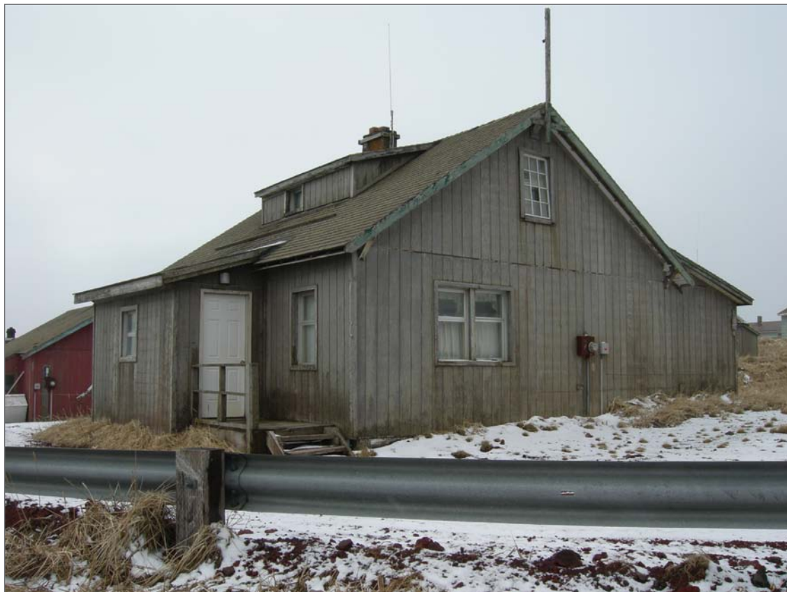
Mobley, Charles, photographer. 2007. East front and north side, Aleut Laborer House 31. Photograph (35mm). NOAA, NOS, Pribilof Project Office, Seattle.
