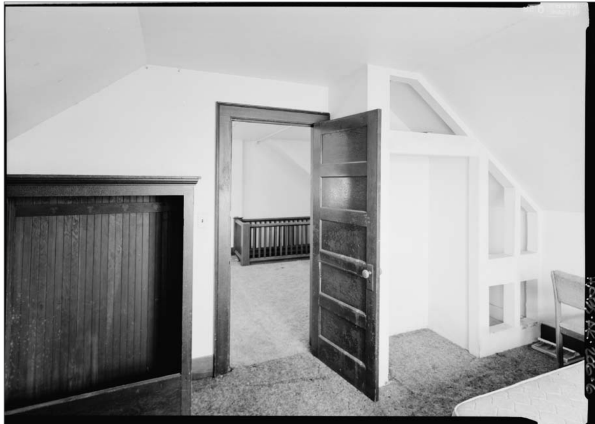
Interior, Teacher House 101, looking from north second-floor bedroom to center room, Teacher House 101, St. Paul Island, Alaska. Jet Lowe, photographer. Photograph (5x7). Library of Congress: HABS AK-206-6, 2004.
