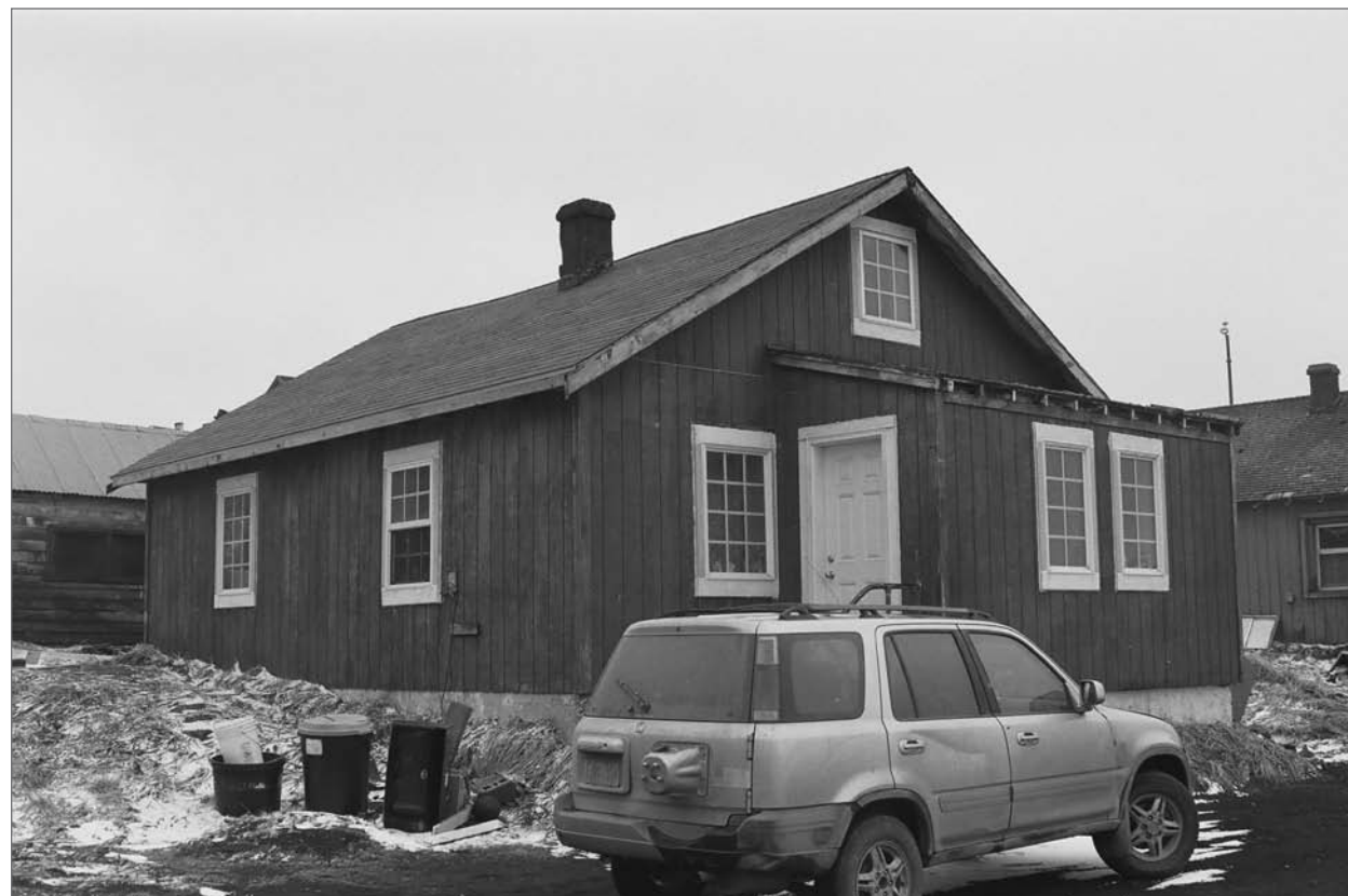
Mobley, Charles, photographer. 2007. South side and east front, Aleut Laborer House 45. Photograph (35mm) . NOAA, NOS, Pribilof Project Office, Seattle.
