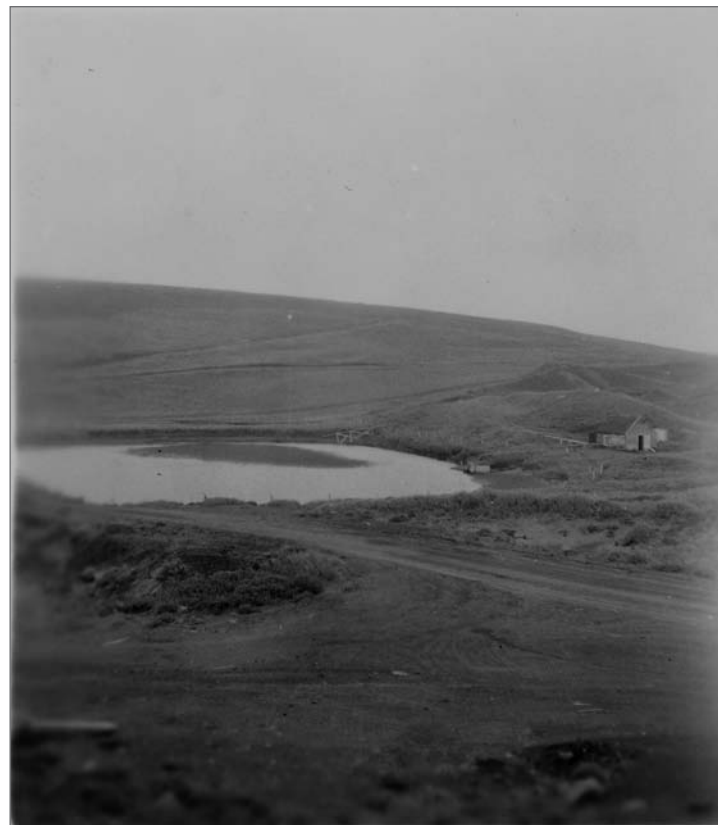
Photograph No. 95-ADMC-3086 (Photographer unknown), 1950; Pump House at Icehouse Lake. Records of the National Oceanic and Atmospheric Administration, RG 370; NARA—Pacific Alaska Region (A).
