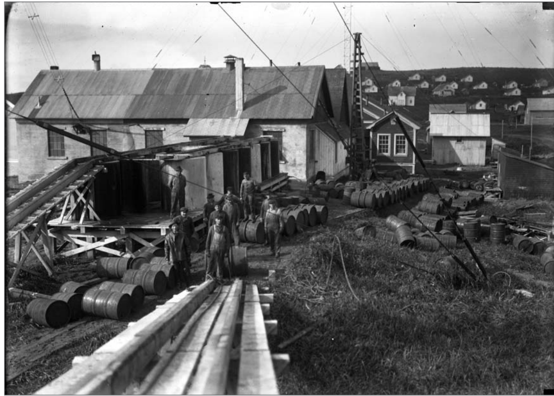
Photograph No. USBF 2.34 (Photographer unknown), 1920; East front and north side, Naval Radio Station Electrical Shop (E-shop), showing fuel storage tanks for supplying the generators. Records of the National Oceanic and Atmospheric Administration, RG 370; NARA—Pacific Alaska Region (A).
