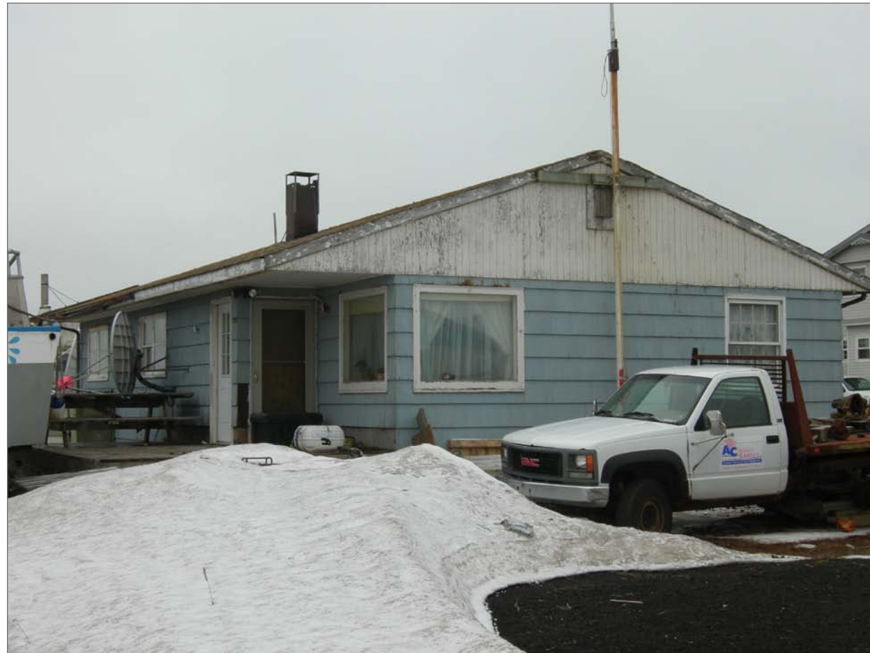
Mobley, Charles, photographer. 2007. East front and north side, Aleut Laborer House 125. Photograph (35mm). NOAA, NOS, Pribilof Project Office, Seattle.
