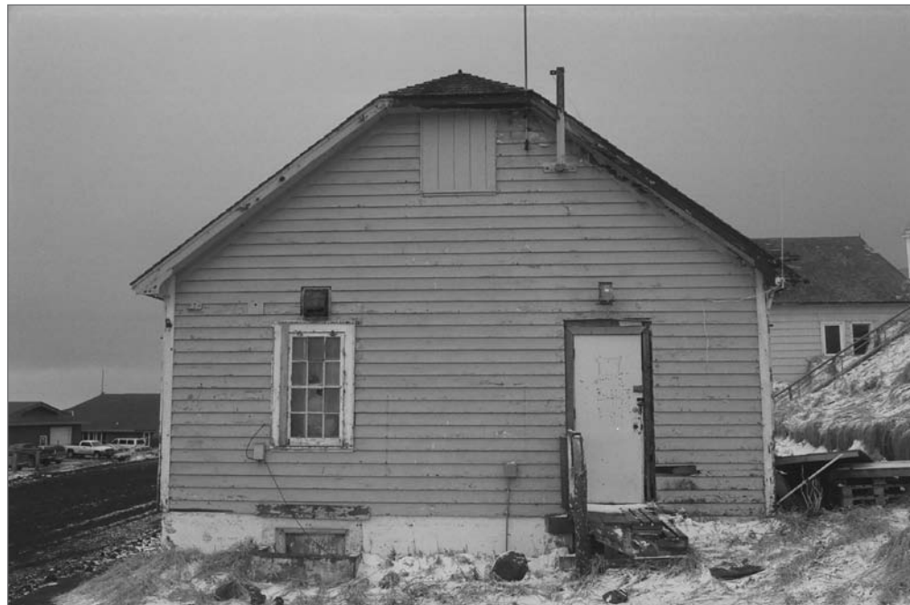
Mobley, Charles, photographer. 2007. North side, Former Fisheries Office. Photograph (35mm) . NOAA, NOS, Pribilof Project Office, Seattle.
