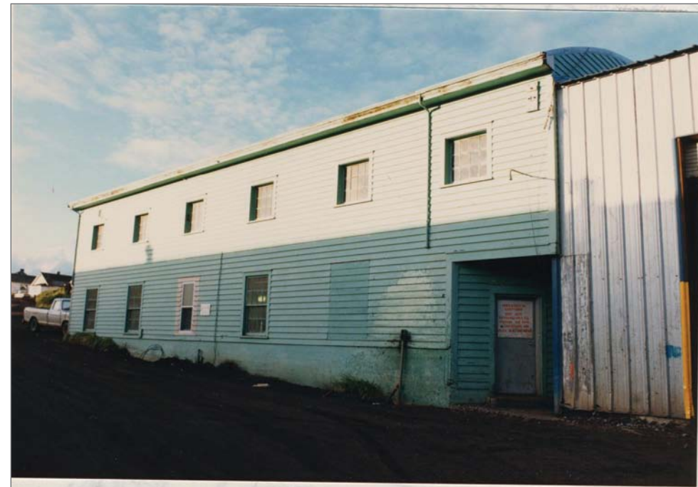
View northwesterly of north elevation adjoining new addition
