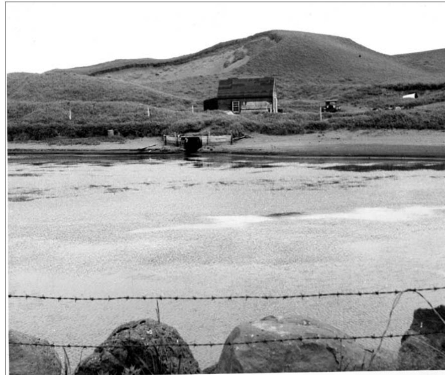
Photograph No. 95-ADMC-257 (Photographer unknown), 1948; Icehouse Lake water reservoir and Pump House. The St. Paul Village obtained its municipal water supply from four wells located about 1.5 miles north-east of the city and immediately east of Telegraph Hill (Fredreka I, Fredreka II, south well, and north well). A fifth well served the USCG LORAN station. The four municipal wells were connected by pipelines that supplied three 200,000-gallon water storage tanks located on Village Hill above the city, August 6, 1948. Records of the National Oceanic and Atmospheric Administration, RG 370; NARA—Pacific Alaska Region (A).
