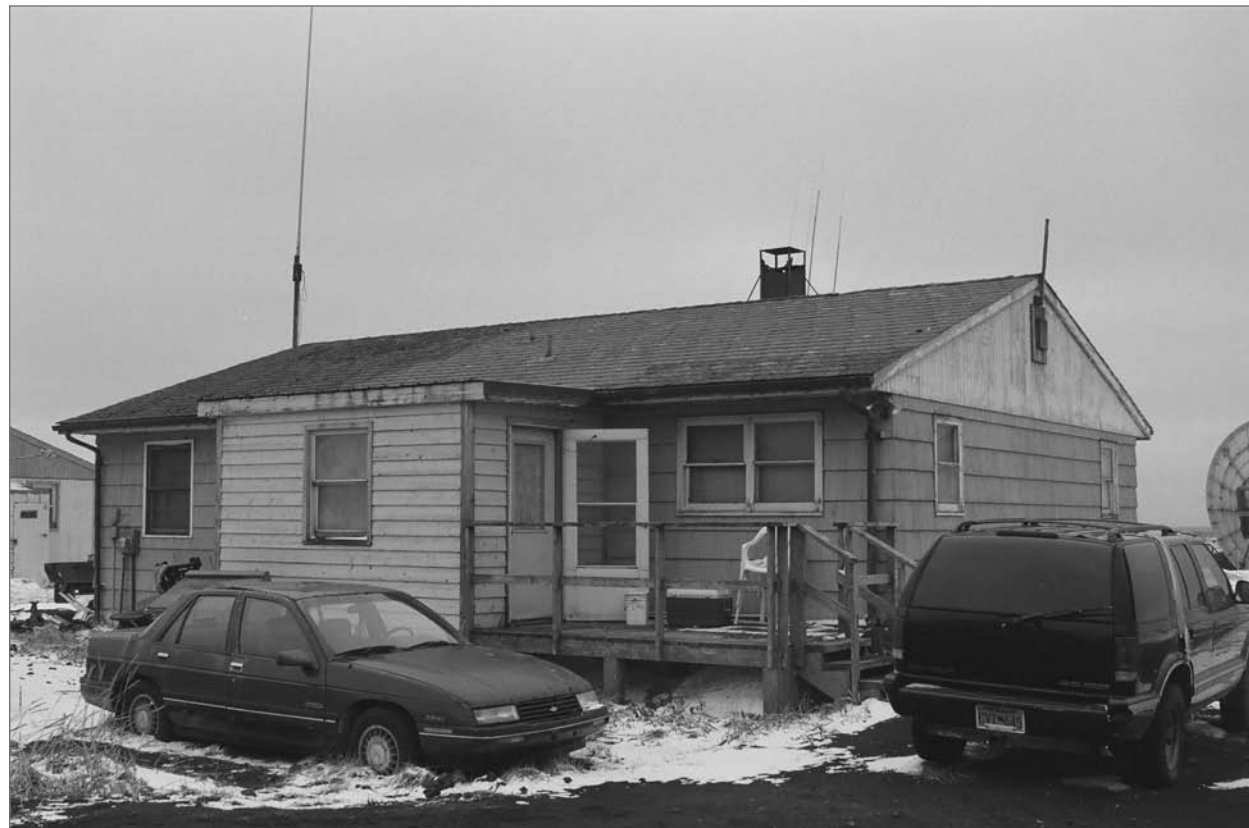
Mobley, Charles, photographer. 2007. West and south sides, Aleut Laborer House 125. Photograph (35mm).
