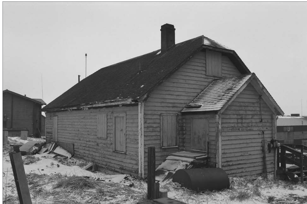
Mobley, Charles, photographer. 2007. West and south sides, Former Fisheries Office. Photograph (35mm) . NOAA, NOS, Pribilof Project Office, Seattle.
