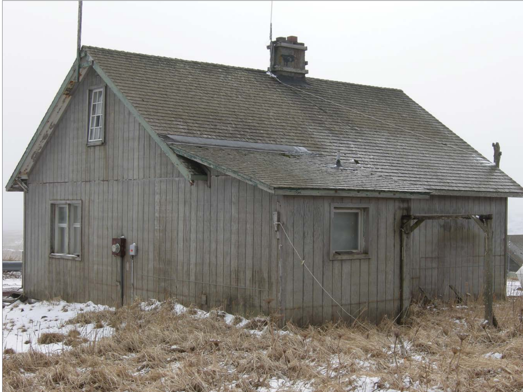
Mobley, Charles, photographer. 2007. North and west sides, Aleut Laborer House 31. Photograph (35mm) . NOAA, NOS, Pribilof Project Office, Seattle.
