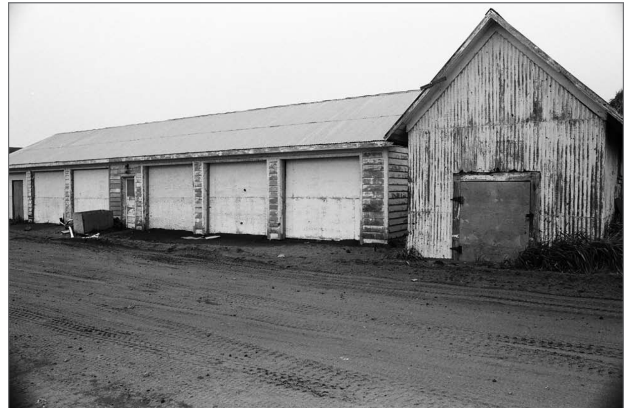
Photographer unknown. 1985. South front, Six-Car Garage, Shingle Shed (right). Photograph . From Faulkner, 1986. Courtesy National Park Service, Anchorage, neg. file 01110004.
