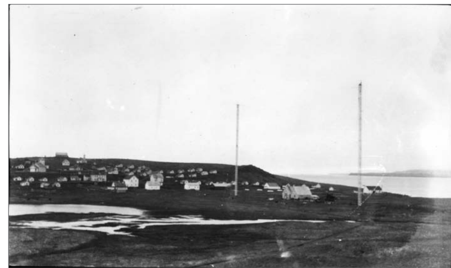
Photographer unknown. Circa 1913. Naval Radio Station, looking west northwest. The gravel used in the concrete anchors for the masts was scratched from between the rocks at East Landing and carried 100 yards on men's backs to wagons for transport to the station. Photograph. Pribilof Islands Photographs Collection, no. 1976-0063-00208, Archives, Alaska and Polar Regions Collections, Rasmuson Library, University of Alaska Fairbanks.
