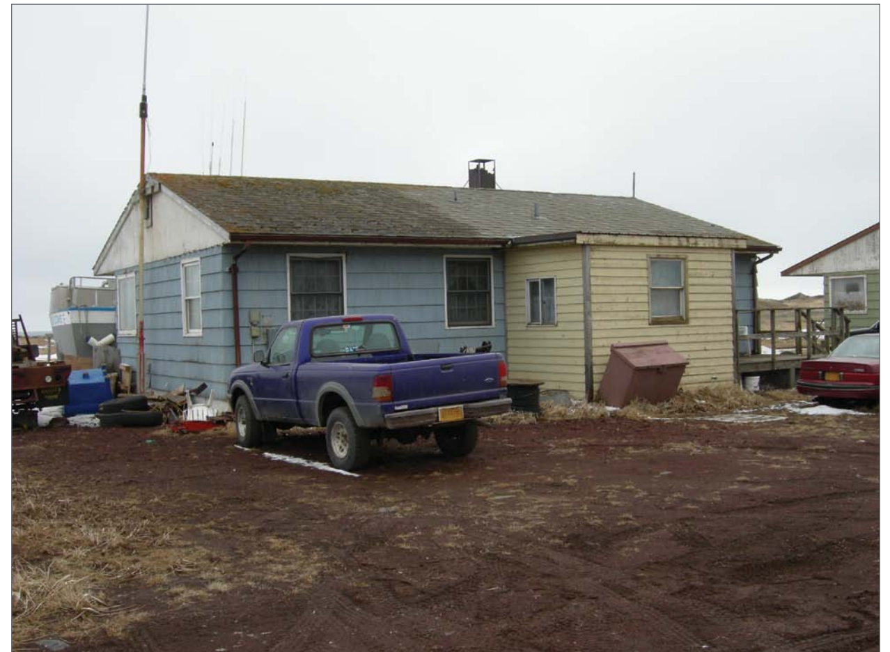
Mobley, Charles, photographer. 2007. North and west sides, Aleut Laborer House 125. Photograph (35mm). NOAA, NOS, Pribilof Project Office, Seattle.
