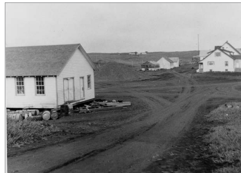
Photograph No. 95-ADMC-2514 (Photographer unknown), circa 1985; Former Paint Shop (left foreground) and Navy Radio Station. Records of the National Oceanic and Atmospheric Administration, RG 370; NARA—Pacific Alaska Region (A).
