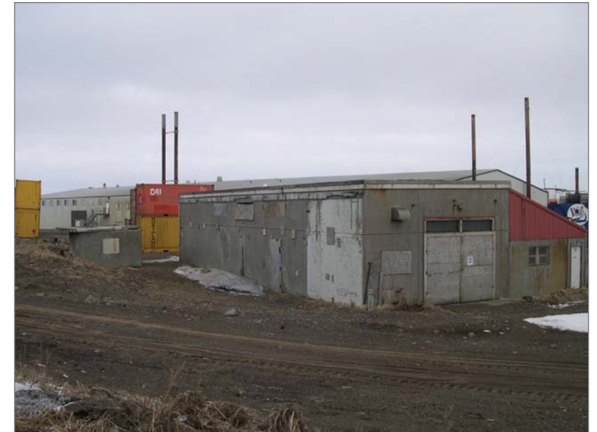
Winandy, David B., photographer. 2006. East and south sides, former Power Plant showing Saltwater Well House 3 (left). Saltwater was used for cooling in the Power Plant, March 3, 2006. Photograph (digital). NOAA, NOS, Pribilof Project Office, Seattle.
