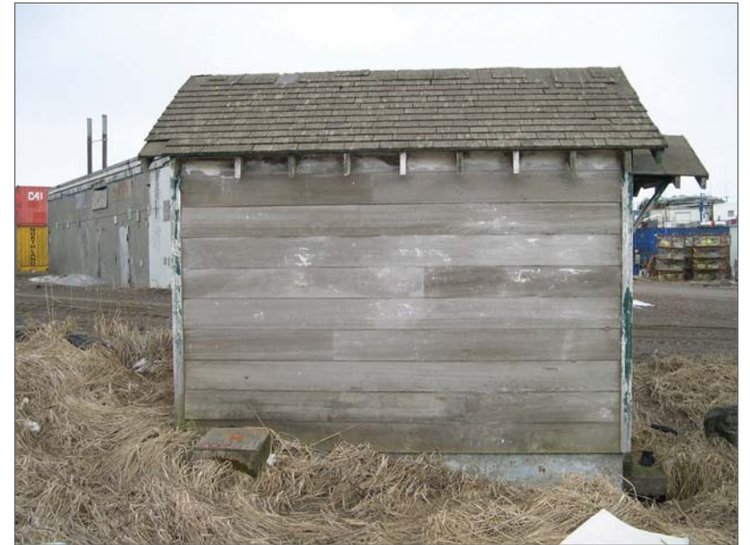
Winandy, David, photographer. 2006. Saltwater Well House 2, March 21, 2006. Photograph (digital). NOAA, NOS, Pribilof Project Office, Seattle.
