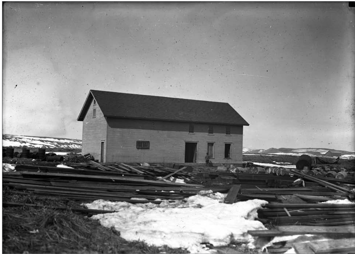
Photograph No. USBF 2.46 (Photographer G Dallas Hanna), May 1919; Former Cold Storage Building, erected 1912. This building has been used for multiple purposes. It was converted to a Machine Shop in 1918, to a Boat House by 1940, to a Plumbing Shop by 1959, and to the Community Garage/Village Automotive Repair Shop in 1966. It was demolished between 1986–1993. Records of the National Oceanic and Atmospheric Administration, RG 370; NARA—Pacific Alaska Region (A).
