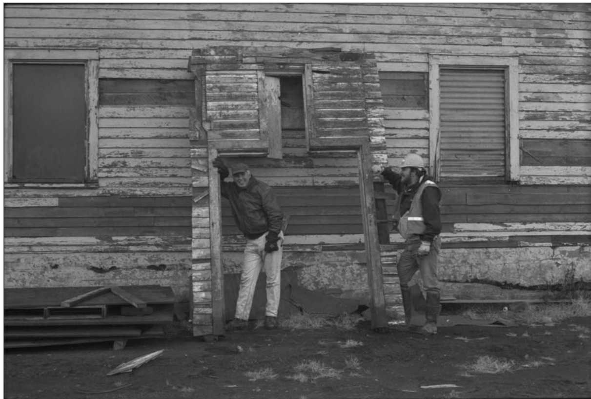
Young, Allison, photographer. 2000. Salthouse A, south end, Key-Hole door frame removed for archiving. John Lindsay (left). Photograph (35mm). NOAA, NOS, Pribilof Project Office, Seattle: sheet JL 110929.1, neg. 4251.
