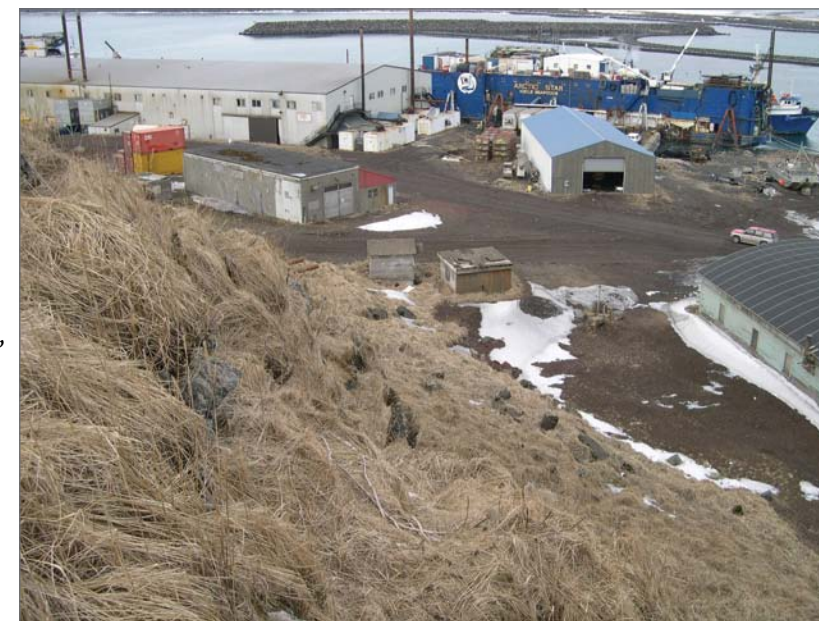
Winandy, David B., photographer. March 21, 2006. Receiving Warehouse (center), Power Plant (left), Machine Shop (right), Trident Seafoods (left background), and Equipment Garage (right foreground). Photograph (digital). NOAA, NOS, Pribilof Project Office, Seattle.
