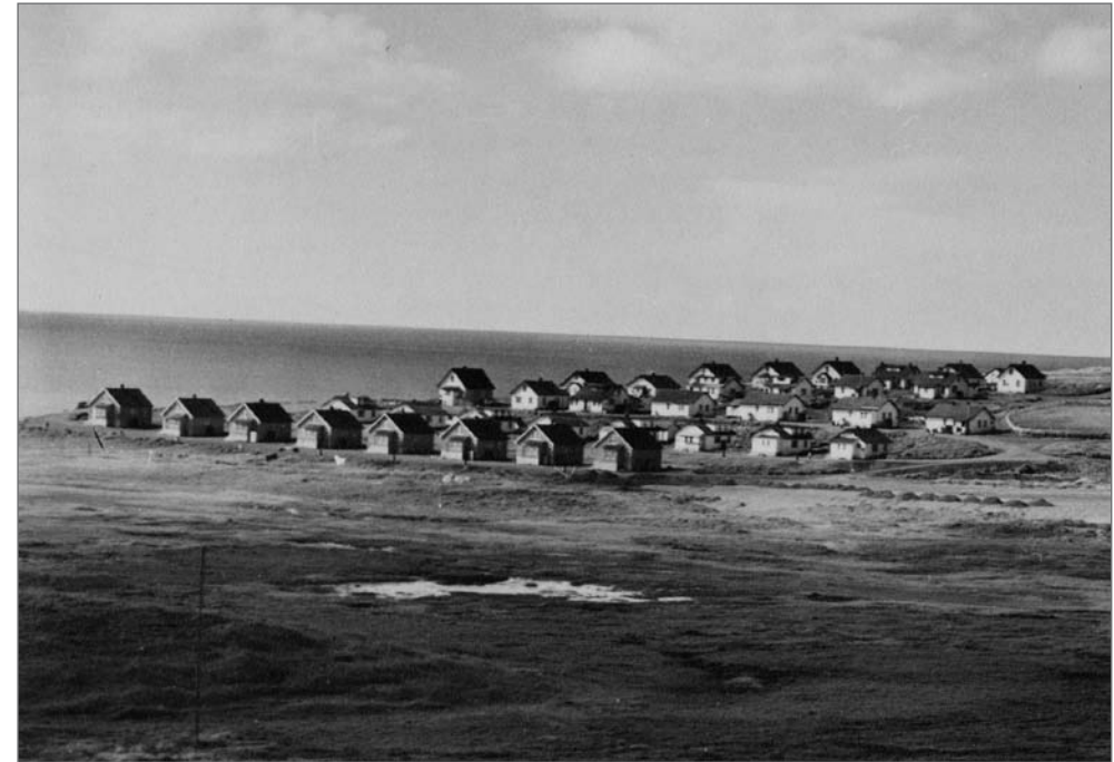
Haddon, Emmett P., photographer. 1949. This photograph shows the housing layout on the south side of St. Paul Village in 1952, looking west southwest, September 21, 1949. The front row of houses (houses 52–59) are Type V houses prior to any significant alterations. Photograph. NOAA, NMML Library, Seattle: Photograph. NOAA, NMML Library, Seattle: Fur-Seal Archives, no file no.
