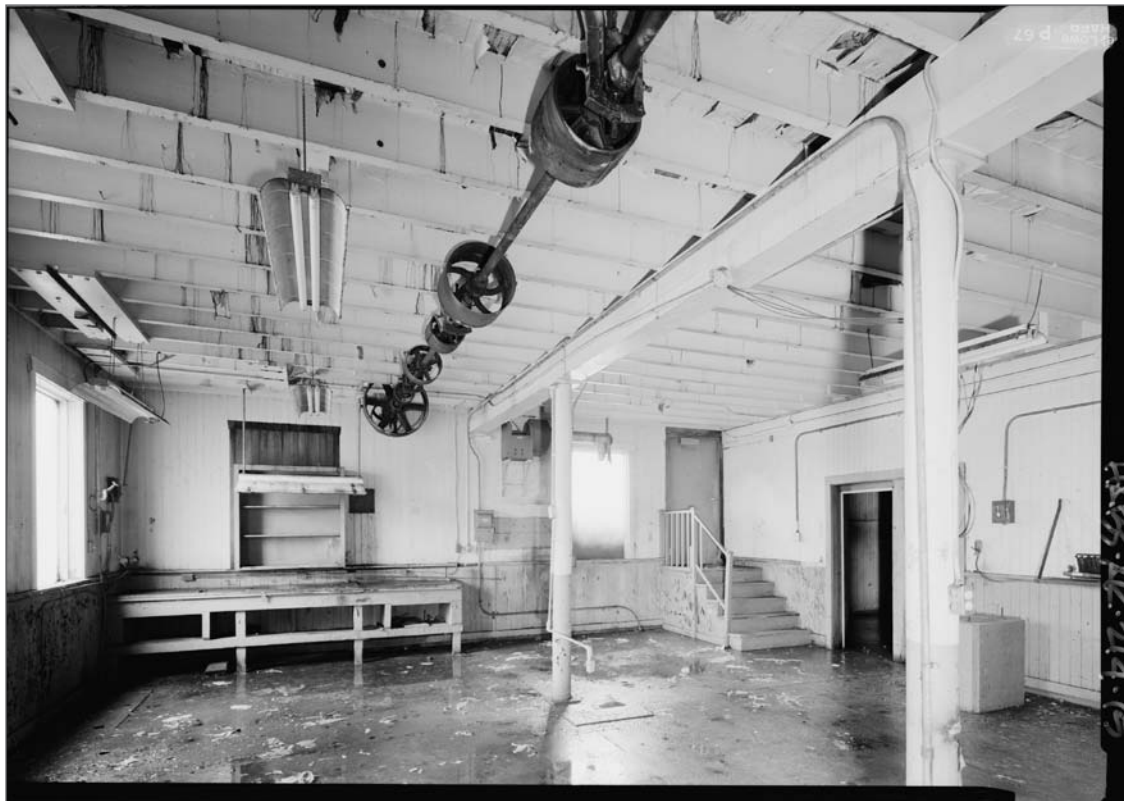
Interior, Machine Shop, looking south, showing line shaft. Jet Lowe, photographer. Photograph (5x7). Library of Congress: HABS AK-214-15 , 2004.
