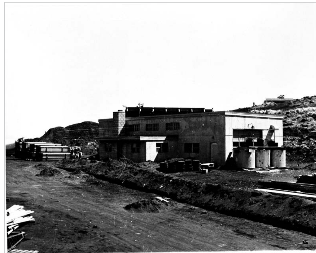
Photograph No. 95-ADMC-931 (Photographer unknown), n.d.; West and north sides, former Power Plant. Records of the National Oceanic and Atmospheric Administration, RG 370; NARA—Pacific Alaska Region (A) .
