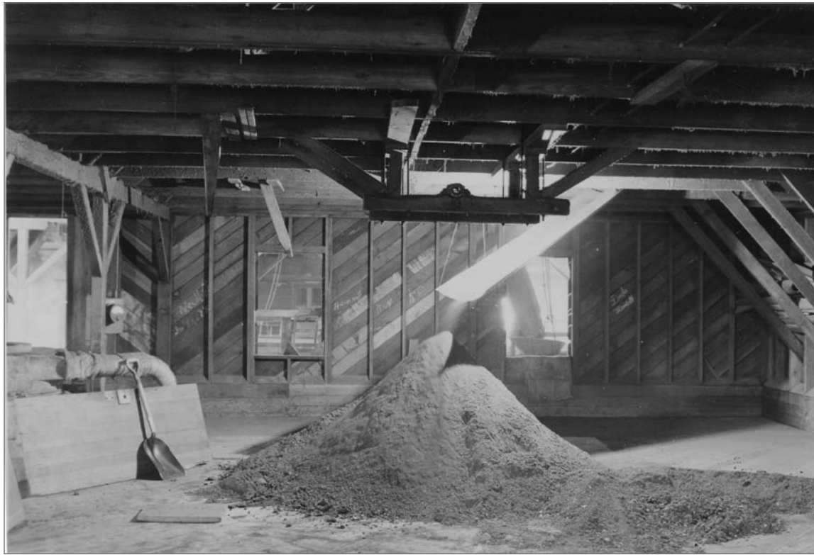
Scheffer, Victor B., photographer. 1947. "By-products plant, St. Paul Island, Alaska, 24 July 1947. Loft, with seal meal piling up. At intervals it is pushed through a hole in the floor to the hammer mill." Photograph. NOAA, NMML Library, Seattle: Victor B. Scheffer Collection, Fur-Seal Archives, neg. no. 2236.
