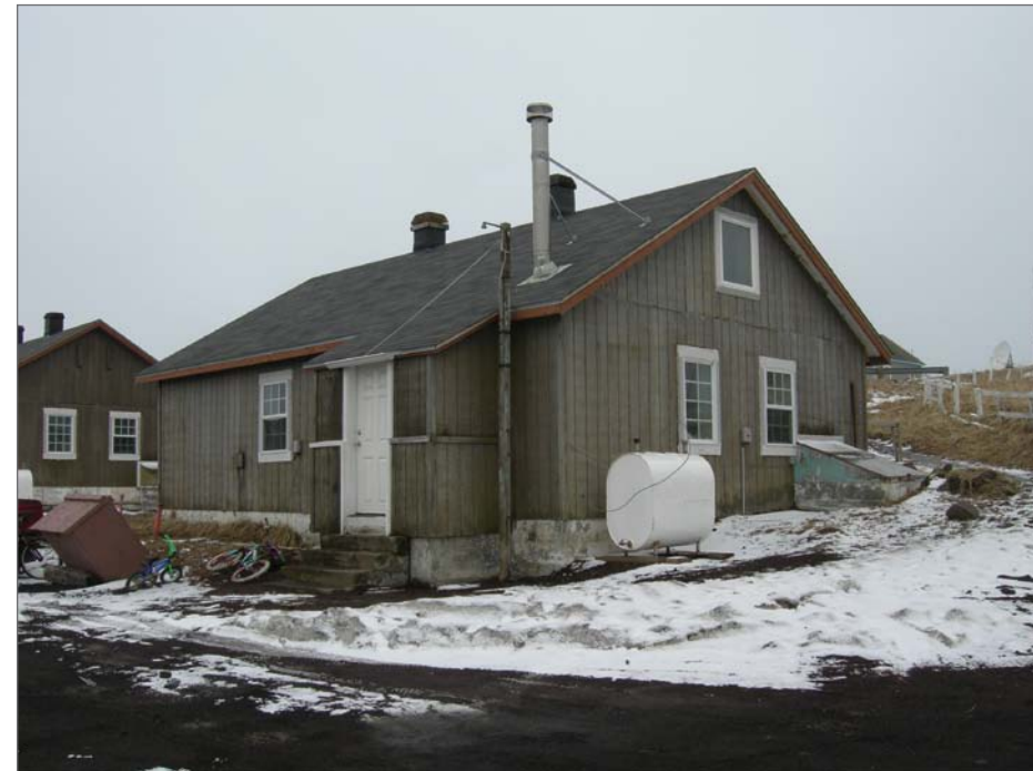
Mobley, Charles, photographer. 2007. East front and north side, Aleut Laborer House 37. Photograph (35mm). NOAA, NOS, Pribilof Project Office, Seattle.
