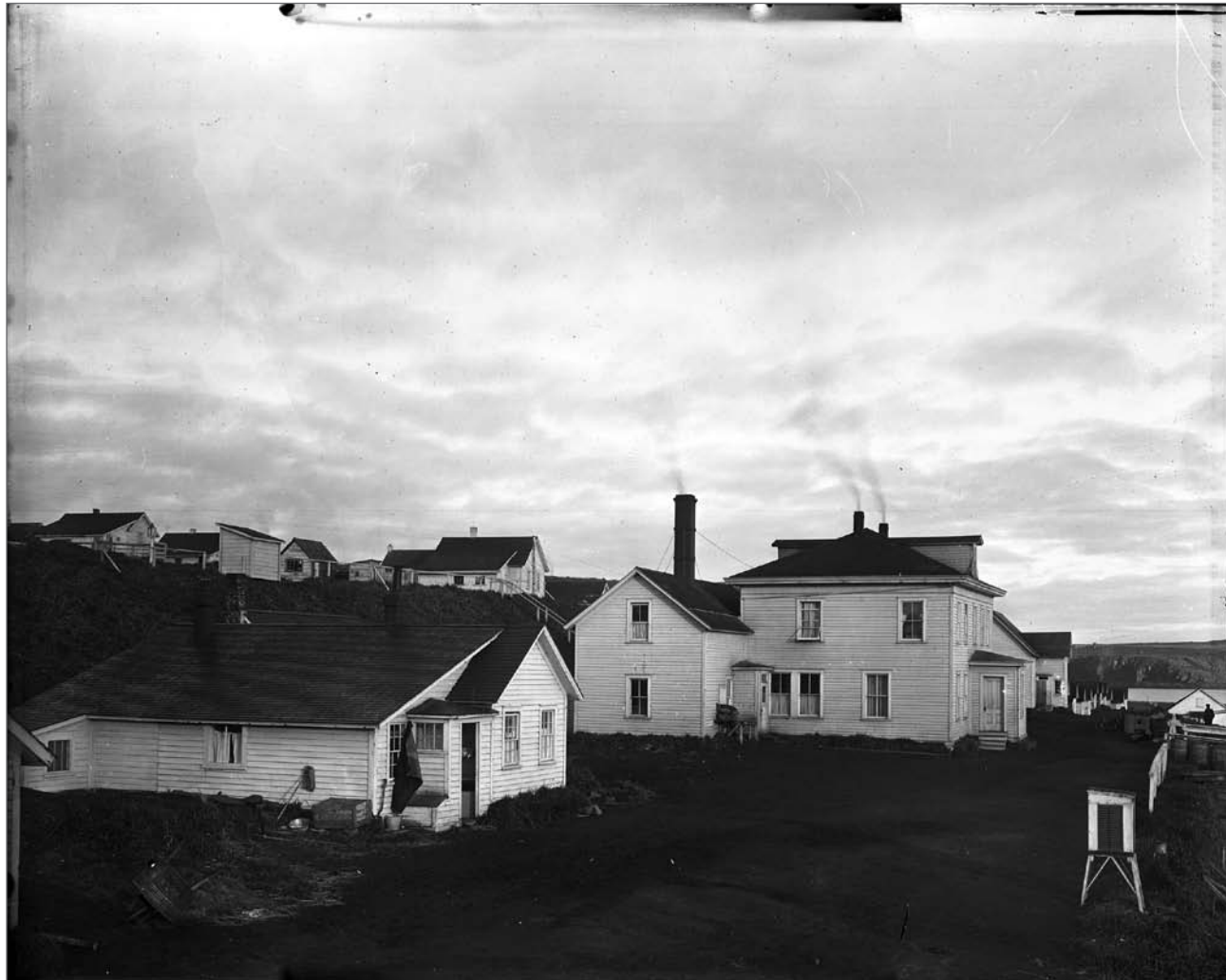
Photograph No. USBF 1.57 (Photographer unknown), n.d.; Stevenson Screen (lower right), St. Paul Island, Alaska, containing meteorological instruments. In 1911, Native carpenters made a Stevenson Screen out of old window shutters found stored in the attic of the Government House. A weather station on St. Paul has collected data from 1872 to the present. Records of the National Oceanic and Atmospheric Administration, RG 370; NARA—Pacific Alaska Region (A).
