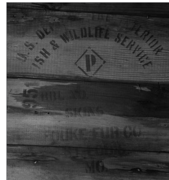
Lindsay, John A., photographer. 2000. Graffiti on ceiling rafters and cross braces; second floor of Salthouse A. Photograph (6x7cm) . NOAA, NOS, Pribilof Project Office, Seattle: sheet JL111381.2, neg. 3874.
