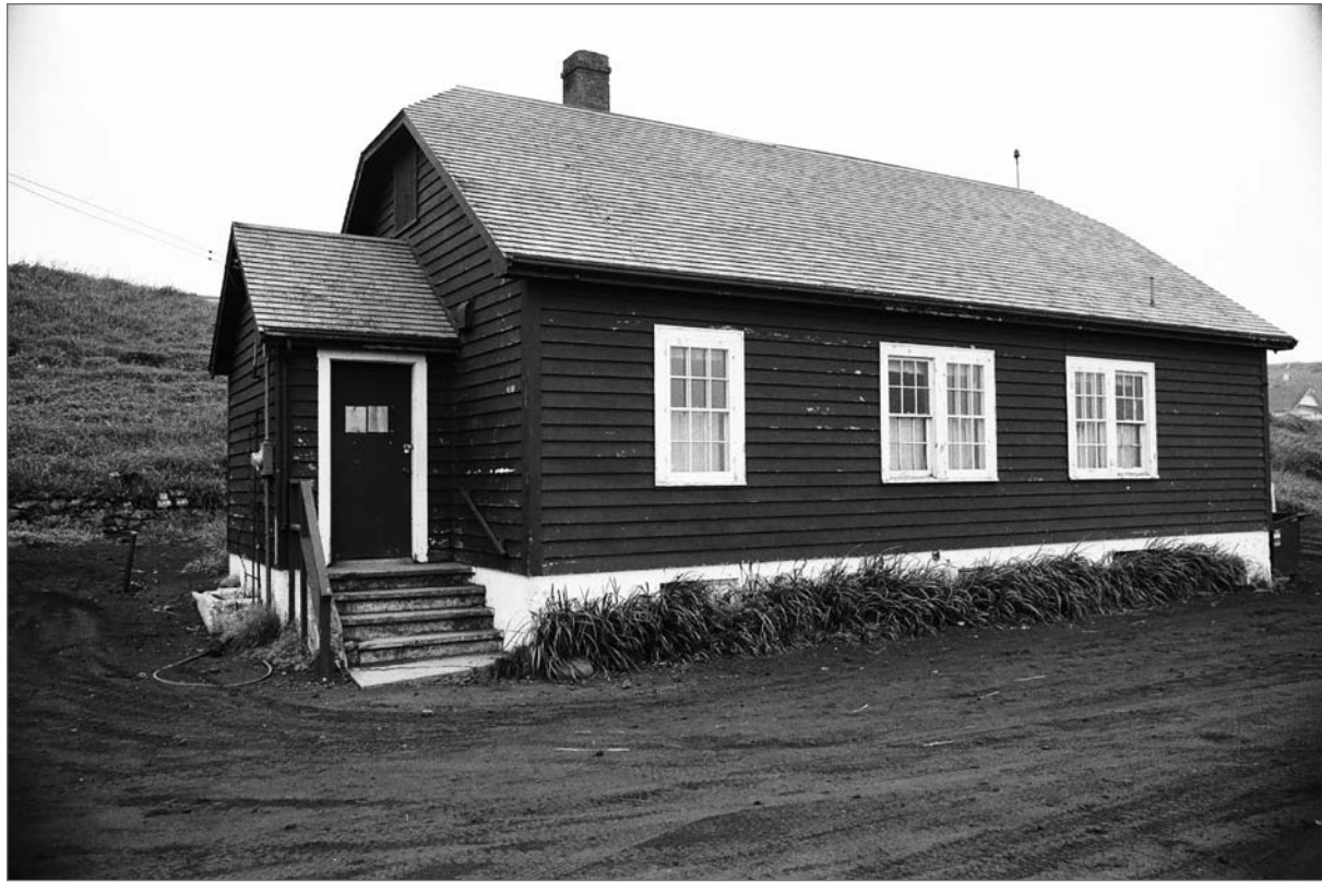
Brodherson, photographer. 1985. South front and east side, former Fisheries Office on Tolstoi Blvd. "Block 18 lot 1 tavern." Photograph. From Faulkner , 1986. Courtesy National Park Service, Anchorage, neg. file 01090036.
