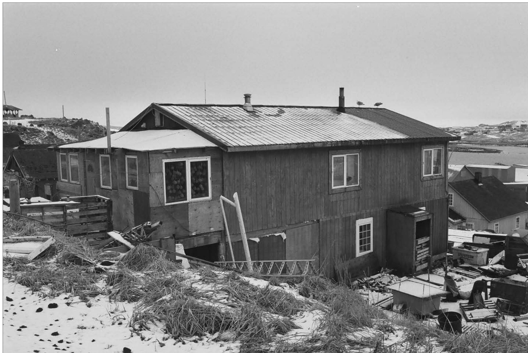
Mobley, Charles, photographer. 2007. West and south sides, Aleut Laborer House 9. Photograph (35mm) . NOAA, NOS, Pribilof Project Office, Seattle.
