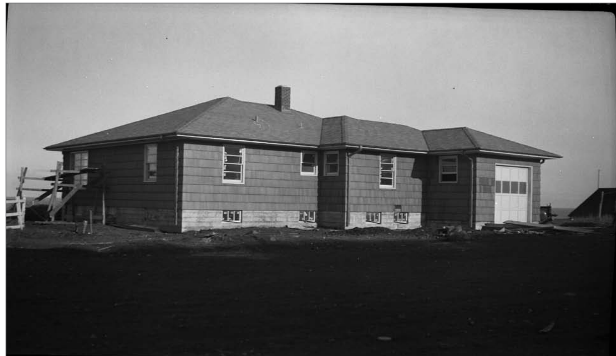
Photograph No. 95-ADMC-3414 (Photographer unknown), 1953; North and west sides, Manager's House/House 115. Records of the National Oceanic and Atmospheric Administration, RG 370; NARA—Pacific Alaska Region (A).
