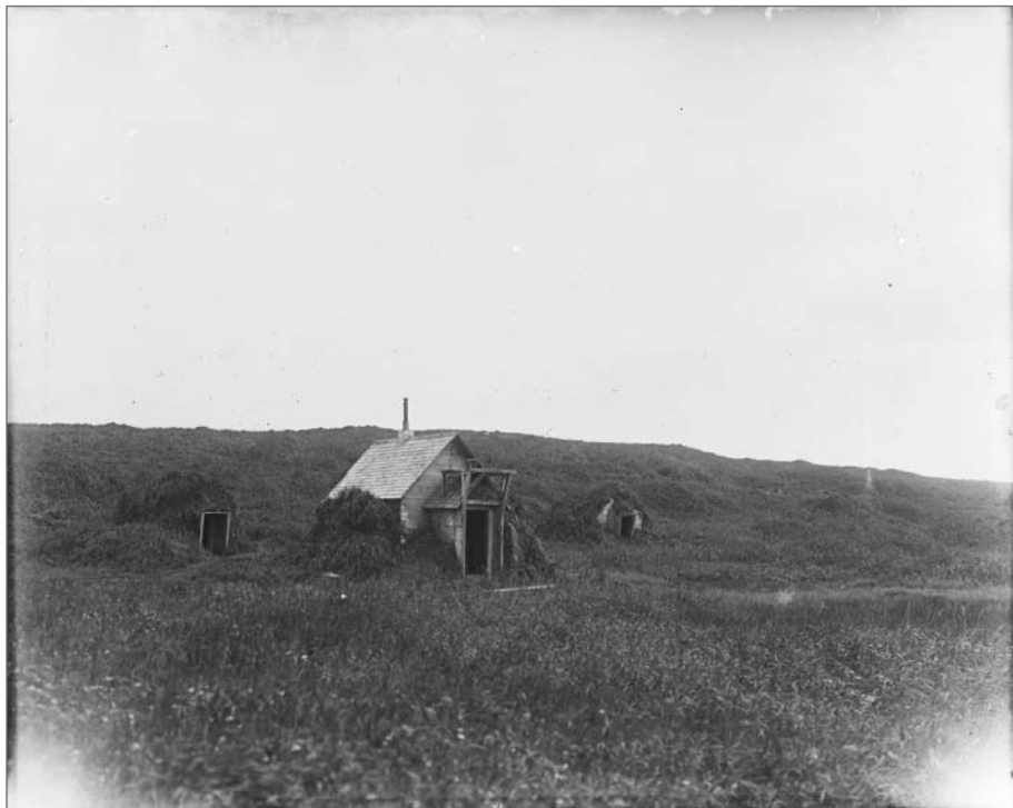
Photograph No. USBF 1.69 (Photographer G Dallas Hanna), 1919; Wells and Pump House, located near site of future By-Products Plant. These wells, approximately 3,000 feet east of the Village, supplied water to residents. In 1915, the Navy installed a small gasoline engine and pump at the wells to deliver water to the Naval Radio Station and village. Water was carefully husbanded because the wells became salty as freshwater was drawn off. Records of the National Oceanic and Atmospheric Administration, RG 370; NARA—Pacific Alaska Region (A).
