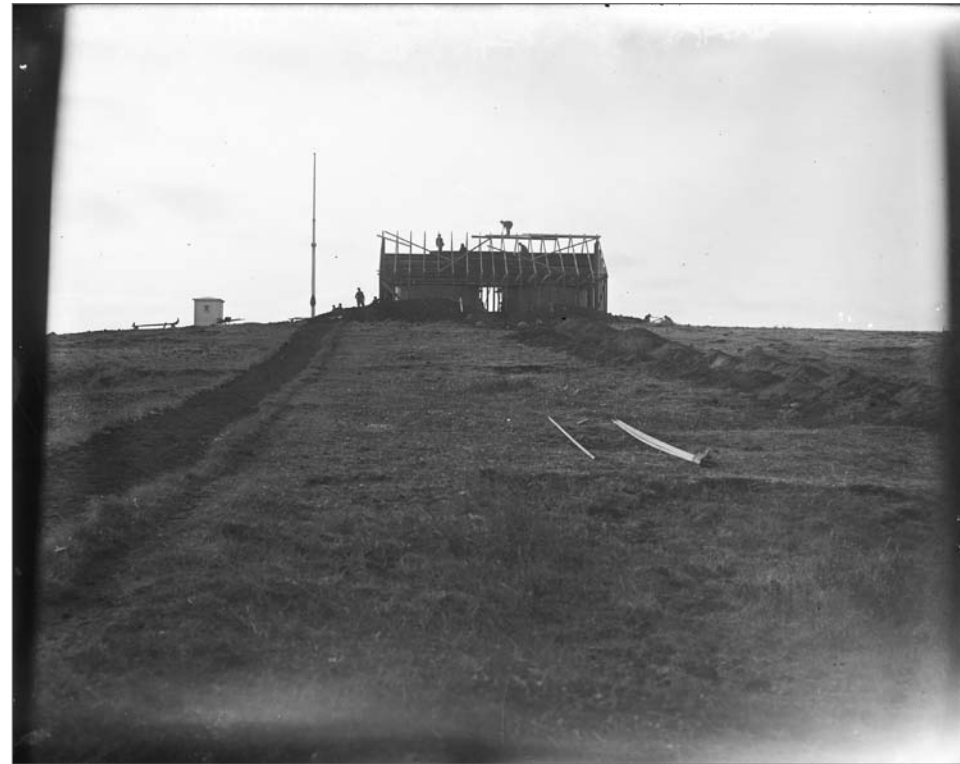
Photograph No. USBF 1.63 (Photographer unknown), 1912; Tank House under construction on Village Hill, showing one of two 20,000-gallon redwood tanks. The small building at left is the Signal House, containing signal flags. Records of the National Oceanic and Atmospheric Administration, RG 370; NARA—Pacific Alaska Region (A).
