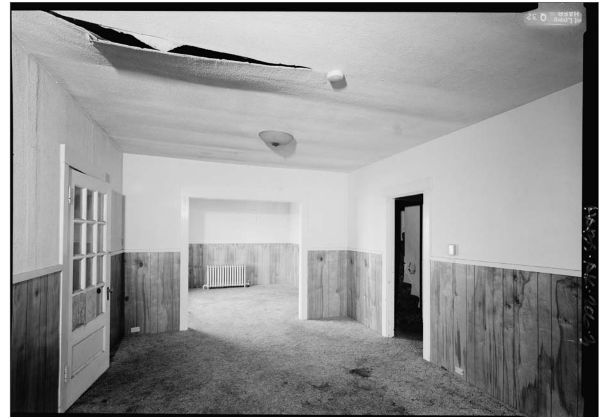
Interior, Teacher House 101, looking from living room to dining room (North to South). Jet Lowe, photographer. Photograph (5x7). Library of Congress: HABS AK-206-3, 2004.
