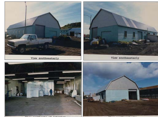
DBS/TRD, photographers. 1985. Various views, Equipment Garage/Halibut Plant. Photograph . From Black-Smith & Richards, 1985.
