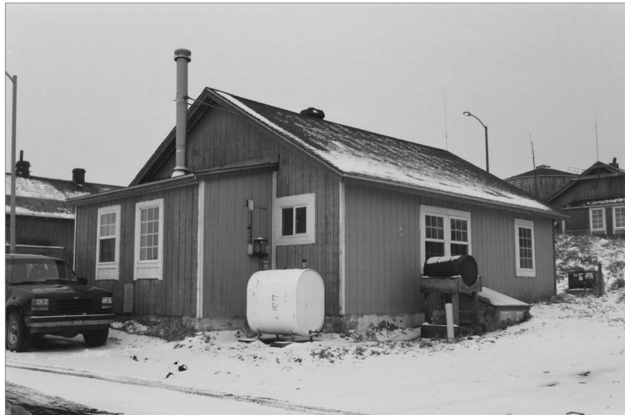
Mobley, Charles, photographer. 2007. East front and north side, Aleut Laborer House 16. Photograph (35mm) . NOAA, NOS, Pribilof Project Office, Seattle.
