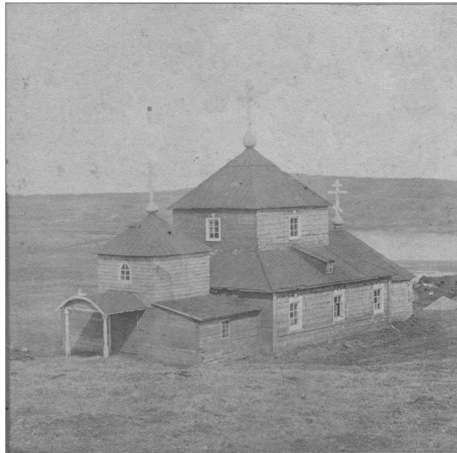
McIntyre, Dr. Hugh H., Alaska Commercial Company Superintendent, photographer. 1872. Chapel, St. Paul Island, constructed of driftwood in 1840. The image is from a stereograph. Courtesy Hugh H. McIntyre III.
