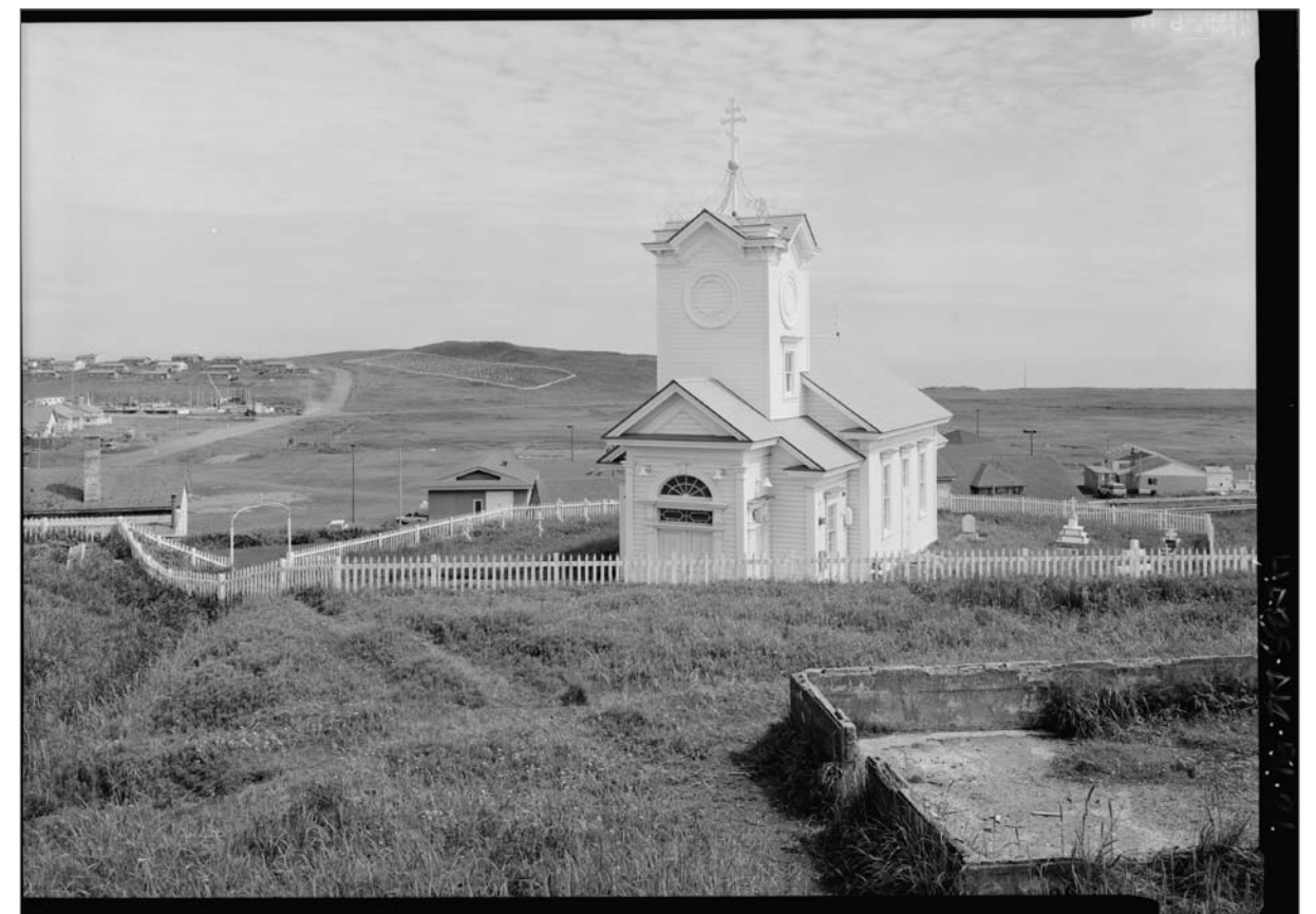
West and south side, Church of the Holy Apostles Saints Peter and Paul, greenhouse foundation in foreground. Jet Lowe, photographer. Photograph (5x7). Library of Congress: HABS AK-51-21 , 2004.
