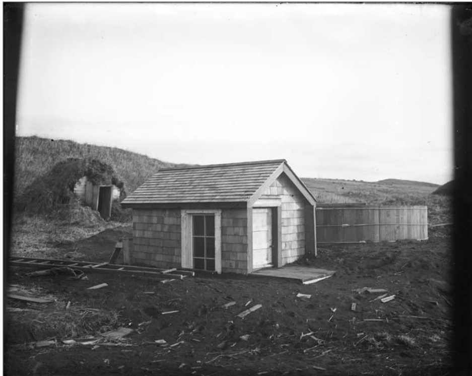
Photograph No. USBF 1.68 (Photographer unknown), 1912; Wells and Pump House. Records of the National Oceanic and Atmospheric Administration, RG 370; NARA—Pacific Alaska Region (A).
