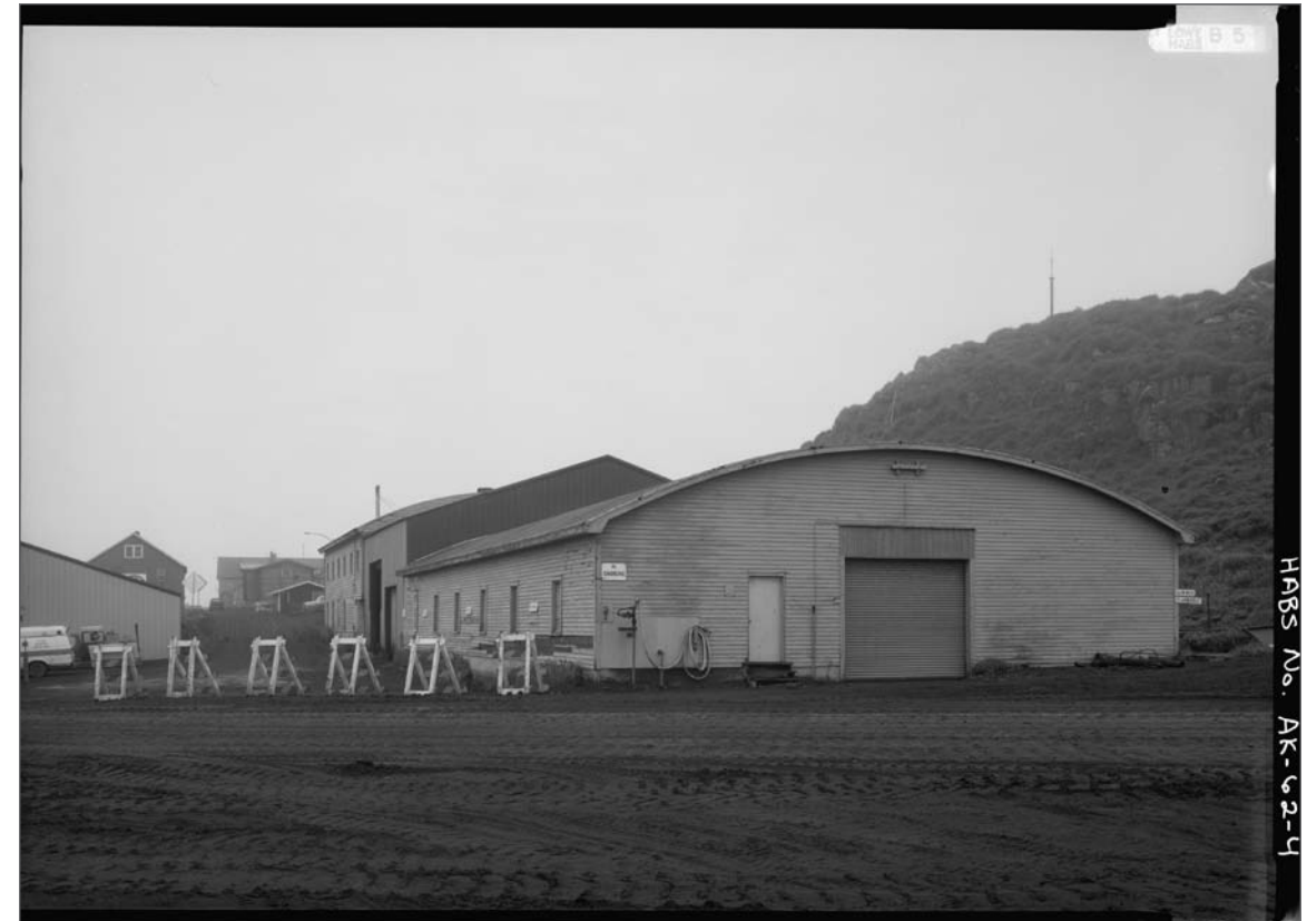
East and north side of former Equipment Garage/Municipal Garage. Jet Lowe, photographer. Photograph. Library of Congress: HABS AK-62-4, 1989.
