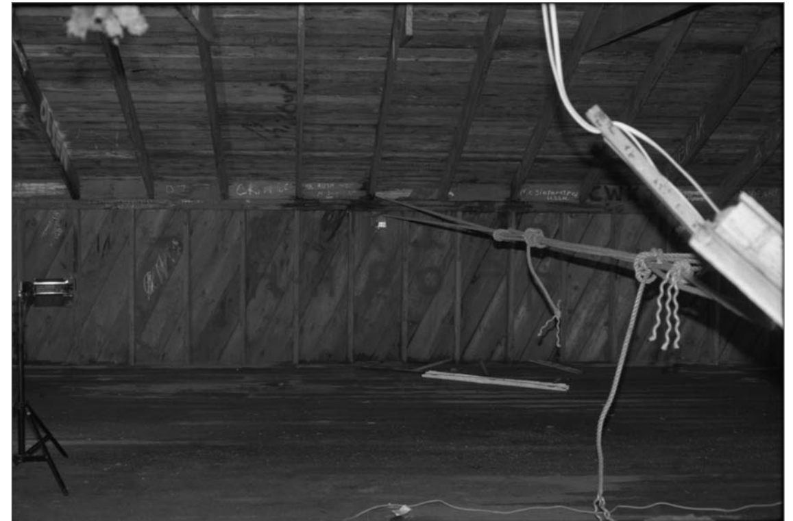
Young, Allison, photographer. 2000. Salthouse A, 2nd floor interior, west wall (north to south: left to right). Note rope linked with the building structure was used to pull the building down. Photograph (35mm). NOAA, NOS, Pribilof Project Office, Seattle: sheet JL 111379.4, neg. 4200, NMML; series includes negatives 4191 through 4202, excluding 4195.
