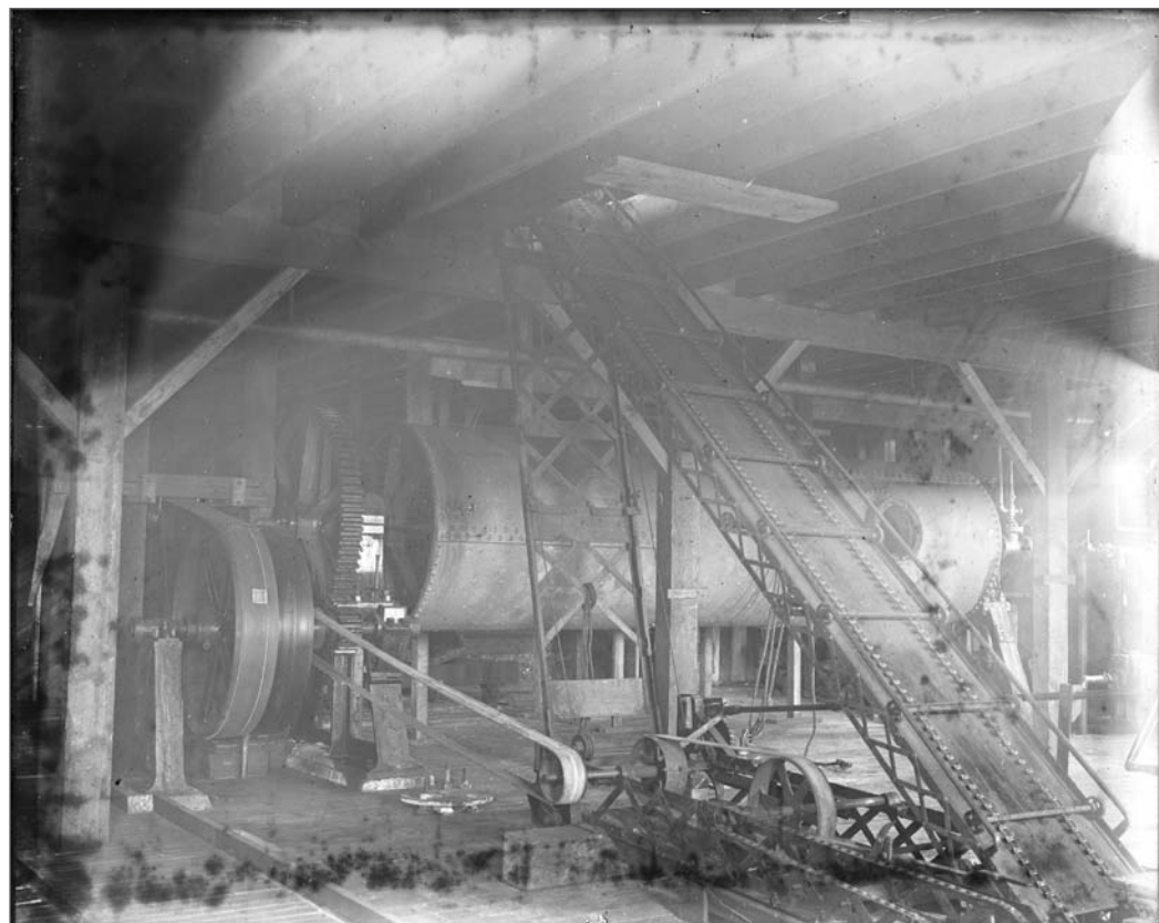
Photograph No. USBF 1.44 (Photographer G Dallas Hanna), 1919; Dryer in By-Products Plant. Records of the National Oceanic and Atmospheric Administration, RG 370; NARA—Pacific Alaska Region (A).
