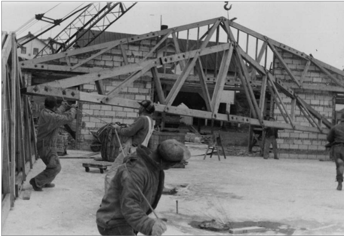
Photograph No. 95-ADMC-1999 (Photographer unknown), 1950's; Men installing trusses, Community Store/Warehouse/Laboratory, looking west. Records of the National Oceanic and Atmospheric Administration, RG 370; NARA—Pacific Alaska Region (A).
