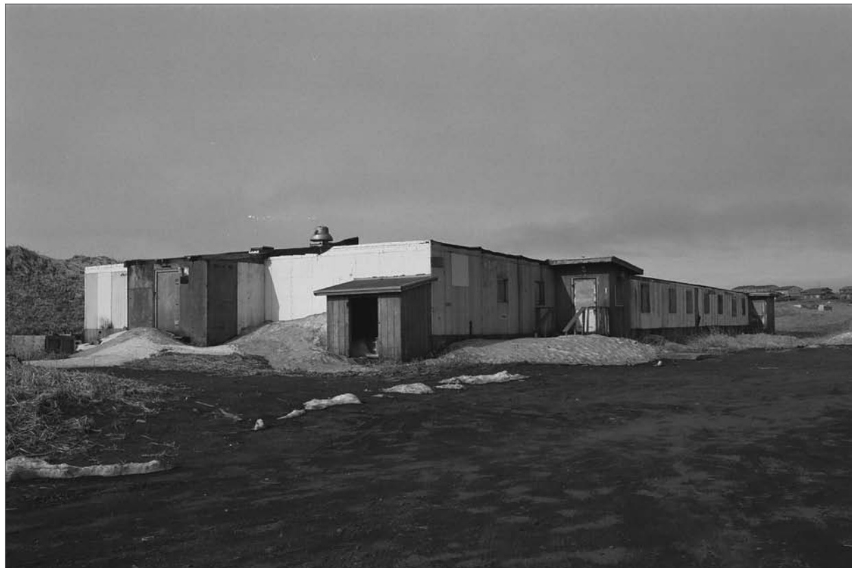
Mobley, Charles, photographer. 2007. West and south sides, former ATCO Trailer Camp. Photograph (35mm). NOAA, NOS, Pribilof Project Office, Seattle.
