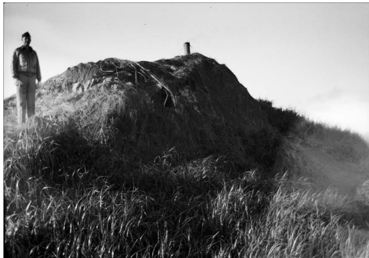
Hill, Evan, photographer. 1943. U.S. Army observation post on Cemetery Hill (Black Bluff), camouflaged with chicken wire and grasses, September 1943. Note: These dugouts are not barabaras. Photograph. Alaska State Library, Historical Collections: PCA 343, Evan Hill Photograph Collection, P343.346.
