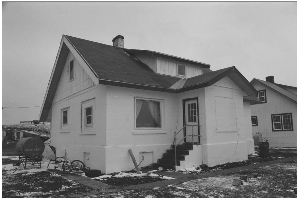
Mobley, Charles, photographer. 2007. South side and east front, Teacher House 103. Photograph (35mm) . NOAA, NOS, Pribilof Project Office, Seattle.
