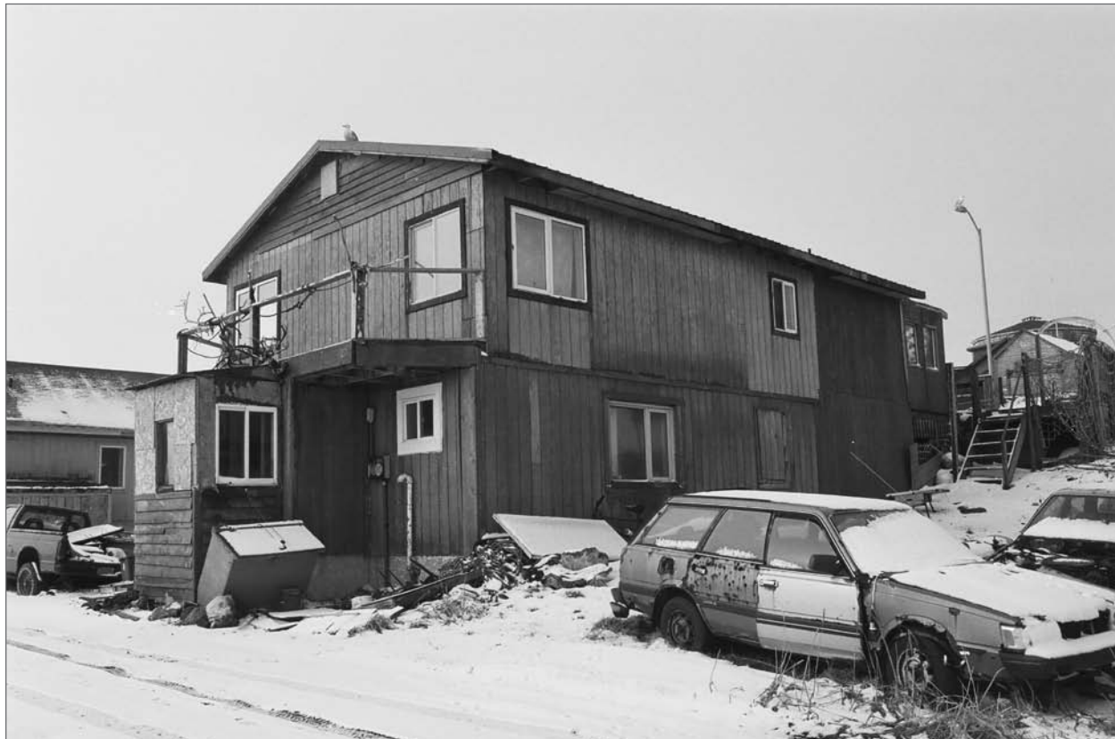
Mobley, Charles, photographer. 2007. East front and north side, Aleut Laborer House 9. Photograph (35mm) . NOAA, NOS, Pribilof Project Office, Seattle.
