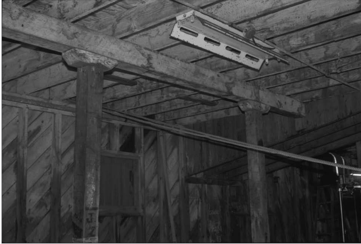
Young, Allison, photographer. 2000. Salthouse A, 1st floor interior, examples of beam framing: beam and post with capitol. Photograph (35mm). NOAA, NOS, Pribilof Project Office, Seattle: sheet JL 110929.3, neg. 4122.
