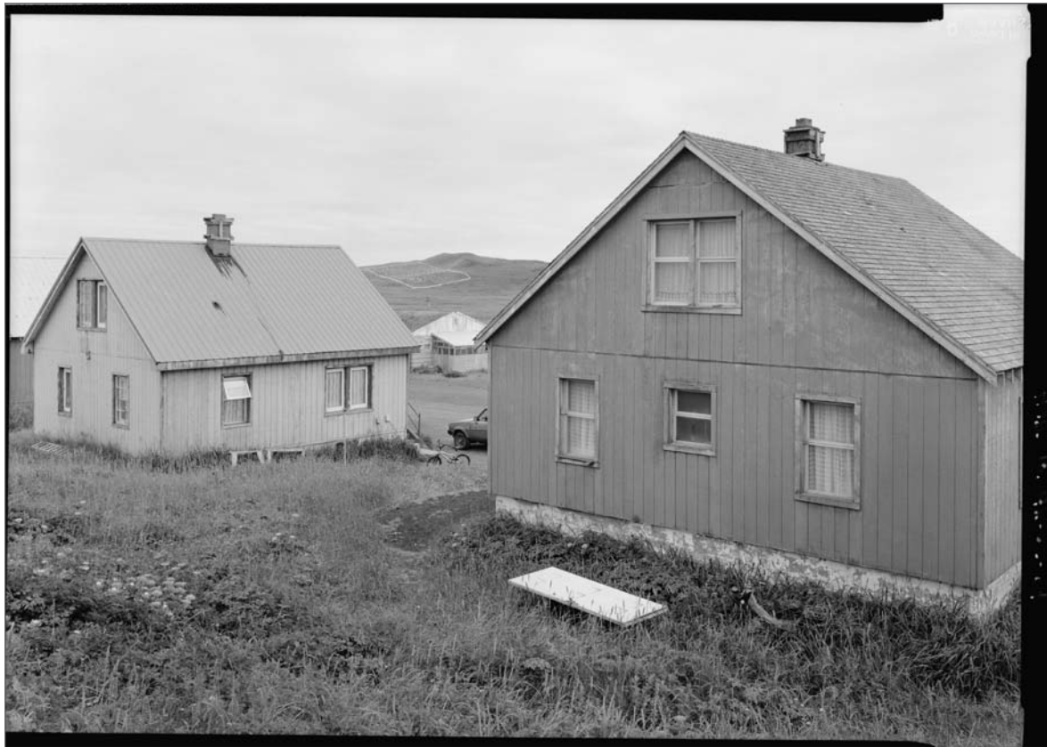
South side of House 53 (left) and House 52 (right). Jet Lowe, photographer. Photograph (5x7). Library of Congress: HABS AK-62-34, 2004.
