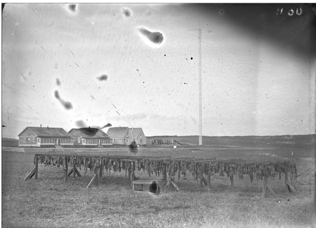
Photograph No. USBF 2.54 (Photographer unknown), 1916; Naval Radio Station, looking northeast. From left: two large quarters, and duplex that housed the radio operator and a power house. Fuel storage tanks for generators are located to the right of the duplex. Fox skin drying racks in foreground. Records of the National Oceanic and Atmospheric Administration, RG 370; NARA—Pacific Alaska Region (A).
