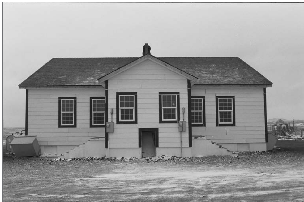
Mobley, Charles, photographer. 2007. North side, Duplex 108/109. Photograph (35mm). NOAA, NOS, Pribilof Project Office, Seattle.
