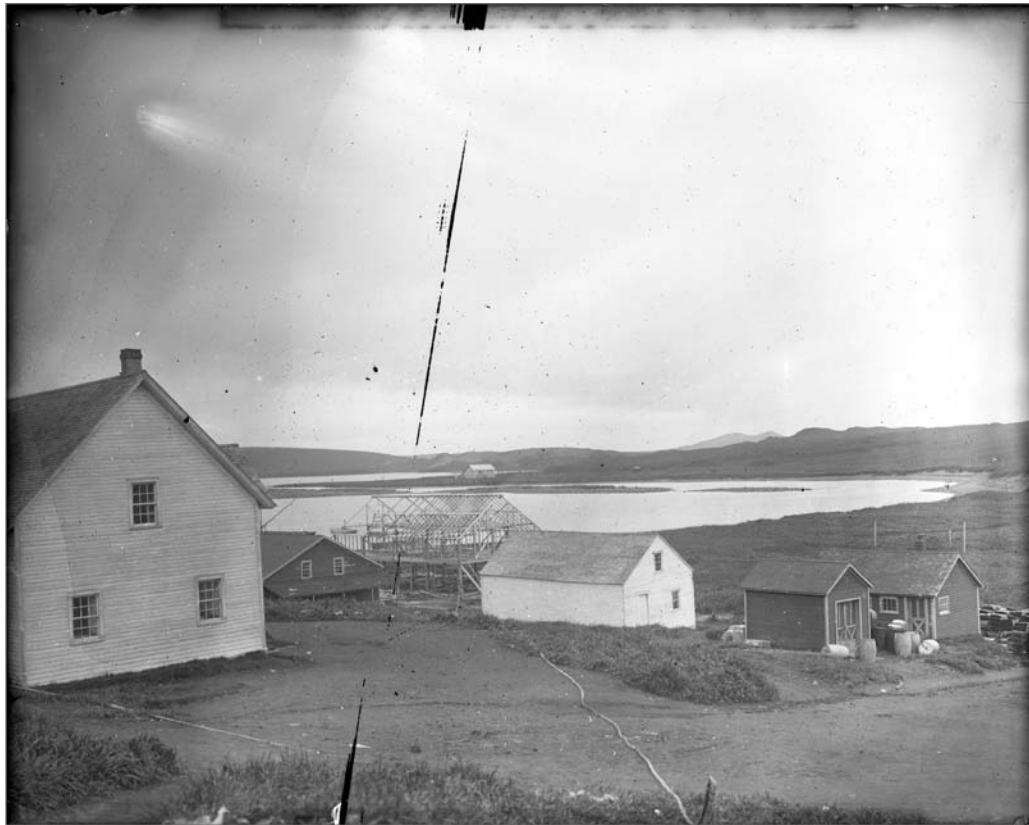
Photograph No. USBF 1.32 (Photographer unknown), n.d.; View from St. Paul Village, showing old Machine Shop (center), old Salthouse (left of Machine Shop), and new Salthouse under construction, with former By-Products Plant in background. Records of the National Oceanic and Atmospheric Administration, RG 370; NARA—Pacific Alaska Region (A).
