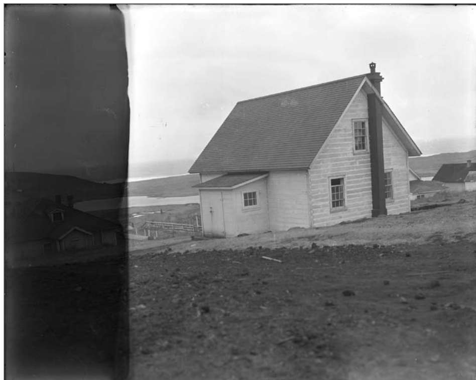
Photograph No. USBF 1.105 (Photographer G Dallas Hanna), November 1914; Former junior schoolhouse. Records of the National Oceanic and Atmospheric Administration, RG 370; NARA—Pacific Alaska Region (A).
