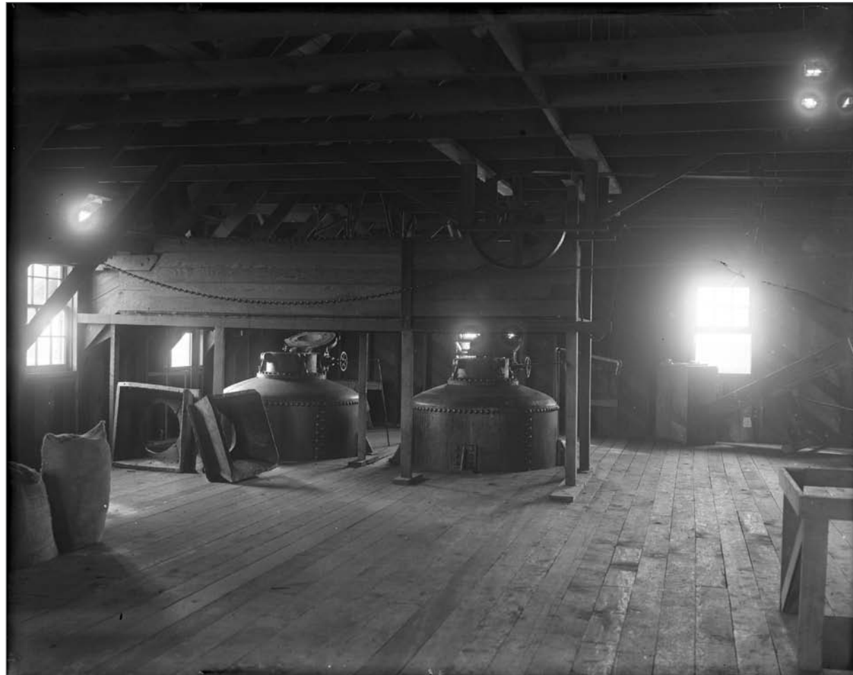
Photograph No. USBF 1.43 (Photographer G Dallas Hanna), 1919; Interior, By-Products Plant, showing retorts. Records of the National Oceanic and Atmospheric Administration, RG 370; NARA—Pacific Alaska Region (A).
