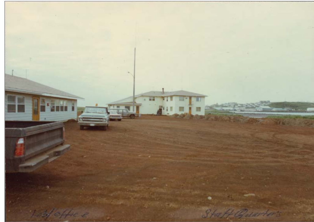
Photograph No. 95-ADMC-1101 (Photographer unknown), 1977; Laboratory (left) and Staff Quarters (right), looking south, with St. Paul Village across Village Cove. Records of the National Oceanic and Atmospheric Administration, RG 370; NARA—Pacific Alaska Region (A).
