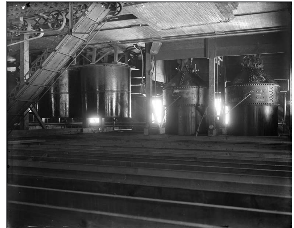
Photograph No. USBF 1.40 (Photographer G Dallas Hanna), 1919; Interior, By-Products Plant, showing rendering tanks. Records of the National Oceanic and Atmospheric Administration, RG 370; NARA—Pacific Alaska Region (A).
