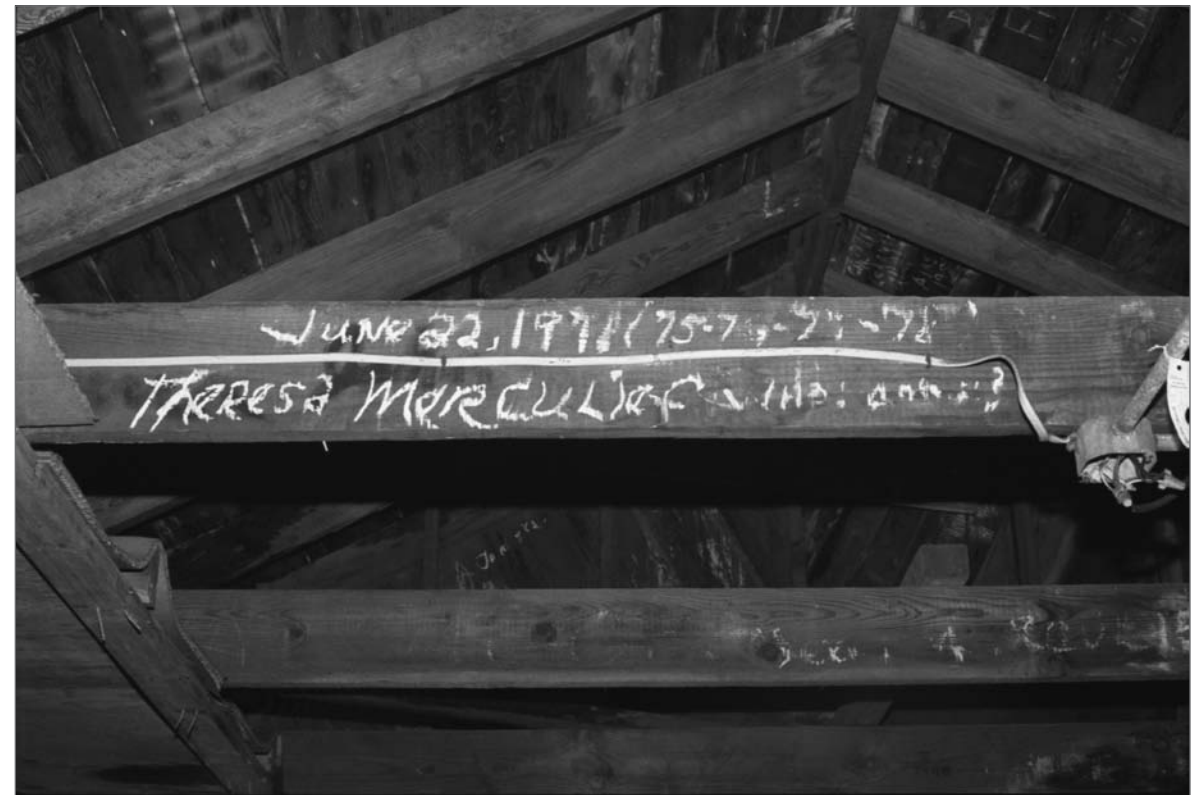
Young, Allison, photographer. 2000. Chalk "June 22, 1971 [illegible], 74, 75, 76, 77, 78 Theresa Merculief [illegible]," also electrical line leading to junction box, on joist, 2nd floor Salthouse A. Photograph (35mm). NOAA, NOS, Pribilof Project Office, Seattle: sheet JL 111379.2, neg. 4097.
