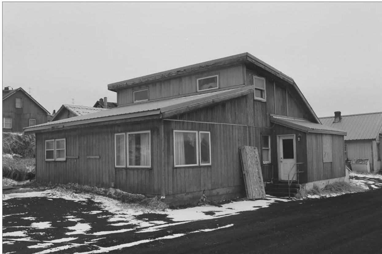
Mobley, Charles, photographer. 2007. South side and east front, Aleut Laborer House 50. Photograph (35mm) . NOAA, NOS, Pribilof Project Office, Seattle.
