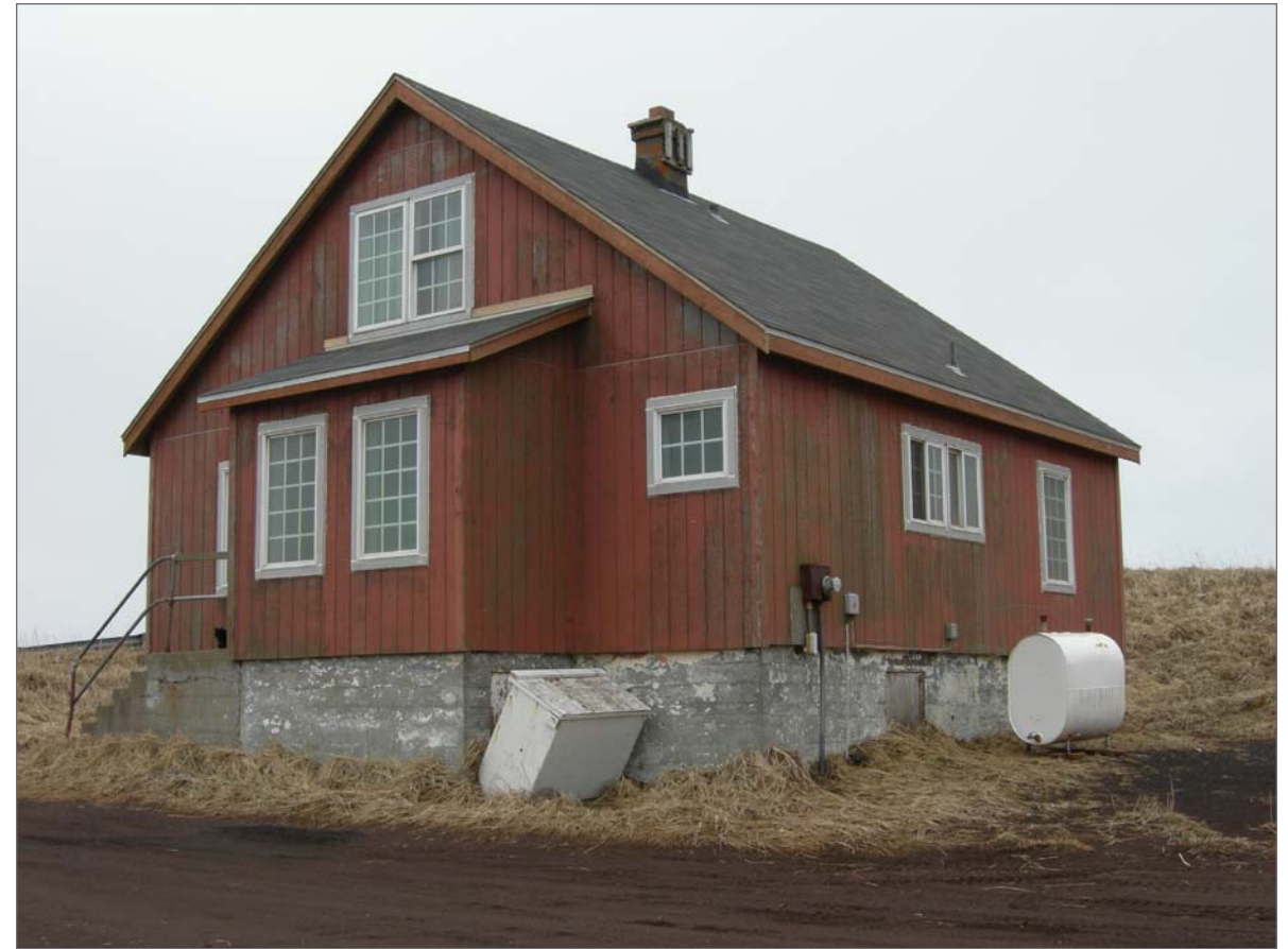
Mobley, Charles, photographer. 2007. East front and north side, Aleut Laborer House 52. Photograph (35mm). NOAA, NOS, Pribilof Project Office, Seattle.
