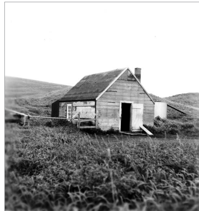
Photograph No. 95-ADMC-3089 (Photographer unknown), n.d.; Pump House at Icehouse Lake. Records of the National Oceanic and Atmospheric Administration, RG 370; NARA—Pacific Alaska Region (A).
