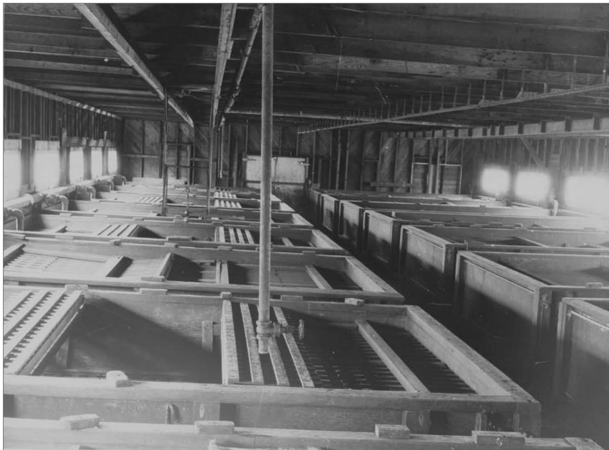
Photograph No. 95-ADMC-181 (Photographer unknown), n.d.; Interior of wash house. Records of the National Oceanic and Atmospheric Administration, RG 370; NARA—Pacific Alaska Region (A).
