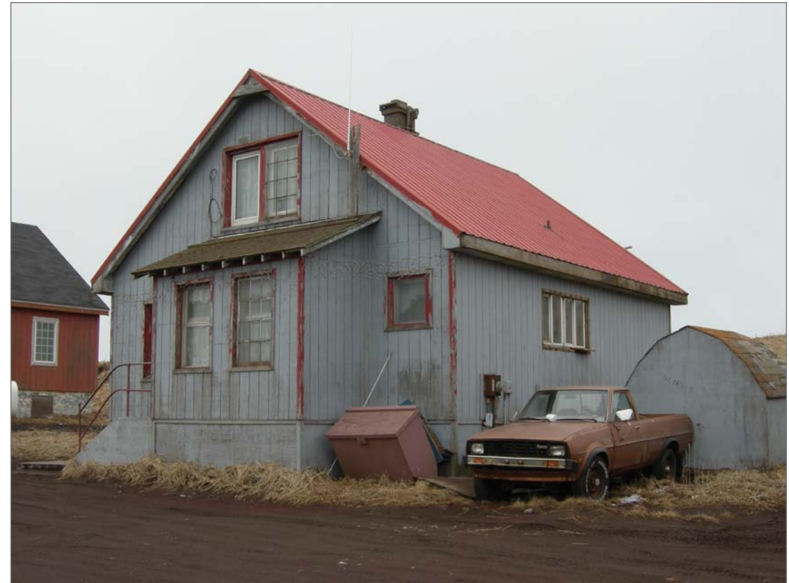
Mobley, Charles, photographer. 2007. East front and north sides, Aleut Laborer House 53. Photograph (35mm). NOAA, NOS, Pribilof Project Office, Seattle.
