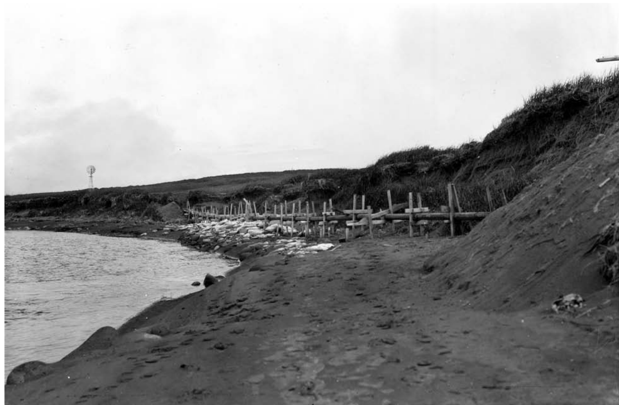
Photograph No. 22-MP-3-32 (Photographer Harry J. Christoffers), 1928; Icehouse Lake windmill in background and exposed freshwater pipeline along Salt Lagoon between Icehouse Lake and village. Records of the National Oceanic and Atmospheric Administration, RG 370; NARA—Pacific Alaska Region (A).
