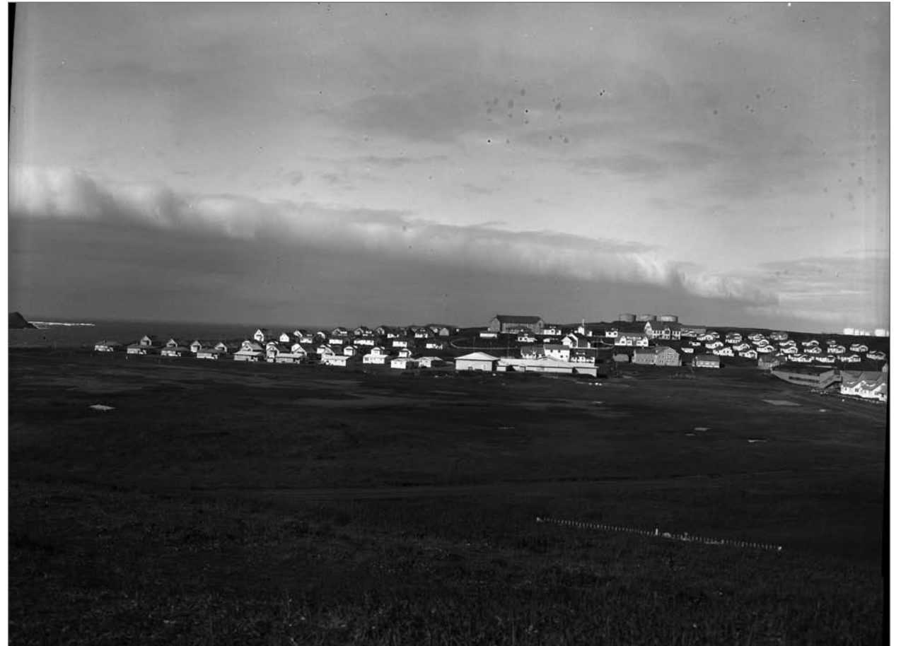
Photograph No. 95-ADMC-3248 (Photographer unknown), circa 1975; Panoramic view of St. Paul Village, note houses 122–128 (left foreground) on Lakeside Street. Records of the National Oceanic and Atmospheric Administration, RG 370; NARA—Pacific Alaska Region (A).
