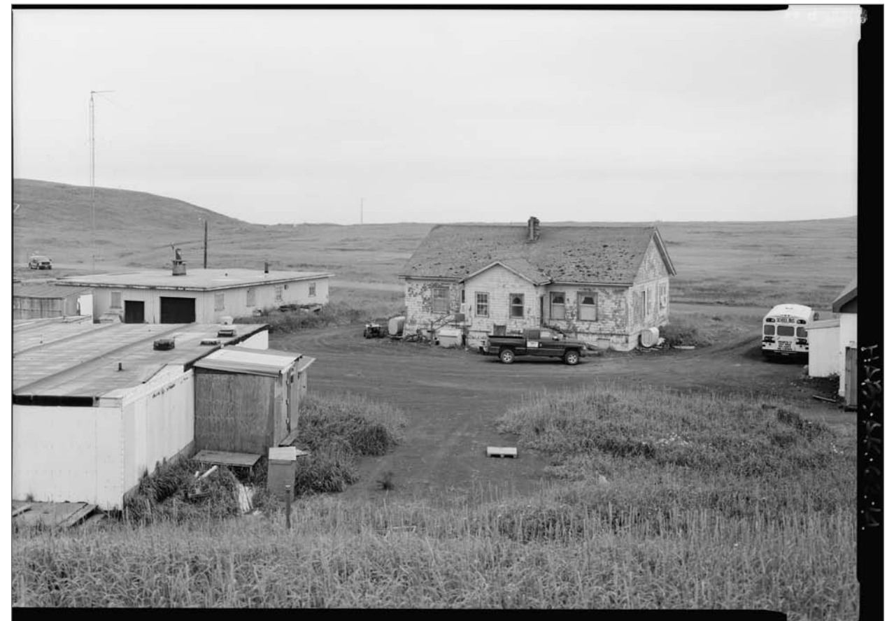
North and west sides, Duplex 108/109, with ATCO trailer camp in the foreground. Jet Lowe, photographer. Photograph (5x7) . Library of Congress: HABS AK-62-14, 1989.
