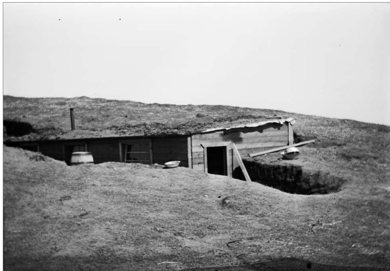
Hill, Evan, photographer. 1943. U.S. Army observation post on Cemetery Hill (Black Bluff), camouflaged with chicken wire and grasses, September 1943. Note: These dugouts are not barabaras. Photograph. Alaska State Library, Historical Collections: PCA 343, Evan Hill Photograph Collection, P343.361.
