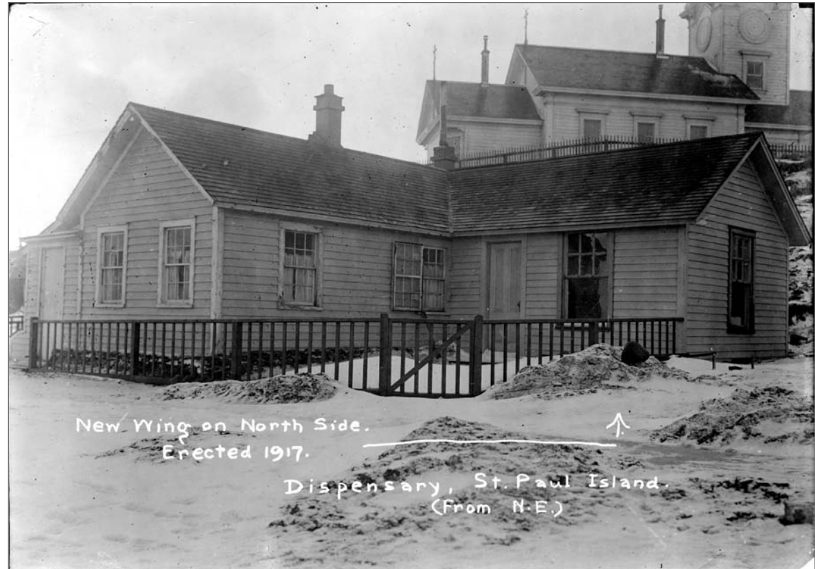
Photograph No. 22-MP-3-36 (Photographer unknown), 1917; East and north sides, Dispensary, showing new wing on north side of building with church in background. Records of the National Oceanic and Atmospheric Administration, RG 370; NARA—Pacific Alaska Region (A).
