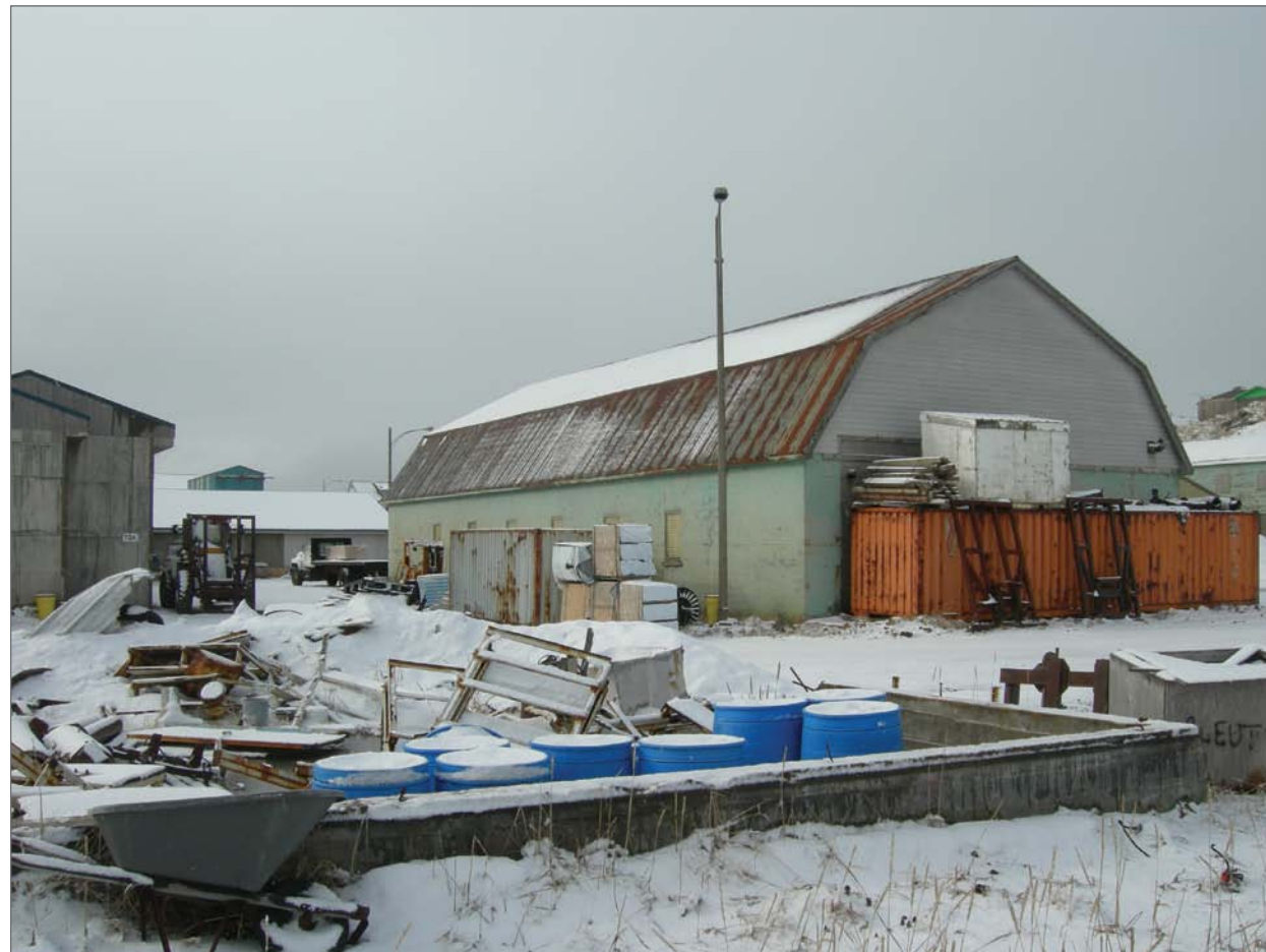
Mobley, Charles, photographer. 2007. East and north sides, Equipment Garage/Halibut Plant. Photograph (35mm) . NOAA, NOS, Pribilof Project Office, Seattle.
