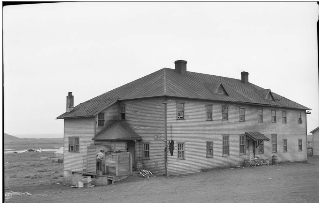
Photograph No. 22-RB-1949-36 (Photographer unknown), 1949; West and north sides, Aleutian Bunkhouse. Records of the U.S. Fish and Wildlife Service, RG 22; NARA, Special Media Archives Services Division, National Archives at College Park, College Park, MD.
