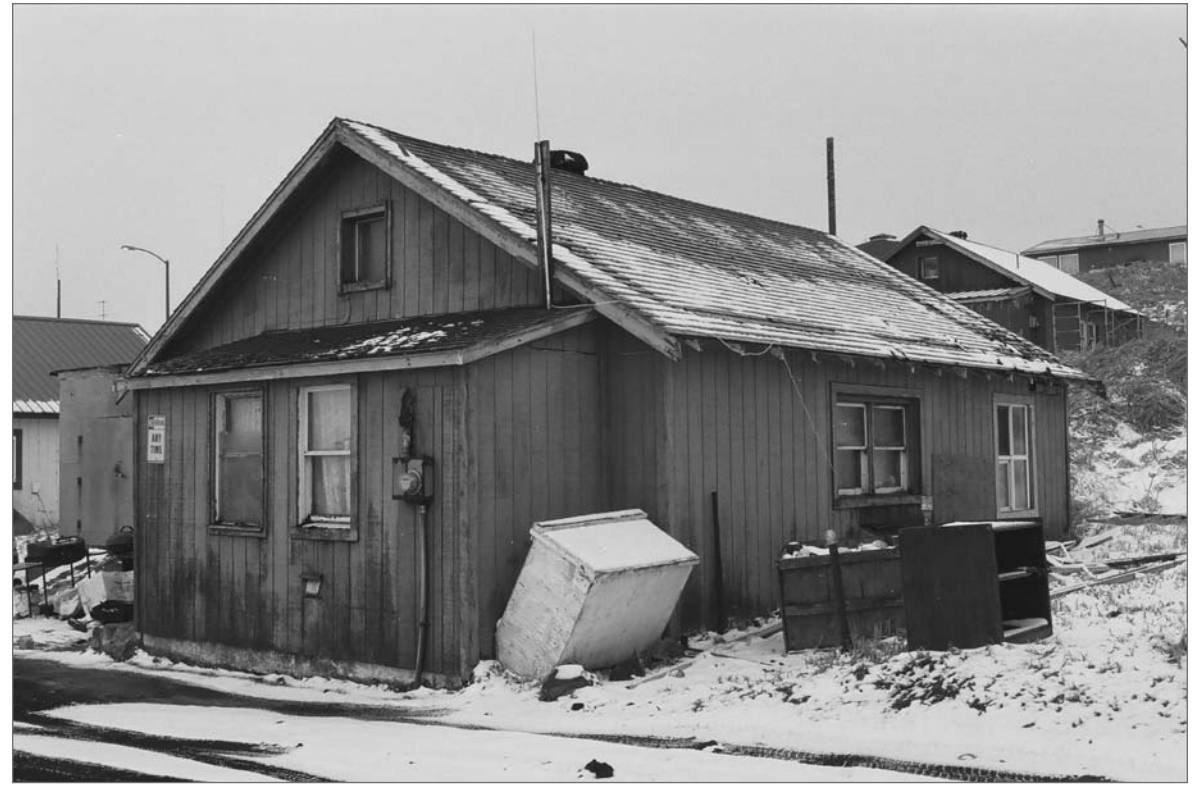
Mobley, Charles, photographer. 2007. East front and north side, Aleut Laborer House 18. Photograph (35mm). NOAA, NOS, Pribilof Project Office, Seattle.
