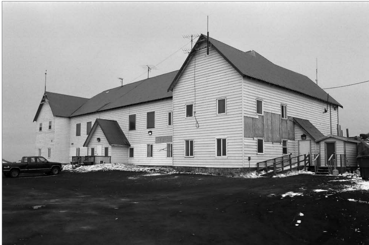
Mobley, Charles, photographer. 2007. East and north sides, Recreation Hall. Photograph (35mm) . NOAA, NOS, Pribilof Project Office, Seattle.
