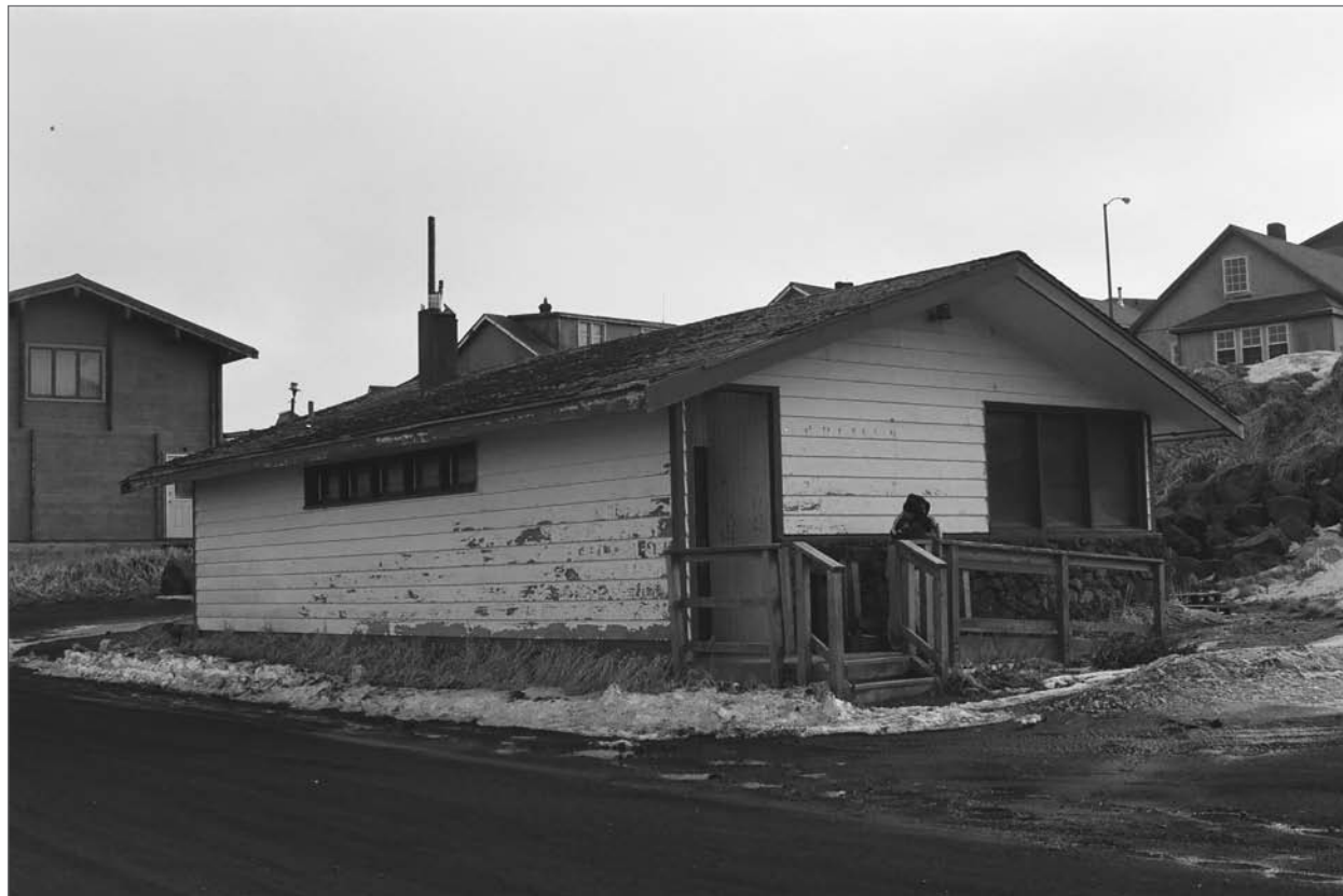
Photograph No. 95-ADMC-3174 (Photographer unknown), circa 1968; East and north sides, Old Post Office/Duna's Kitchen. Records of the National Oceanic and Atmospheric Administration, RG 370; NARA—Pacific Alaska Region (A).
