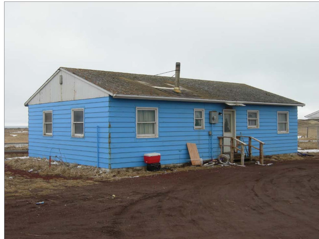
Mobley, Charles, photographer. 2007. North and west sides, Aleut Laborer House 128. Photograph (35mm). NOAA, NOS, Pribilof Project Office, Seattle.
