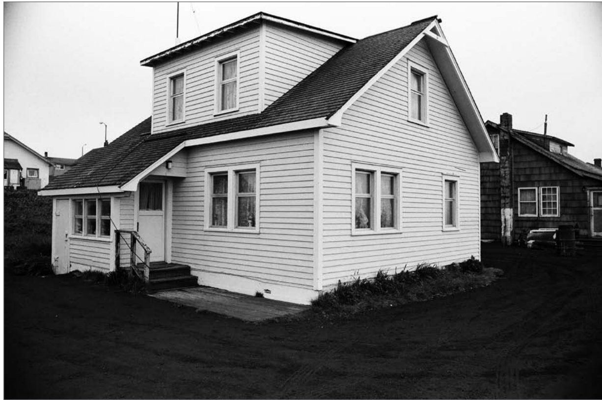
Brodherson, photographer. 1985. South front and east side, Aleut Laborer House 42 "Block 13 lot 2...Native 1918 type." Photograph. From Faulkner, 1986. Courtesy National Park Service, Anchorage, neg. file 01090018.
