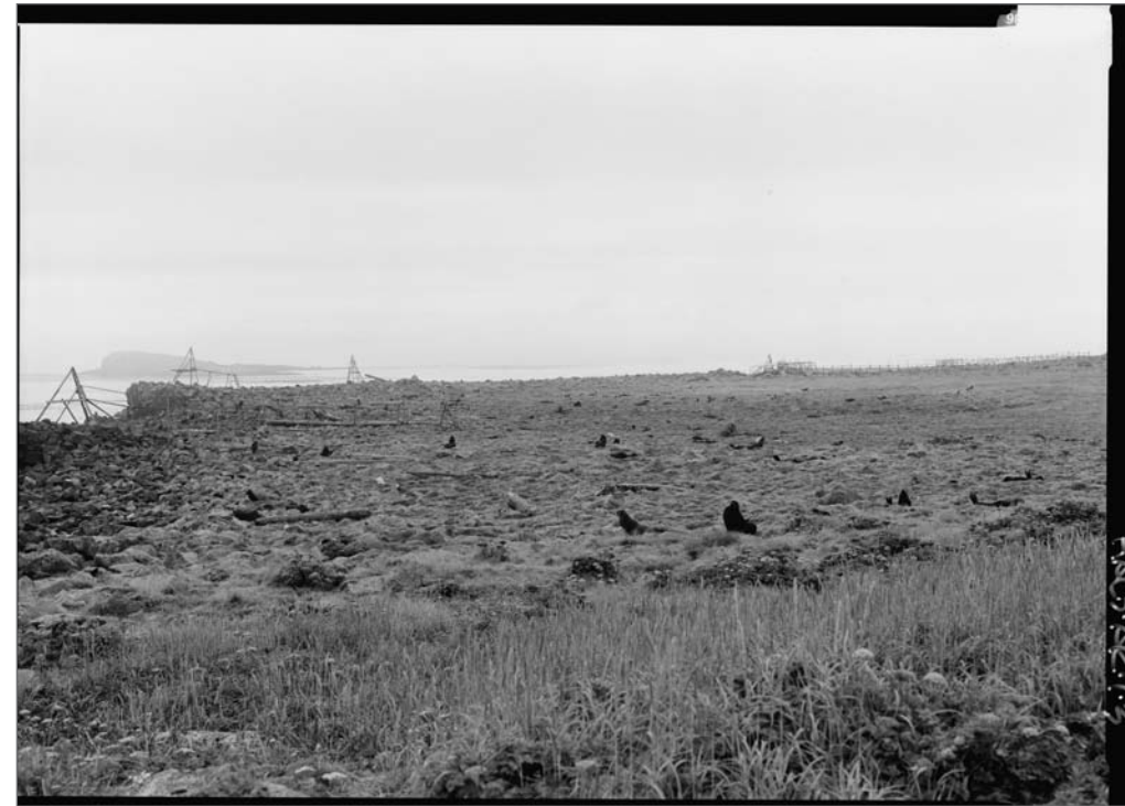
View of the Reef Rookery, looking southwest toward Sea Lion Rock. Jet Lowe, photographer. Photograph (5x7). Library of Congress: HALS AK-1-3 , 2004.
