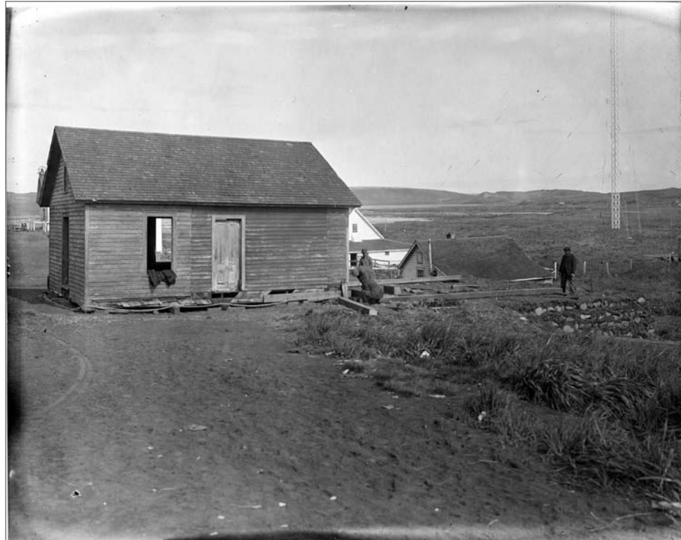
Photograph No. USBF 1.76 (Photographer Hanna, G Dallas), 1914; Men moving a wooden building. This building was probably an old store house that was relocated across the street from the dispensary for use as a hospital. Buildings were frequently disassembled or relocated due to the scarcity of materials on the Pribilof Islands. Records of the National Oceanic and Atmospheric Administration, RG 370; NARA—Pacific Alaska Region (A).
