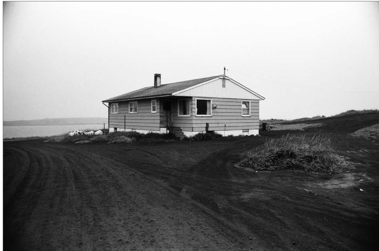
Brodherson, photographer. 1985. East front and north side, Aleut Laborer House 120. Photograph. From Faulkner, 1986. Courtesy National Park Service, Anchorage, neg. file 01090022.
