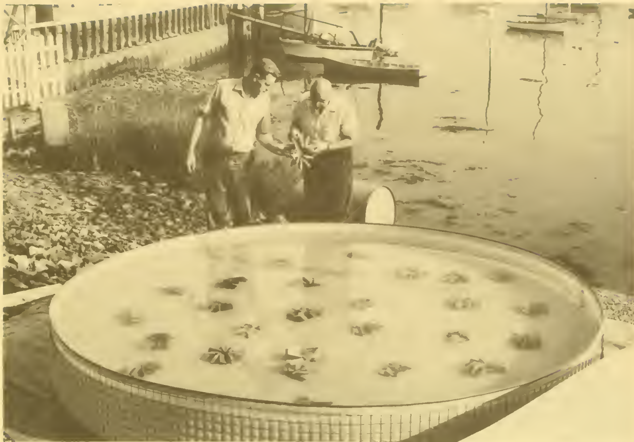
Figure 11.--Biologists experimenting with artificial collectors for oyster set to find a substitute for old shells, which are not easily available in some areas where oysters are cultivated. Artificial collectors may also be used in oyster hatcheries where mature larvae will be released to set on them after they are placed in small ponds or tanks similar to the one shown in photograph.
