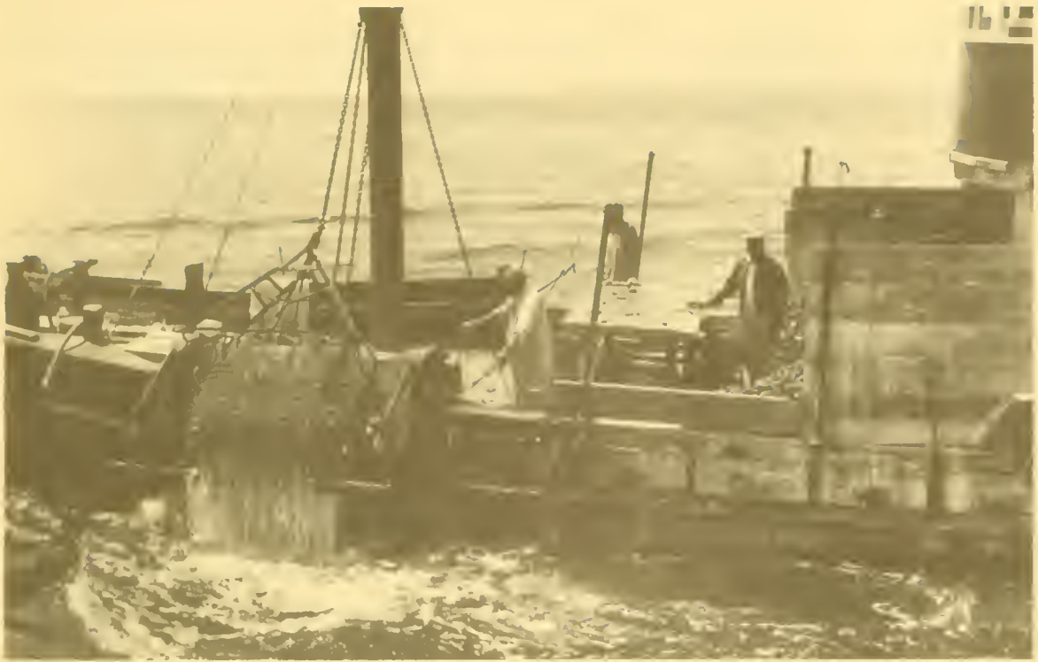
Figure 22.--Conventional type of machine-operated oyster dredge widely used on private oyster grounds.
