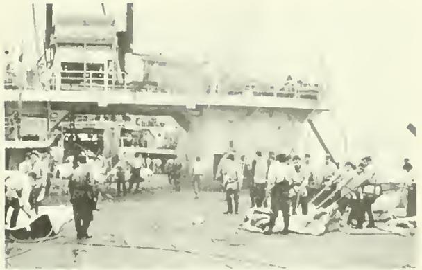
Final stages of whale butchering on Japanese whale factory ship. After the whale has been completely stripped, the large strips of blubber are cut into smaller pieces and sent below deck for rendering into oil. Meat is frozen for human food or animal feed. The bones are sawed into pieces for reduction to meal, and only the entrails are discarded. It takes less than 15 minutes to completely butcher a whale.
