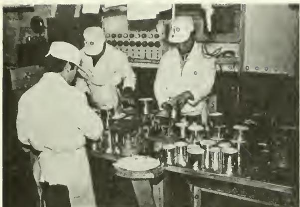
Cans of hand-packed king crab meat being checked for appropriate weight on Japanese factory ship in eastern Bering Sea. Inspected cans are conveyed to next compartment where they are sealed and then cooked in retorts.
