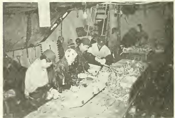
King crab meat being shaken from the shells in a Japanese factory ship in the eastern Bering Sea. Complete processing is done on the fishing grounds, largely by hand labor.
