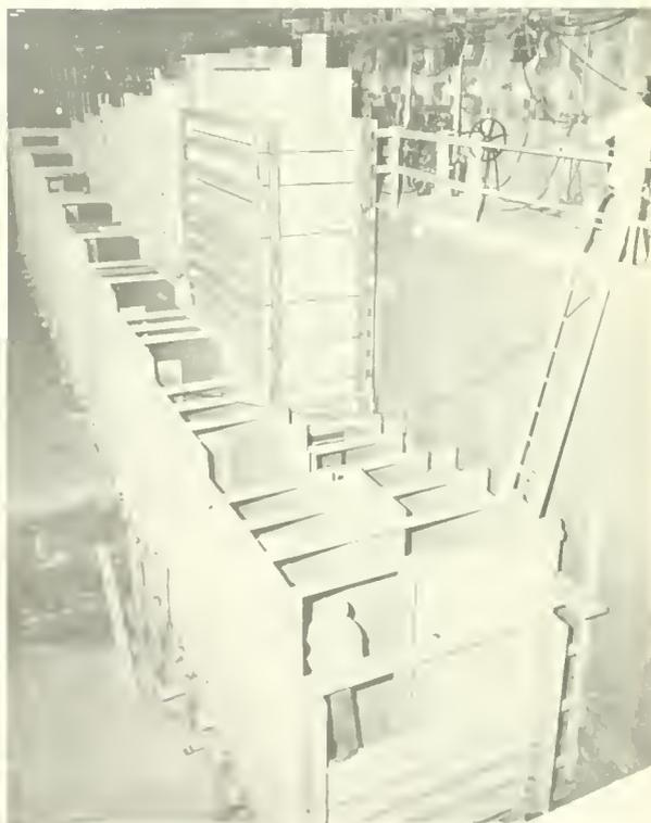
Figure 8.—The 16-pool, 1-on-8-slope endless fishway nearing completion. Worker stands in fish entry gate. Locking unit for lowering and recycling fish appears in center.
