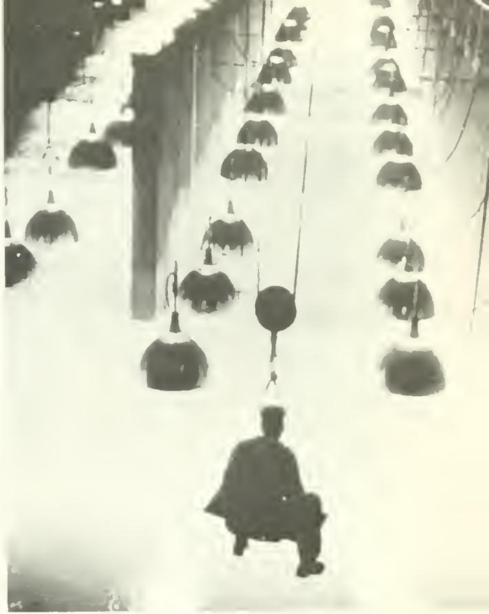
Figure 6.—Full-scale experimental fishways in operation. Standard lighting conditions are created by mercury-vapor lamps. Picketed barriers and release gates for the control of fish have yet to be erected.
