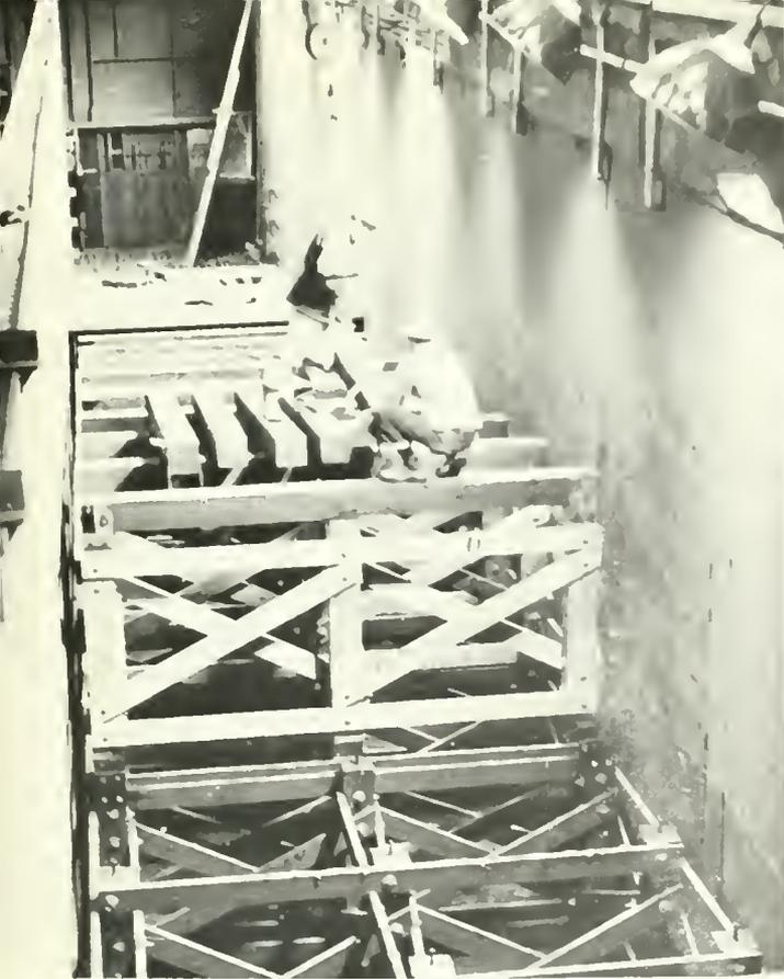
Figure 5.—Experimental fishways under construction. Careful planning and great ingenuity are required in building temporary structures capable of supporting and controlling large volumes of water.
