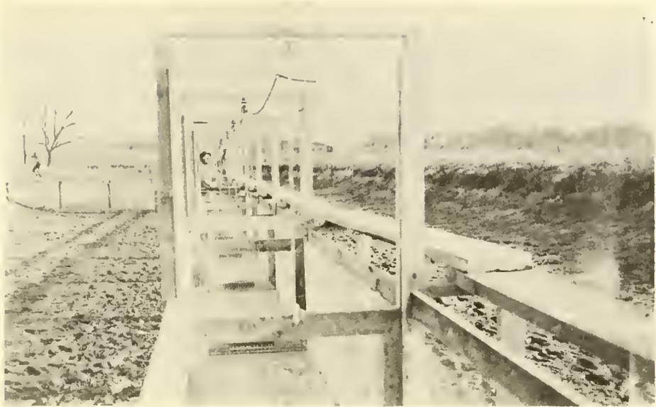
Figure 2. Dry pond, trap structure completed, gates rigged and in place.
