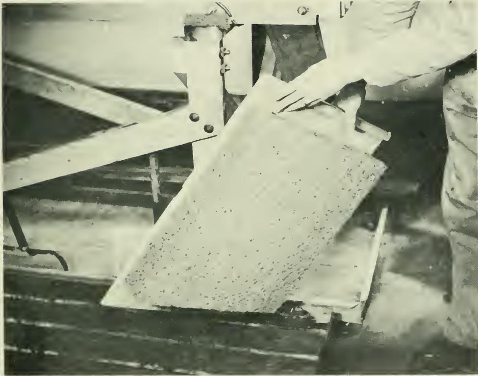
Figure 4. --One of the covers from the experimental tank showing the 3-inch layer of rubberized horsehair used to soundproof the entire inner surface of the tank. In the tank, there was a layer of 1-inch foam rubber under the layer of horsehair.
