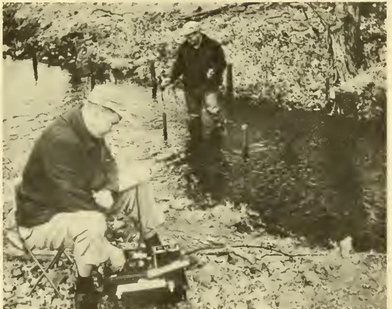
Figure 10.--Using the conductivity bridge for determining apparent velocity in the controlled-flow channel at Mill Creek. Operator in background is dropping conductivity cell into the chamber of a standpipe.
