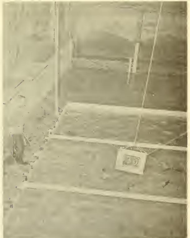
Figure 5.--The main tank as used in studies of electrostatic response of adult squawfish. An electrode array was enclosed within the tank and was energized by the generator and electronic pulse unit on the deck.
