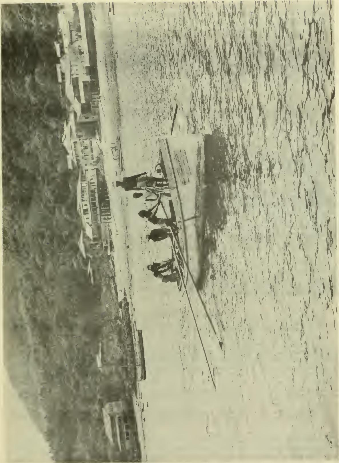
Figure 3 --- Pearl-fishing boat used for diving during the expedition. Mast and sails were removed. Air pump is located in the middle.
