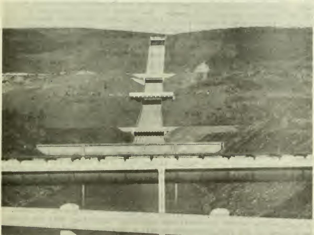
Figure 4.-- Irrigation ditches from the Yakima River crossing the Terrace Heights Wasteway of the Roza Canal near Yakima, Washington. Crossing from top to bottom are: Roza Canal; Selah - Moxee Canal; Highway bridge; Ray Slavin Branch of the Moxee Ditch; Middy Branch of the Moxee Ditch; Union Gap Ditch.
