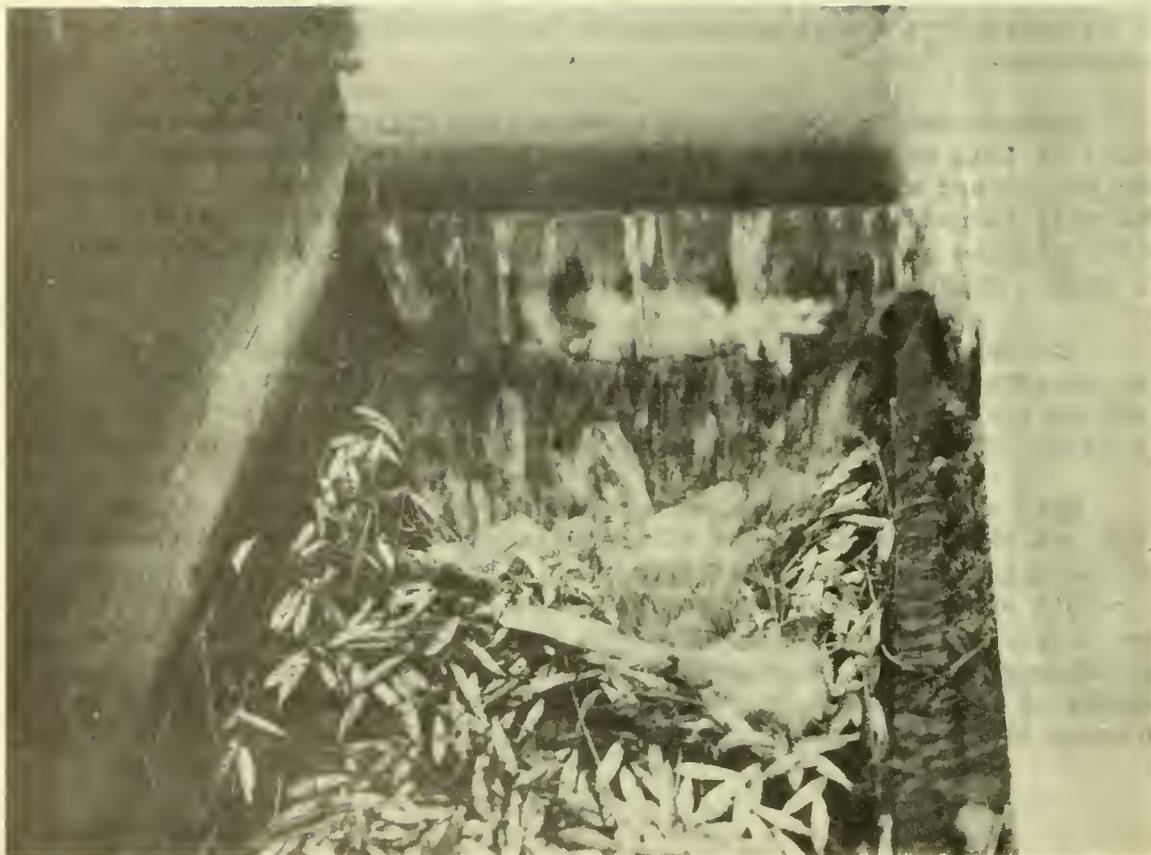
Figure 6.-- Dead chinook fingerlings in a Wenatchee River unscreened irrigation diversion ditch on July 14, 1940. Over 1,800 dead fingerlings were found in this ditch on the above date. A properly constructed and operated screen would have prevented this loss.
