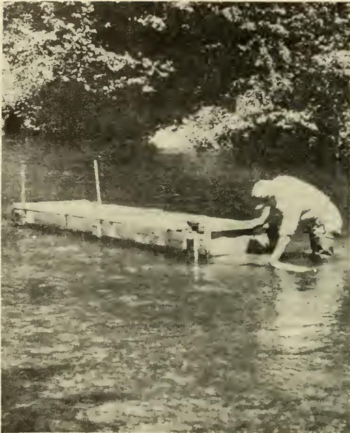
Figure 49.--Raceway used in Ocqueoc River to determine length of hatching period and production of larvae from the redds. Left hand of attendant is on funnel from which plankton net extends downstream.
