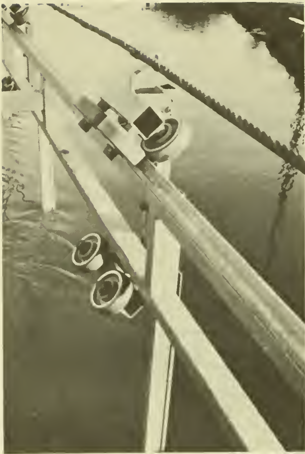
Figure 8.--Connector between haul-line and carriage.
