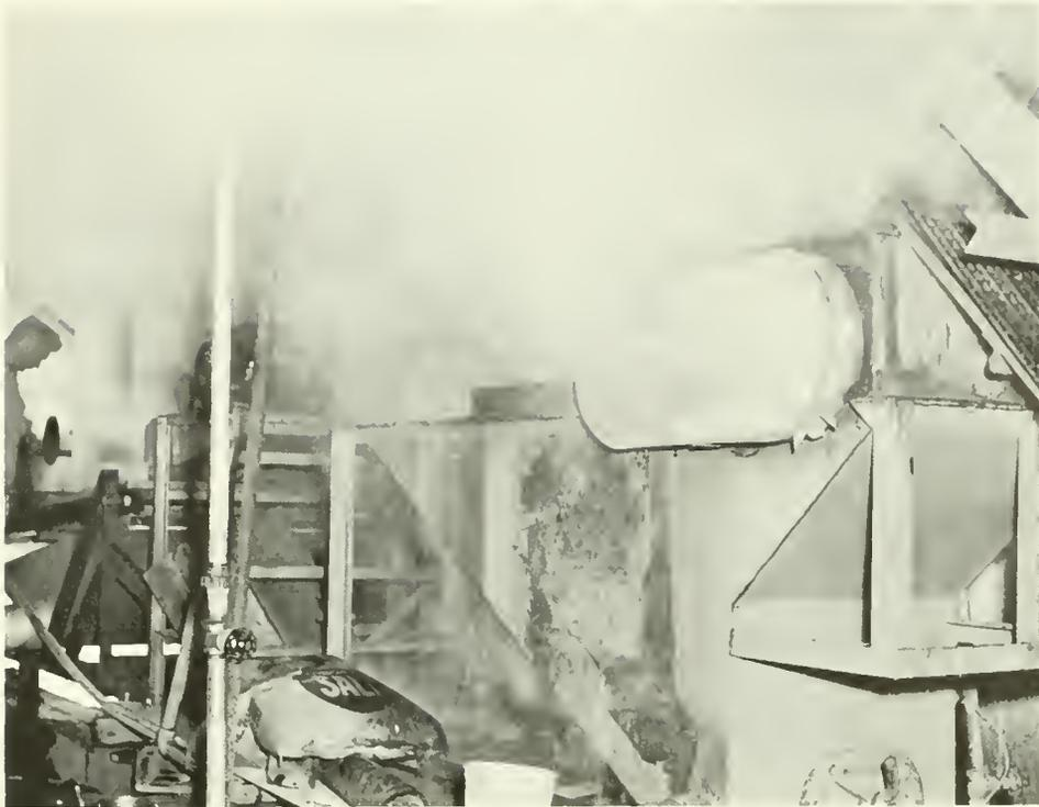
Figure 2.—The shell stock hot water, heat shocking tank with the conveyor for transferring the shell stock to the second set of rotating metal rollers.
