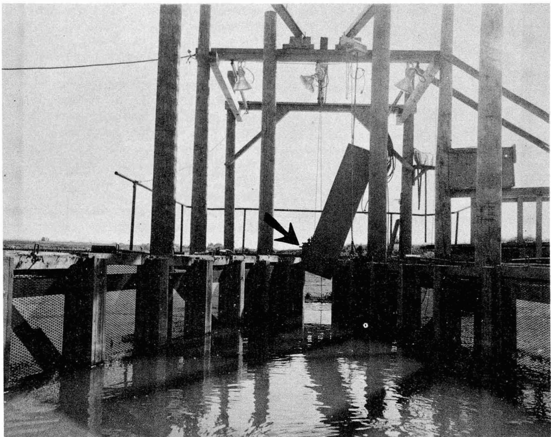
FIGURE 10.—Lead-in screens and throat (arrow) of array trap.
