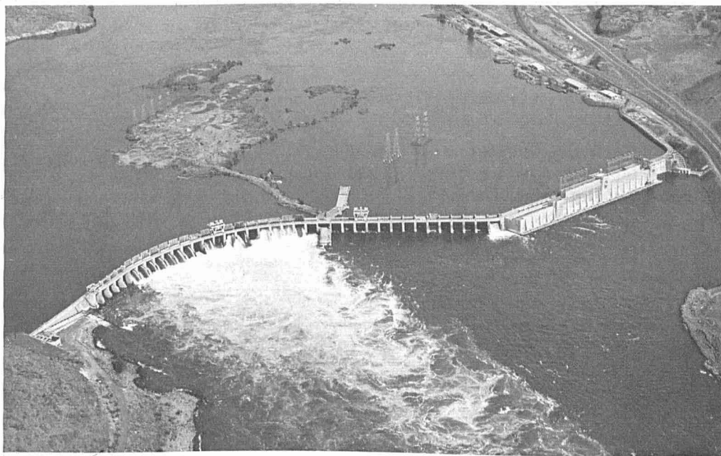
FIGURE 4.—Rock Island Dam after Wanapum Dam had been built. Note how the rocks and the lower portion of the right-bank fish ladder, visible below the dam in Figure 3, have been inundated in Figure 4.
