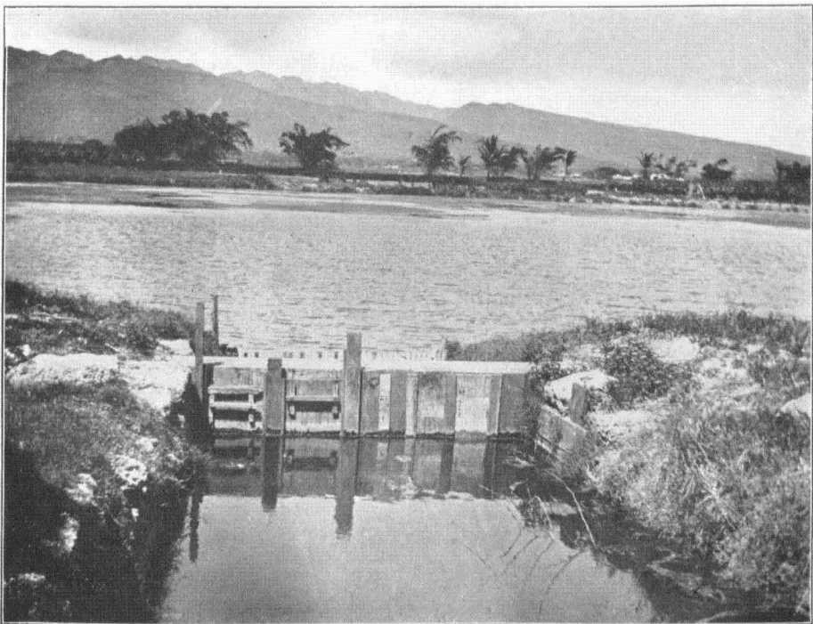
SLUICWAY LEADING INTO INTERIOR FISH POND, WAIKIKI, OAHU.
