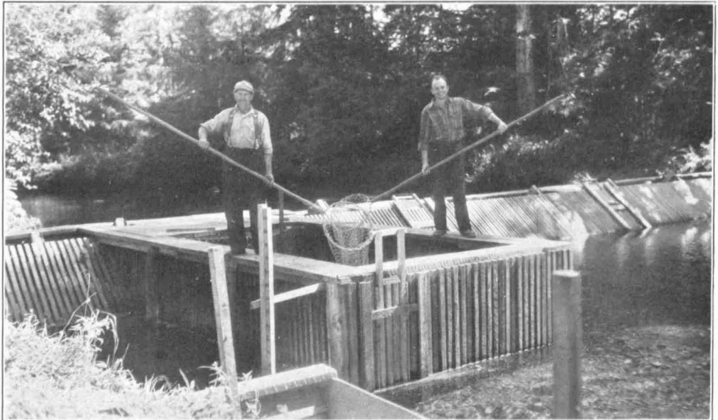
FIGURE 7.—Fish trap built in weir at Snake Creek. The large dip nets held by the operators were used to lift the salmon out of the trap. The sliding gate in the weir just to the right of the trap was opened when the salmon were counted through the weir.
