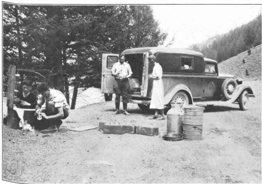
FIGURE 5.—One of the field-laboratory trucks, showing stream-side operations. These trucks were equipped with apparatus and chemicals, sampling and collecting outfits, dredges, and seines. Each truck unit was able, therefore, to make detailed investigations at any stream site which could be reached by car.
