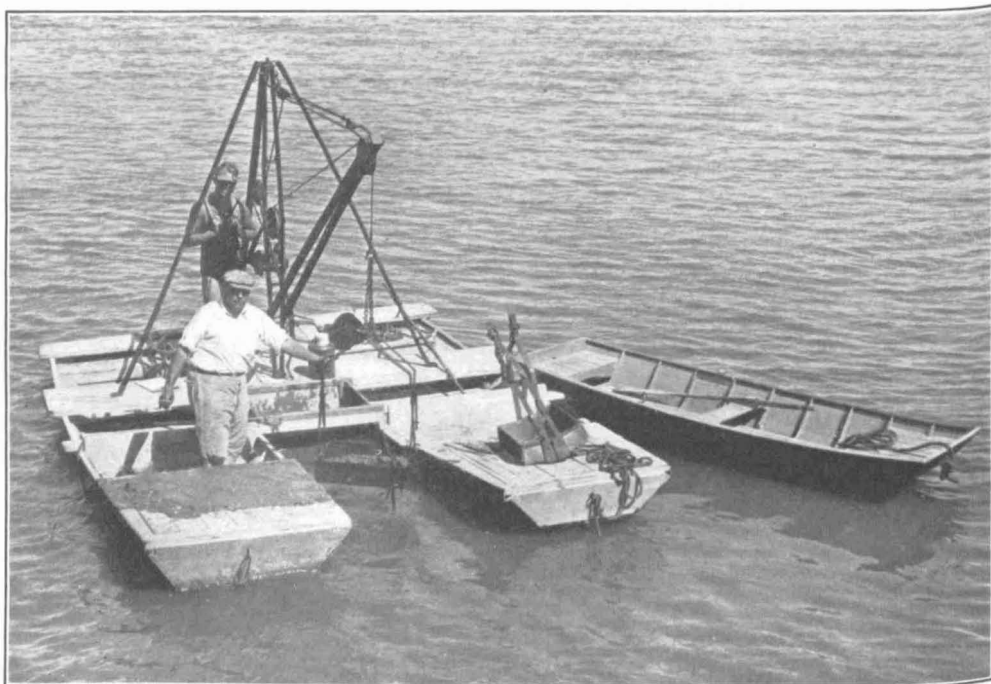
FIGURE 4.—Mussel dredge in operation from catamaran. This dredge was used in the study of bottom conditions where rocks and other obstructions made use of Peterson dredge impossible.
