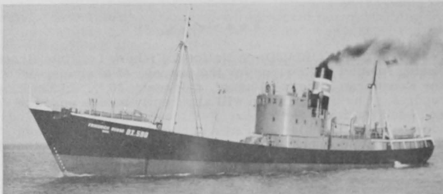
A 590-ton German steam trawler (capacity, 275 metric tons).
