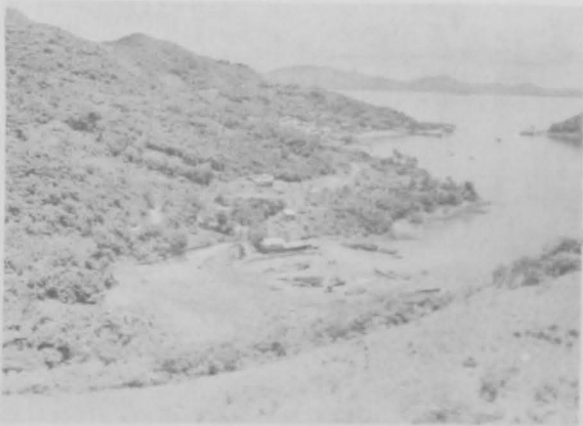
Fig. 9 - Taboga Island showing construction and dirt movement in the foreground. (Photo taken the latter part of 1955.)
