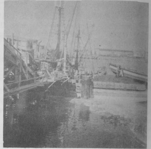
FIG. 1 - SUCTION PUMP HOOK-UP UNLOADING SARDINES FROM VESSEL TO CONVEYOR BELT AT PORT HUENEME.
