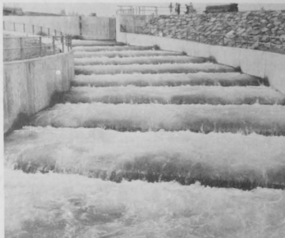
Fish ladder at Bonneville Dam, Columbia River.
