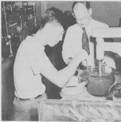
Fig. 1 - Experimental ore flotation employing fish-oil fatty acids is being carried out at School of Mines and Metallurgy, University of Minnesota.
