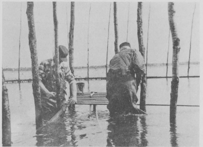
Fig. 8 - Building the ramp for the bottom of the gate.
