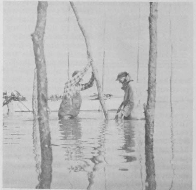
Fig. 3 - Setting one of the heart poles. Water temperature during this early spring operation averages 35-39 degrees F. Summer temperatures will go up into the 70's.
