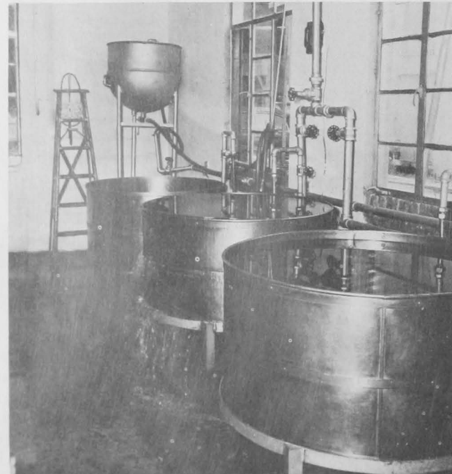
Fig. 21 - Oysters are bailed from the low-mounted blower tanks in this installation. Tanks may hold 20 to 40 gallons of oysters.
