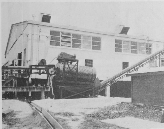
Fig. 39 - Canning oysters is an important industry in the South. Canneries start operations in the Spring when the yield per bushel of oysters is at its seasonal high. The shellstock is washed to keep mud and debris from the cookers.
