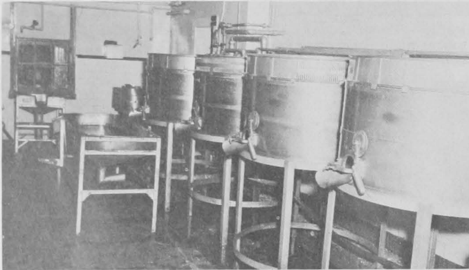
Fig. 19 - Chesapeake Bay plants use blowers to clean the shucked oysters. In this plant, blowers are mounted high enough so that they discharge through the open gate-valve directly onto the packing skimmer. Note the slotted collar to retain oysters during the overflow rinse period.
