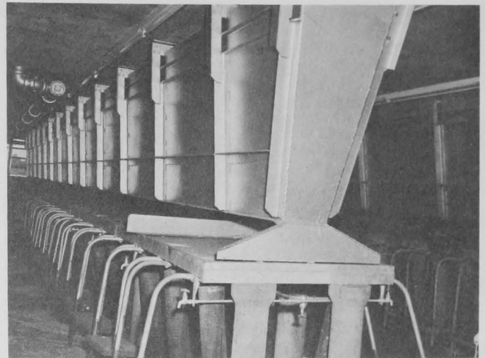
Fig. 12 - These shucking benches have overhead bins. Large rubber pipes under the bench carry empty shell to a basement conveyor system.
