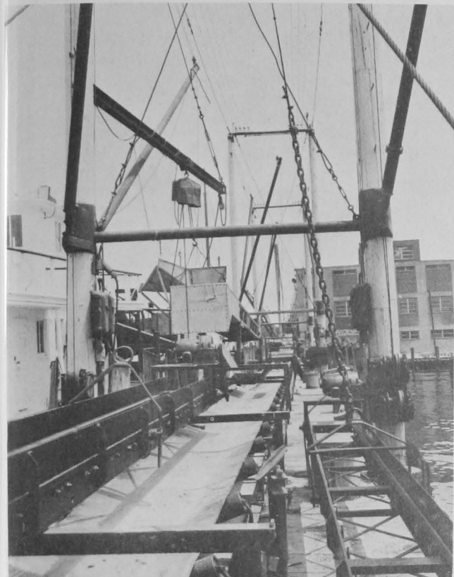
Fig. 3 - This plant has a dock conveyor system by means of which eight large dredge boats can be unloaded at one time.
