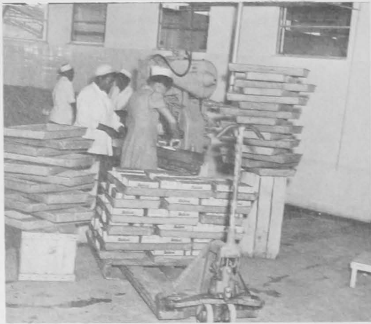
Fig. 31 - Space is left between units to permit circulation of the freezing air blast.
