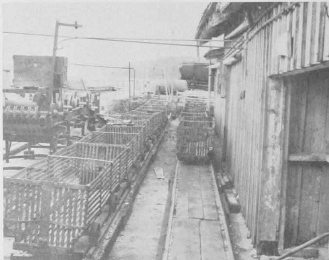
Fig. 43 - Metal-slot cars hold the shellstock during steaming. On the left is a specially designed shellstock washer with mesh belt removed.
