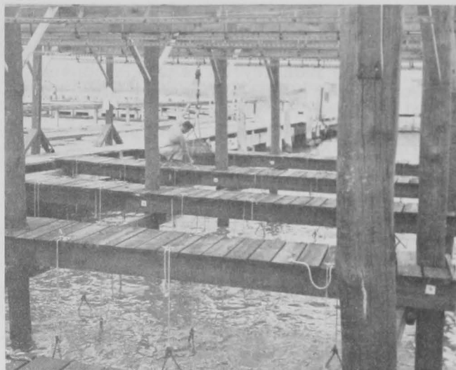
Fig. 1 - Overall view of tray rack showing construction of walks and position of superstructure.
