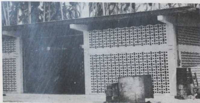
Fig. 3 - Prior to shipment, bagged fish meal is stored in this ventilated building of Puerto Caimito fish meal plant.
