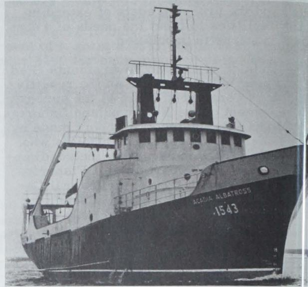
Fig. 1 - The Acadia Albatross, one of Canada's newest and most modern stern trawlers, is an all-welded steel vessel strengthened for navigation in ice. Main specifications are: length overall 152 feet, breadth molded 33 feet, and gross tonnage about 6,000 tons. The vessel was launched in Lauzon, Quebec, November 23, 1964, for a Nova Scotia fisheries firm.
