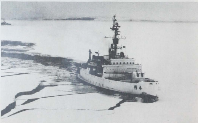
Fig. 9 - The 310-foot, 8,449-ton, 21,000-horsepower U. S. Coast Guard "Glacier," America's largest icebreaker, opens a channel in the Antarctic's McMurdo Sound. The vessel now is engaged in a 2- year international oceanographic study of the Weddell Sea.
