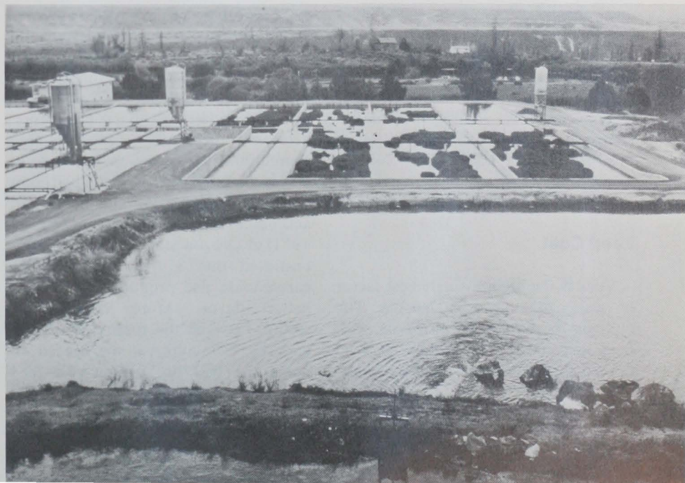
Figure 5.—Large-scale trout production ponds near Buhl, Idaho. The tall metal silos are for dry feed storage and supply the feed lines to the automatic feed dispensers in each raceway.
