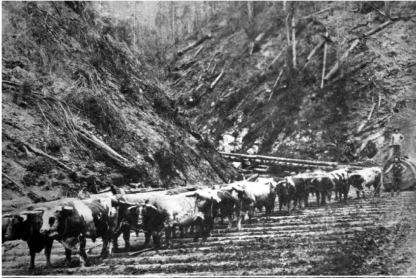
Figure 7.—Oxen hauling logs on a “corduroy road” in Mendocino County, ca. 1851. Photo courtesy of the Held-Poage Memorial Home and Mendocino Historical Society, Ukiah, California, from the Robert Lee Collection.
