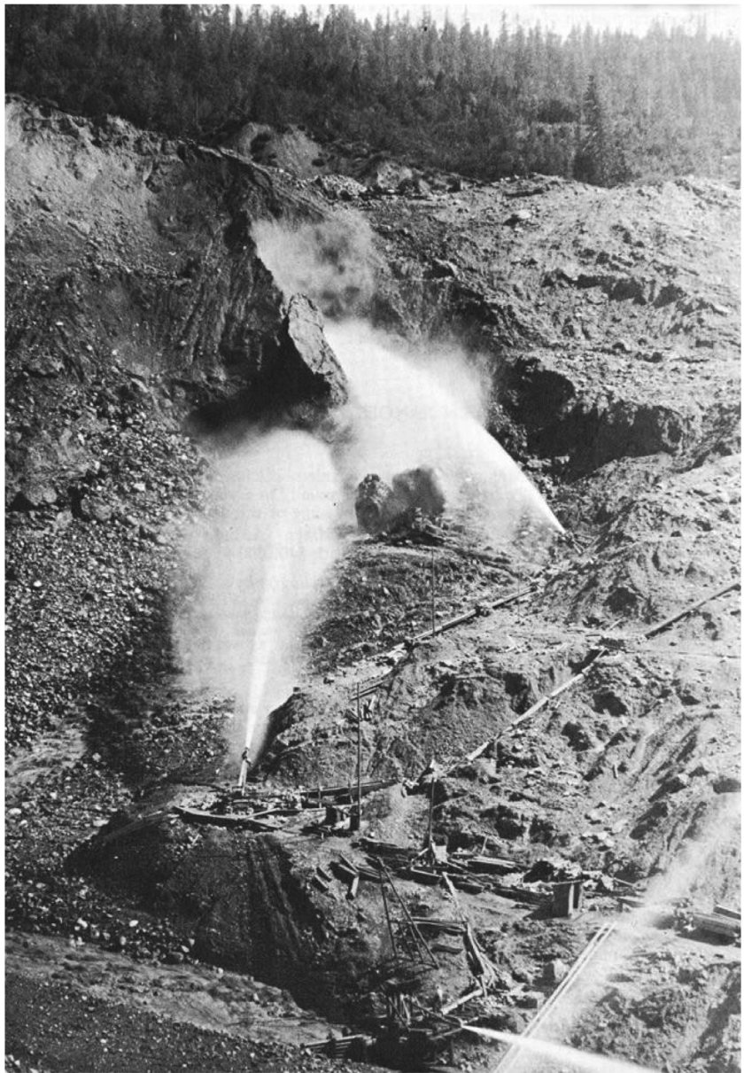
Figure 10.—Hydraulic mining at the La Grange Mine (1851–1918) near Junction City in the Trinity River basin. Photo taken ca. 1914. From Clark 1970.
