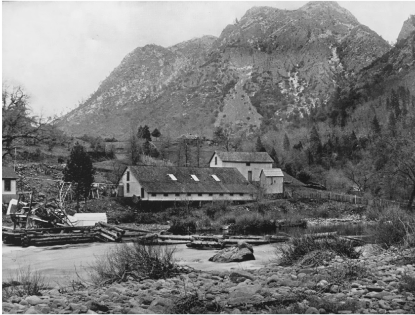
Figure 5.—Baird Hatchery along the McCloud River taken between 1890 and 1897. Figure from Stone (1897).
